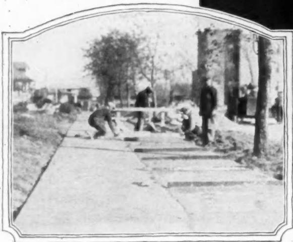
Sidewalk, Floosmoor, Ill. High-Early-Strength *Universal* concrete obtained by J. D. Smith, contractor, using standard *Universal* (not special) cement, the same quality *Universal* regularly handled and furnished by Darr Coal & Supply Co., Hazel Crest, Ill.
