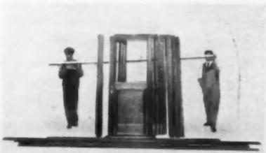
Here is the partition shown at top of page, taken apart and ready to be re-erected in new location. Note how compactly it piles for storage or shipment.
