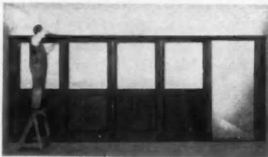
Lower crown moulding is also screwed in place. Remove it and the coupling irons and sections are ready to be moved.
