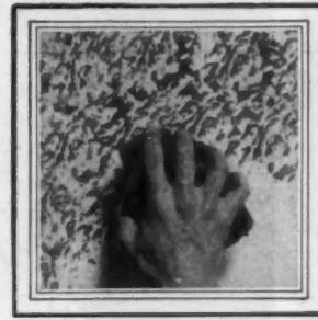
3. Then the flat side of the sponge is tamped against the wall, leaving an individual design where the high parts of the sponge come in contact with the surface.
