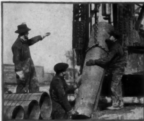
—that's one section of a spirally reinforced steel shell for a Raymond Concrete Pile—every Raymond Concrete Pile is poured into a spirally reinforced tapered steel shell and the shell is left in the ground.
