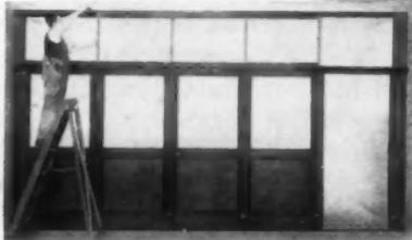
Removing crown moulding with screwdriver. Extension posts then slip down out of sight into main posts.
