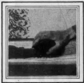
2. After a light undercoat is applied and allowed to dry, a little of the darker finish is poured on a board or other flat surface, into which the flat side of the sponge is pressed.
