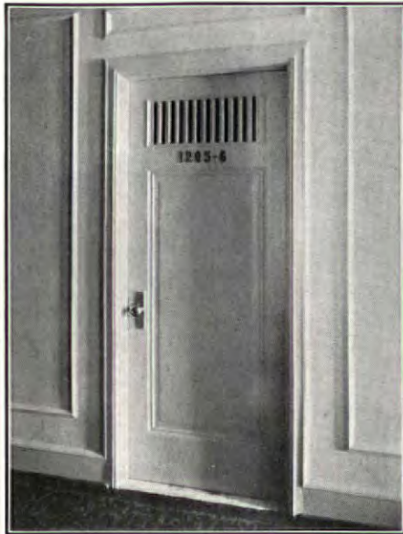
Typical door in a modern hotel equipped with VENTADOOR, a ventilating panel that excludes light and vision. SEND FOR BOOKLET CATALOGUE IN SWEET'S
