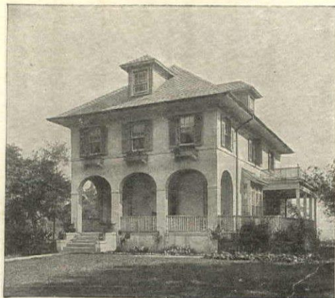
A stucco finish on a Natco Hollow Tile wall becomes a part of the wall itself
