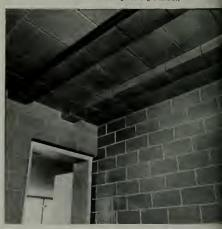
(above) Office Storage Vault at Friden Calculating Machine Comp 8" Kraftile Housing blocks faced with 4" Kraftile Glazed Wall I provide 12" fire-and-waterproof walls, Ceiling is pre-cast Kr beams and 4" thick Kraftile slabs, Will carry 75 lbs. per sq. f
