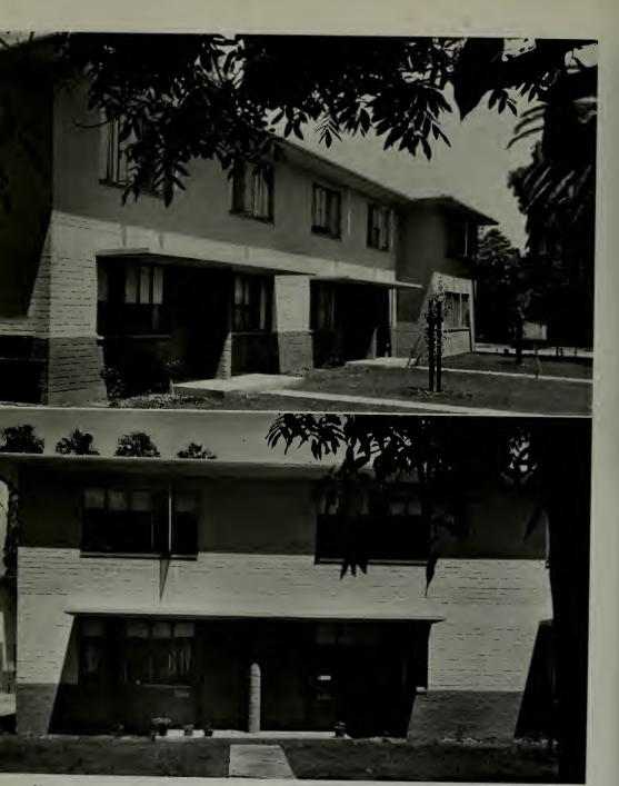
Close up of a twin apartment unit showing wide overhang flat roof and hooded entrances, the latter formed by a cantilevered extension of the second floor slab
