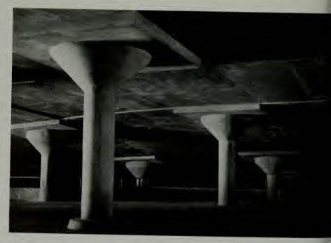
Irregular shaped columns, some 50 in number, serve as floor supports, formed in metal and installed by the Steel Form Contracting Company
