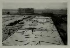
SISAL paper used to cure and protect concrete floor at United Airlines Terminal
