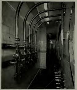
Government Collor contains four 100-barrel and eleven 250-barrel glass lined tanks. The Wall Units are Kraftile Ceramic Glazed. Cellular, they are ideal for a refrigerated room like this. Kraftile Vitreous 8 x 8 Quarry Tile is used to finish the floor here, in the Meter Room, and the entire working area of Machinery Hall. 13,300 square feet were used—the largest quarry tile installation in San Francisco last year
