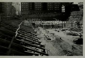
Detail of paired timber braces for steel piles. The 24-foot variation in street levels (between corners at upper right and lower left! determined lengths and angles of braces
