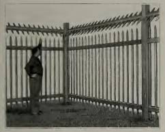
the WPB. The fencing, which is of sturdy construction, weighs 20.4 pounds per lineal foot, 2,000 lineal feet or 44,000 pounds to a car. This innovation in plant protection has been approved by the Chief Engineers and the Provost Marshal of the Army Engineering Corps.
