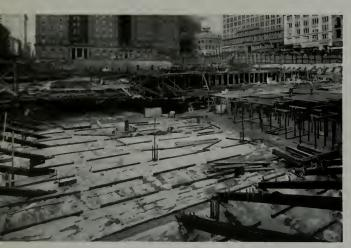
Most reinforcing bars were spread around the timber braces; a few pierced them. Adjacent slabs had extra reinforcement. Fiberboard sheathed the timbers during pouring. 300,000 sq. ft. of sisal fibre reinforced paper used to cure and protect the concrete
