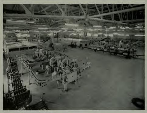
MACHINERY HALL, THE FIFTH FLOOR OF THE NEW BOTTLING PLANT, WHERE ALL BOTTLING, LABELING AND PACKAGING OPERATIONS ARE CONCENTRATED
