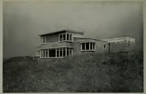
OCEAN SIDE, WILCOX COTTAGE Sandblasted and gray-stained siding with appearance very similar to buildings tempered by sea fronting structures 10 years old; 85 # white granulated surface rolled roofing;  $16 \cdot oz$ , copper flashing and galvanized nails throughout
