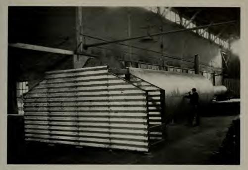
This Armco iron air-raid shelter is 50 ff. long and  $7\frac{1}{2}$  ft. high and will accommodate 50 persons. Four unskilled workmen can erect the shelter with simple tools in a few hours.
