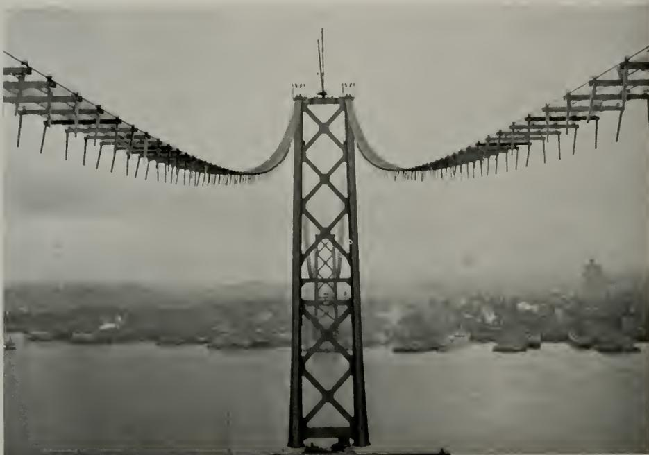
CAT WALKS, EACH TEN FEET WIDE, WITH WIRE MESH FLOOR FOR WORKMEN TO TRAVEL OVER WHILE HUGE CABLES ARE BEING STRUNG
