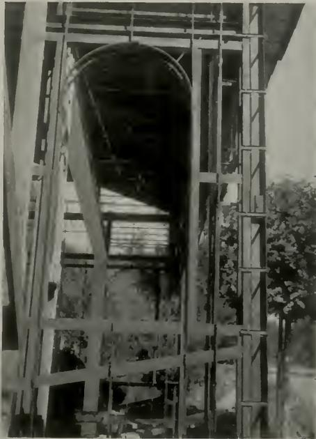
STEEL FRAME HOUSE—Exterior view at south end of garage showing method of using  $\frac{3}{4}$ " furring channels around corners and method of using  $\frac{3}{4}$ " furring channels for arched window openings.
