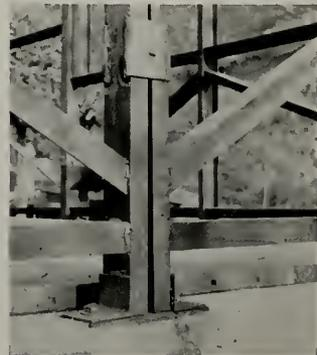
STEEL FRAME HOUSE—Steel anchor bolts are imbedded in concrete foundation to secure column members of the steel wall framing units.
