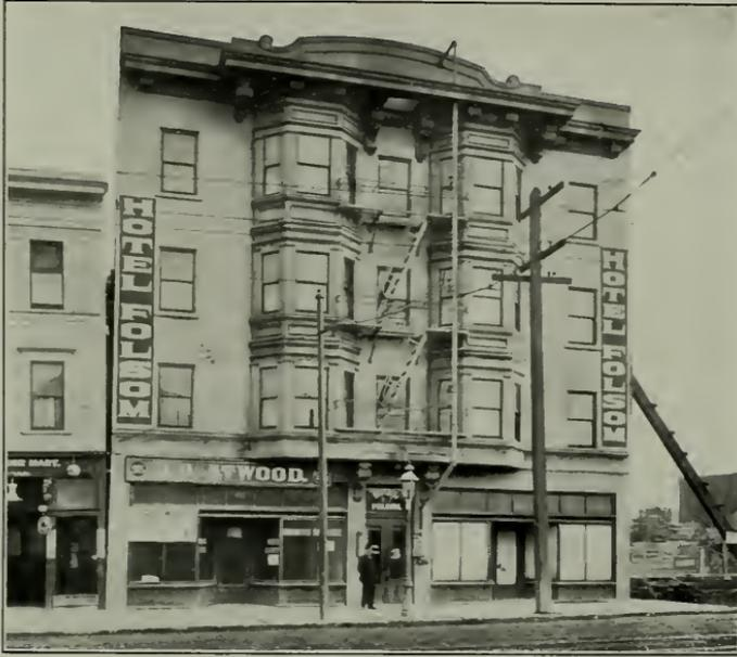
*The Walls of This Concrete Building Lean Over More Than Two Feet at the Top*
