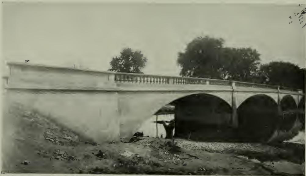
*Three-Span Concrete Bridge at Plainfield
