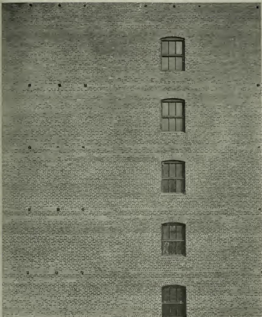
*Reinforced Brick Wall on Steel Frame Eight-Story Building. Wall Eight and One-Half Inches Thick.
