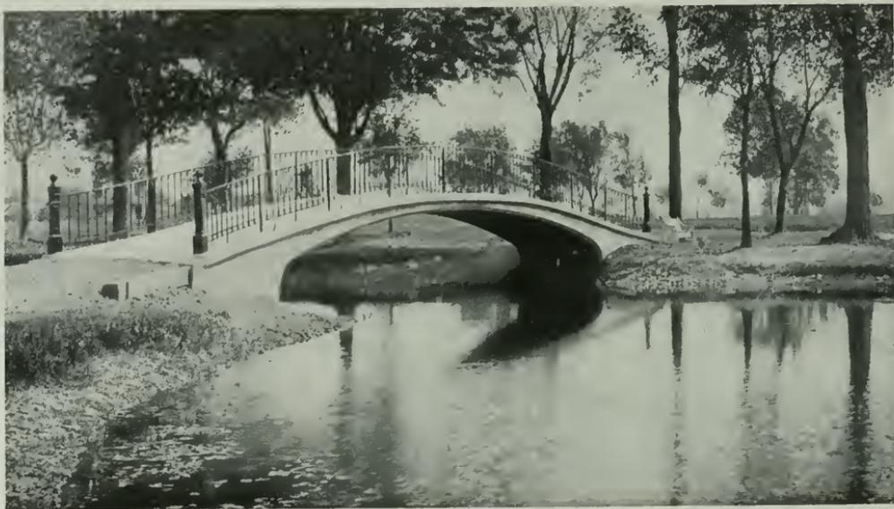
*An Attractive Reinforced Concrete Bridge with 40 foot Span and Ornamental Iron Railing
