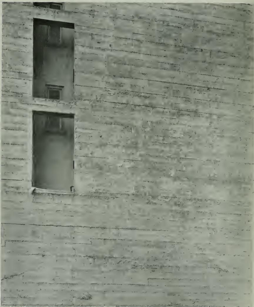
*Reinforced Concrete Wall on Steel Frame Nine-Story Building. Wall Six Inches Thick.
