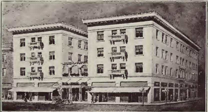
*Montgomery Hotel, San Jose. An All-concrete Structure, Reinforced with Deformed Steel Bars. This Building Is Nearing Completion and Will Cost Close to \$200,000
