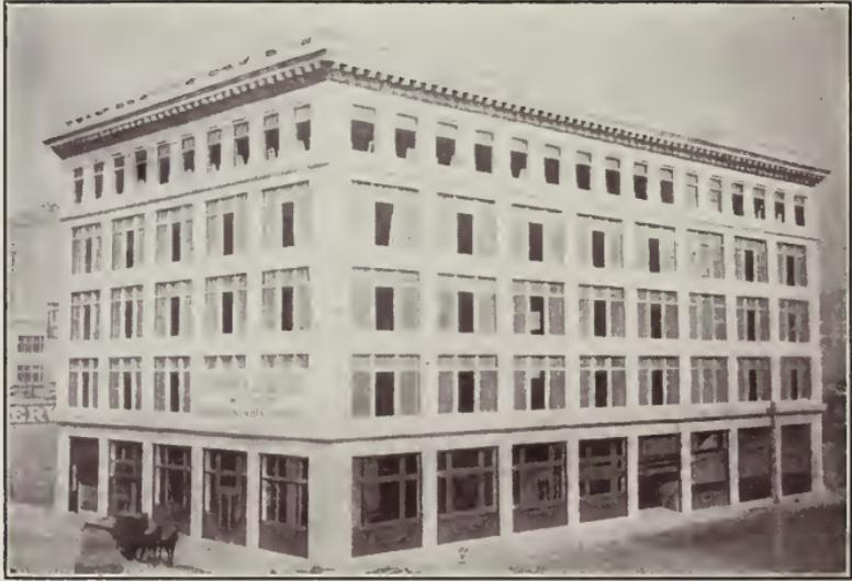
*Tillmann & Bendel Building, San Francisco. One of the First Concrete Buildings for Wholesale Purposes Completed after the Fire. The Kahn System of Reinforcement Is Used
