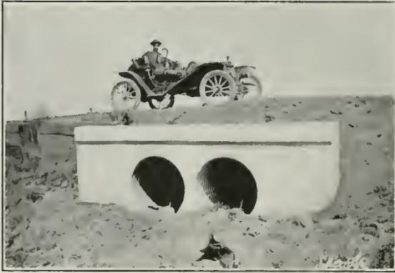
*A Wooden Bridge Has Been Replaced by Two American Ingot Iron Corrugated Culverts and Work Done by the San Joaquin County Highway Commission, Mr. R. M. Morton, Engineer, Under Bond Issue by that County of \$1,800,000*
