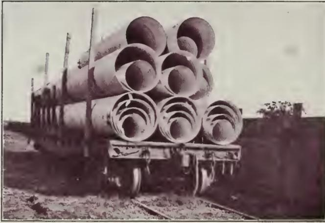
*Carload of American Ingot Iron Culverts. Ranging from 12 to 36 Inches in Diameter.*
