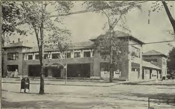
Ferroinclave was used for Roof of this Garage
