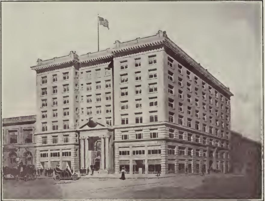
*Y. M. C. A. Building, San Francisco, Steel Frame and Reinforced Concrete Walls
