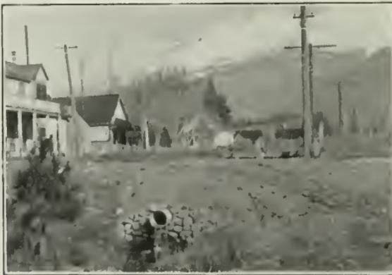
*An Ingot Iron Corrugated Culvert Under the Main Street of the Town of Susan. Note the High Snow Capped Peak of Mt. Shasta in the Back Ground*
