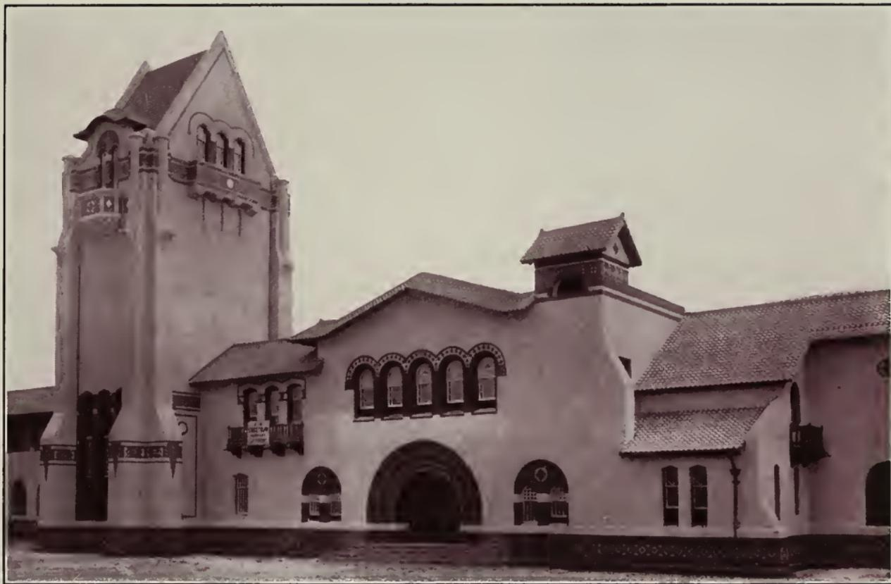
*Tower and Main Entrance, San Jose State Normal School. This Building Is Roofed with Red Clay Tile. The Exterior Treatment of Concrete Walls Is Pebble Dash and Faience Tile*
