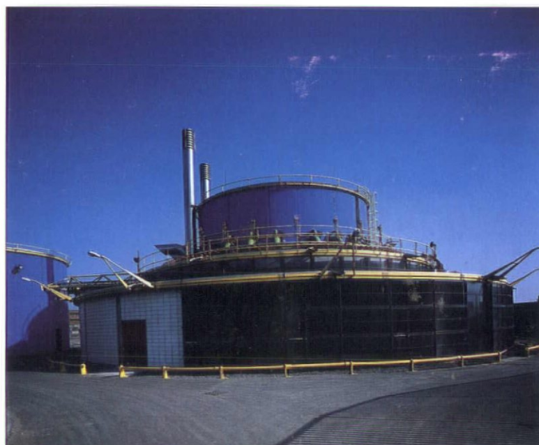
Richard Rogers, Pumping Station, Royal Victoria Dock, London
