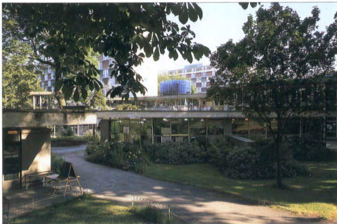
Single storey Infant School in the foreground, double storey administration department with staff room patio in the background Photographs (colour): Mario Bettella
