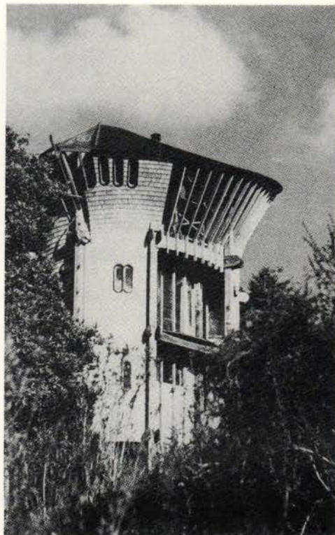
11 House at Stinson Beach, California, 1969, Valentino Agnoli. While the guidebook describes this house by a former Goff student as one of several 'handcrafted, technological fantasies', the structural discipline is readily visible as part of the exterior expression of columns and beam ends. The handcrafted label applies equally appropriately to almost any free-standing house anywhere. The verbal fantasies stimulated by Goff's architecture are also part of the professional response to the more original buildings by his apprentices. (Photo: 'A Guide to Architecture in San Francisco and Northern California', by Gebhard, et al)
