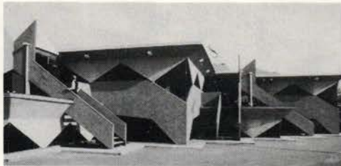
20-23 Shalako South Office Building, Albuquerque, 1973-4, Bart Prince. The cheapest type of construction, wood truss and frame, covered with stucco and the tightest planning restrictions produced a speculative rental property on a busy corner. The economy of a first floor down half a flight makes maximum use of required foundation walls and allows equalised rents for both floor levels. Air-conditioning units eliminate the need of openable windows. Fixed smoked glass contrasts with the stuccoed, structural triangles.
