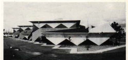
20-23 Shalako South Office Building, Albuquerque, 1973-4, Bart Prince. The cheapest type of construction, wood truss and frame, covered with stucco and the tightest planning restrictions produced a speculative rental property on a busy corner. The economy of a first floor down half a flight makes maximum use of required foundation walls and allows equalised rents for both floor levels. Air-conditioning units eliminate the need of openable windows. Fixed smoked glass contrasts with the stuccoed, structural triangles.
