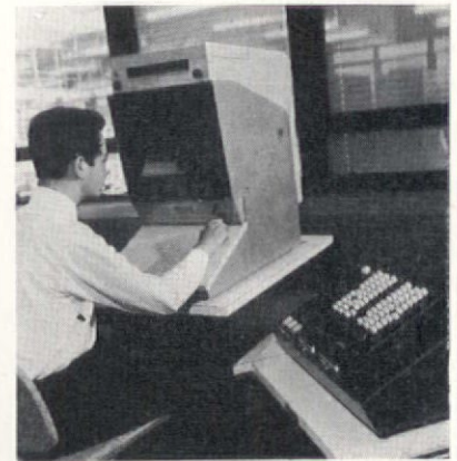
3 Miracode retrieval system for reproducing details of microfilmed statements
