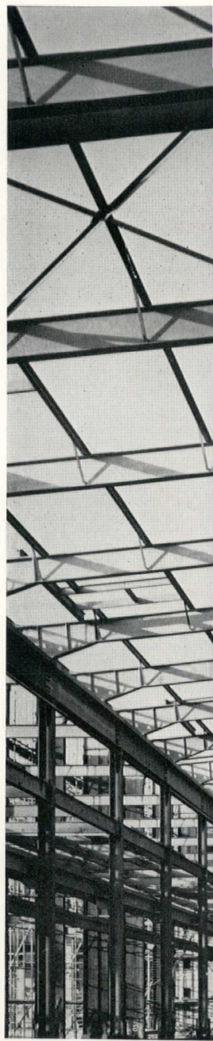
Thames Board Mills. Typical welded rigid frame
