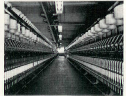
Ardsley Mill, near Wakefield, 1912; interior and exterior of this early in situ reinforced concrete mill, still retaining the form of the early nineteenth-century mills Photo: Harrisons Studio, Bradford
