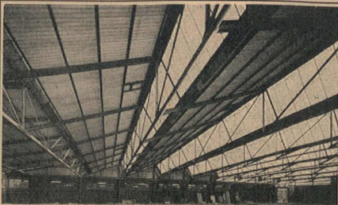
North light construction gives clear roof area 120' wide × 300' long.
