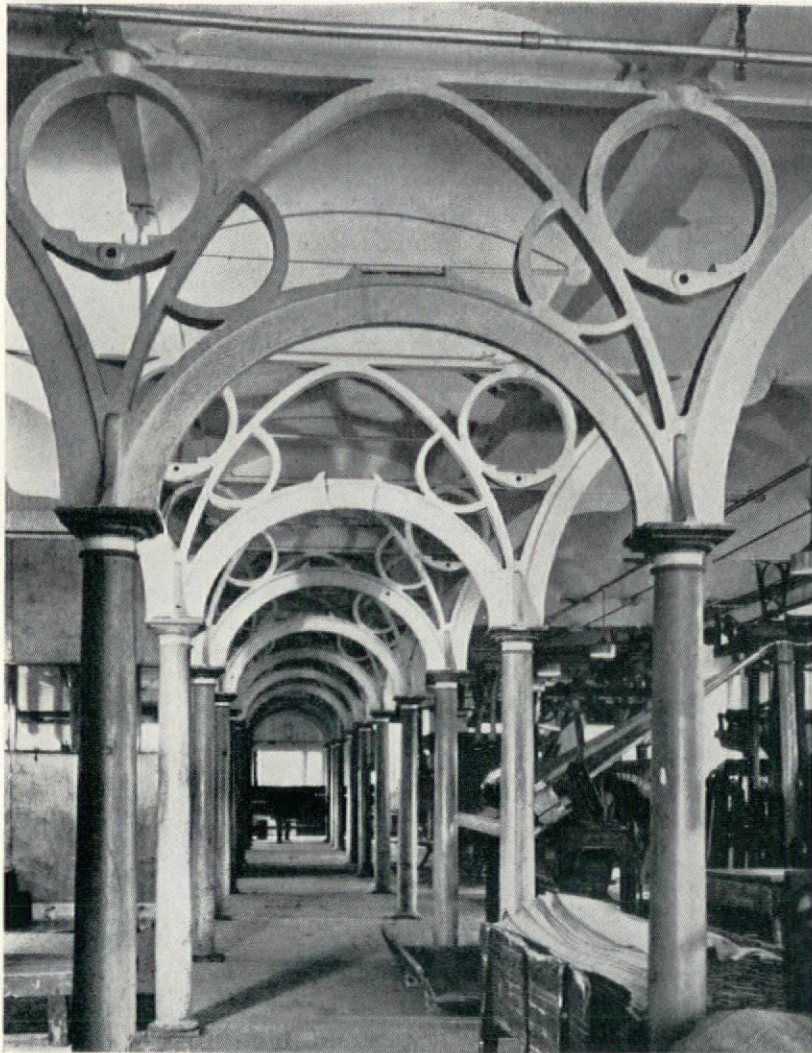
◁ Interior of Stanley Mill showing the unusual cast iron structure. This mill combined with its functional elevations some refined Georgian style detailing Photo: The Functional Tradition
