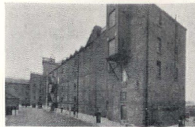
Exterior view from south. During conversion in 1897, most of the windows were blocked up. Steam engines in the end blocks were linked by shafts and gearing to the machines on each floor Photo: Architectural Review April 1950
