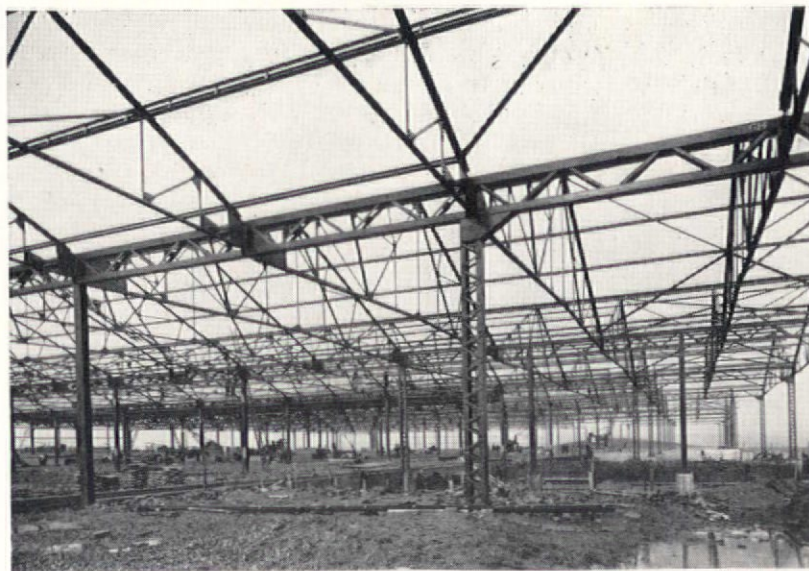
Edison Swan Electric Co. Typical multi-bay factory. Pitched roof with 'N' girder truss
