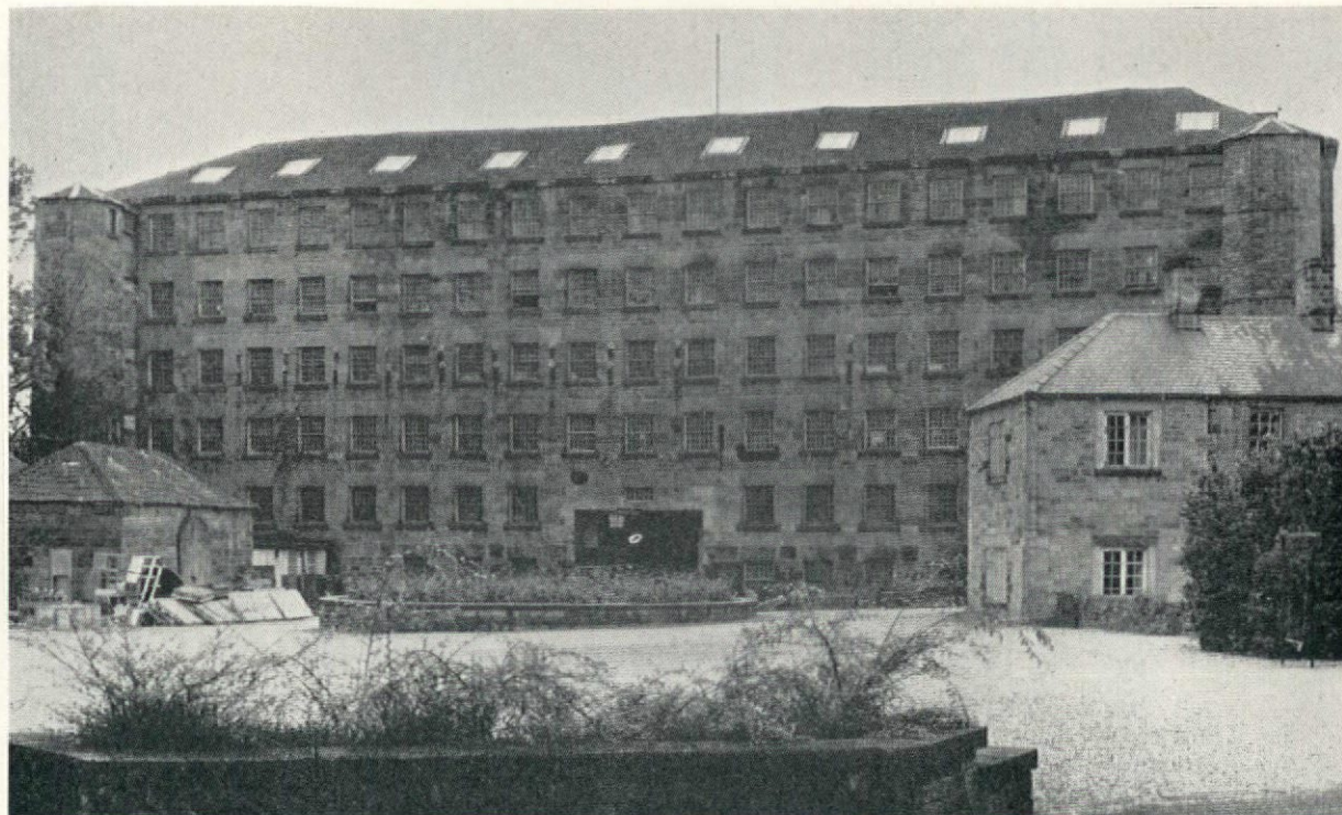
Calver Mill, Middleton, Derbyshire. 1785. One of the great early cotton mills of 6 storeys with 3ft thick walls at the base and an internal structure of cast iron columns supporting wooden beams now replaced by steel Photo: The Functional Tradition J. M. Richards, 1958
