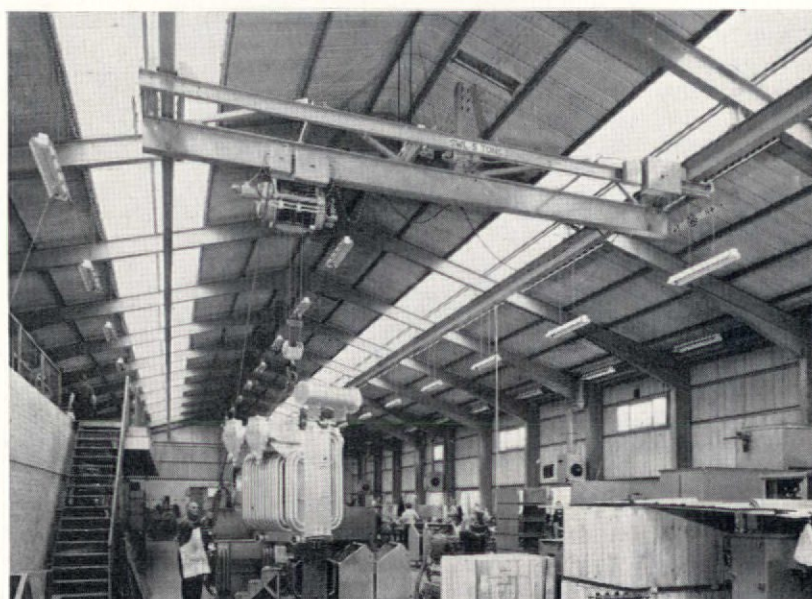
Condor Frame. Standard welded portal frame with small floor-controlled slung crane suspended from roof Photo: A'Court
