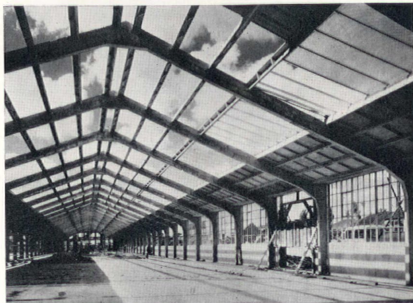
Pre-cast concrete portal. Apart from the ability to make simple fixings to the frame, the disadvantages and advantages of either material are marginal Photo: C & CA
