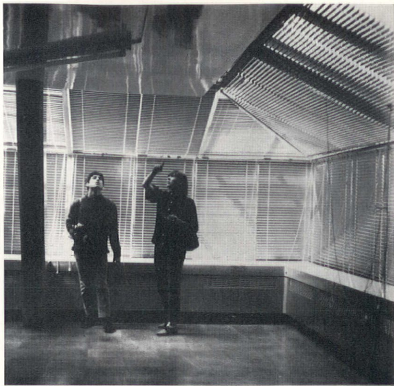
The venetian blinds are used on the underside of the step-out glazing. Ceilings are painted white gloss and raking columns and upstand beams (which are also horizontal ducts and window seats) are painted grey gloss
