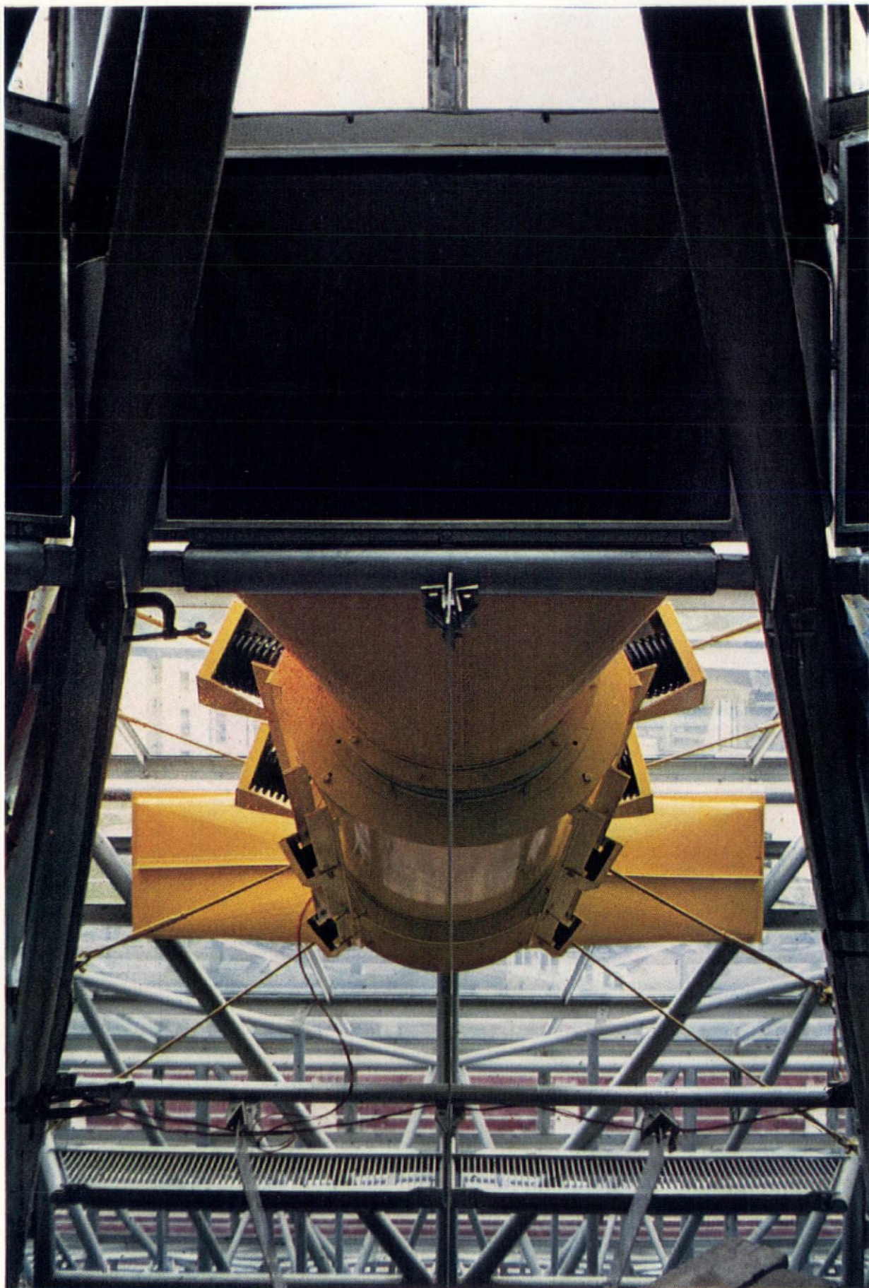
One of the extract machines hanging in the apex of the trusses which span over the Reading Room. The other machines are red and blue
