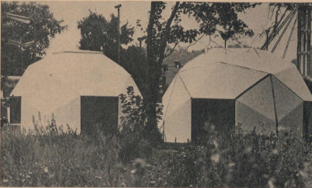
The Octagon House , made from corrugated paperboard, half an inch thick, in three layers, waterproofed and finished with a resin based coating which contains fine aggregate, giving the board a hard and flameproof surface. The panels come flat and ready surfaced. The edges are folded in and bolted to join the panels. No other framework is used. The floor area is 422 square feet; basic price about £300. The pavilions can be joined together, a function of the close packing geometry which underlies the design.
