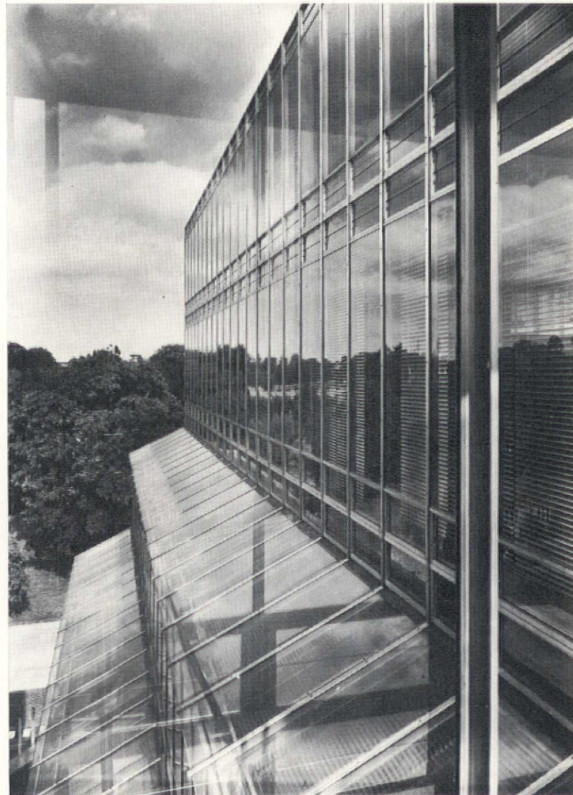
View of north elevation from the glazed link between the towers and the upper floors. Glass louvres at high and low level provide draught free ventilation as they are positioned behind the upstand beams
