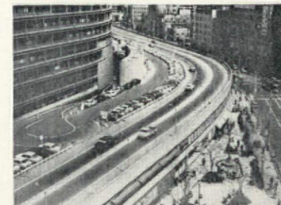
17, 18, 19. Central Station Bypass, Tokyo. Commercial uses have been relocated within the road structure, and the elevated roadbed creates better conditions for pedestrians at ground level while offering good views for motorists
