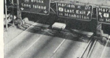
12. Opposing lanes of traffic stacked one above the other will achieve a narrower right-of-way. (a), (b) and (d) also permit local traffic and pedestrian access across the roadbed at ground level
