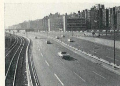
11. The motorway can with advantage be located alongside existing horizontal barriers which in themselves form edges to neighbourhood areas. The Turnpike in Boston, routed alongside railway tracks
