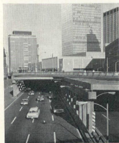
10. Continuous decking over the motorway is expensive and can produce unpleasant driving conditions for drivers. Freeway below the Prudential Centre, Boston
