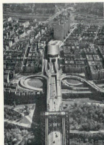
13. The Port of New York's development over the George Washington Bridge approach provides a unique example of buildings functionally related to the freeway being successfully incorporated within the motorway structure—namely the Bus Terminus Building and associated car parking facilities Port of New York Authority (Forum), March 1967
