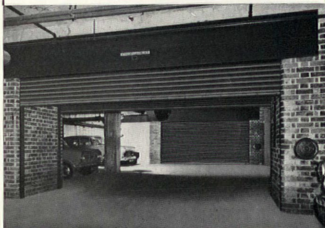
14 foot 'Protex' shutters installed in the car park basement of a new building at Whitechapel, London.
