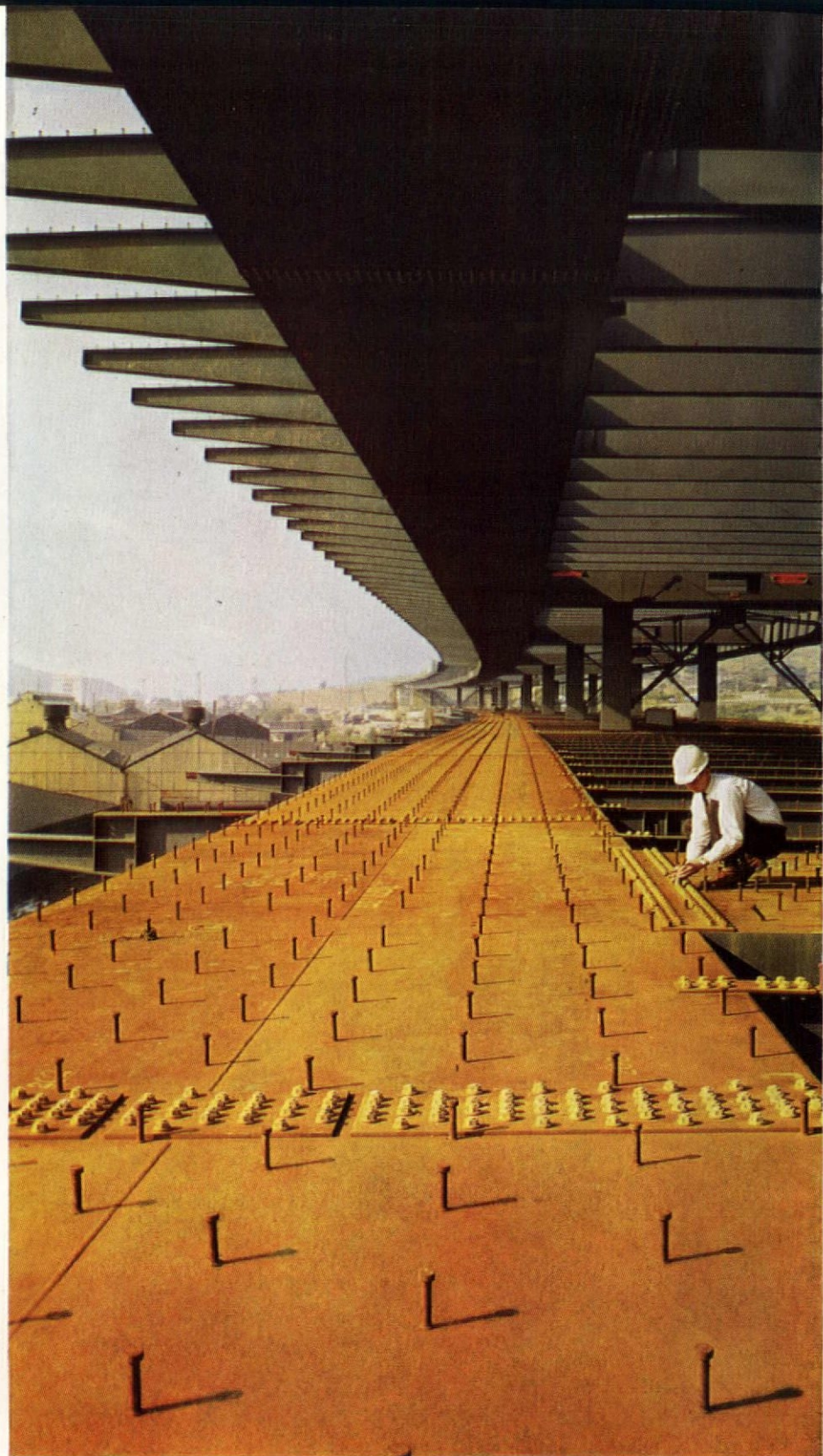
Spectacular two-tier Tinsley Viaduct. A major contribution to Britain's highway programme, this unique steel-girder structure spans a congested area in the Don Valley at Sheffield, and will carry M1 above and a local trunk road on its lower deck. Savings have been substantial due to final choice of a steelwork structure with large-
