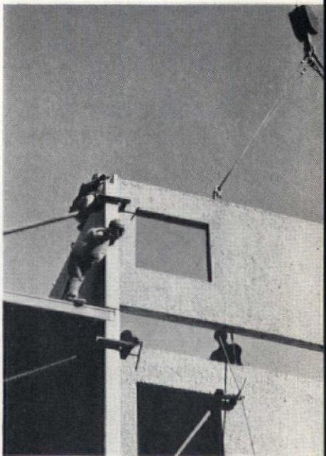
Walling units being guided over the 8ft long post-tensioning rods and placed in position.
