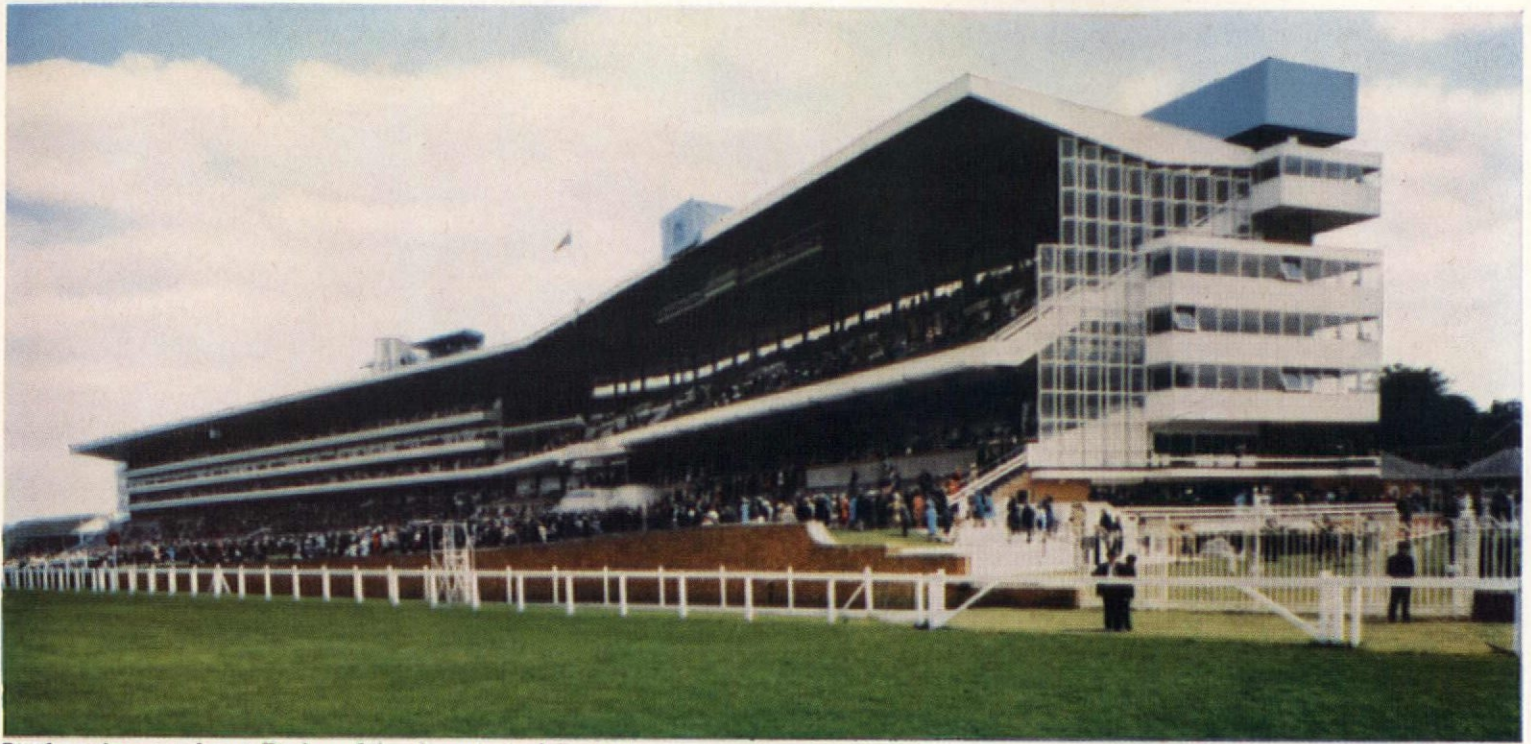
Steel—a winner at Ascot. Design of the elegant, steel-framed Queen Elizabeth II Grandstand takes advantage of advanced cantilever construction. New Royal Enclosure extension steelwork was completed in only 12 weeks. Structural steel by Boulton & Paul (Steel Construction) Ltd. Main Contractor: George Wimpey & Co. Ltd.
