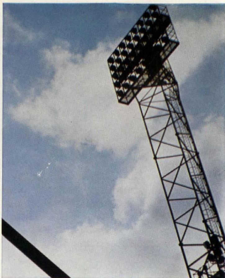
Higher lighting standards in strong, lightweight, cost-saving tubular steel. Flood-lighting towers are neat in appearance, offer less wind-resistance, cost less to paint and maintain. Hot-dip galvanizing resists corrosion. Designed by Ove Arup & Partners. Steelwork by Stewarts & Lloyds Ltd.
