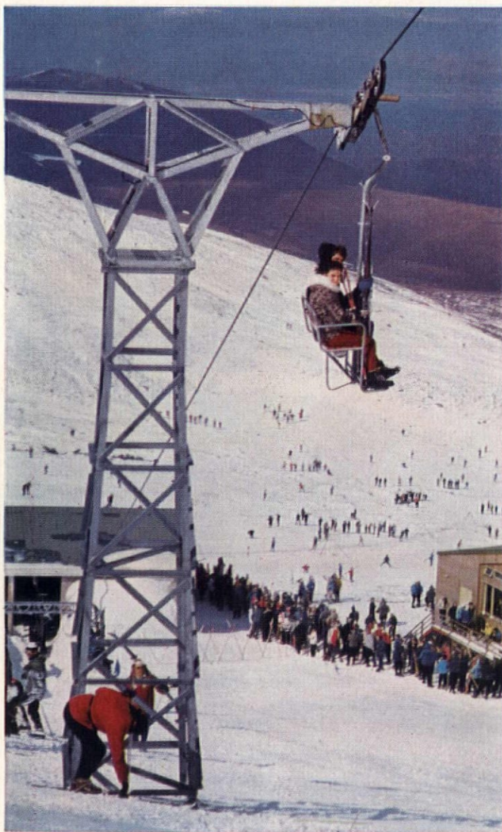
More accessible snowfields. Steelwork for the Cairngorm 'Chairlift', Aviemore, incorporates tubular and angle lattice construction—corrosion-protected by hot-dip galvanizing. Consulting Engineers: Blyth & Blyth. Steelwork by R. W. Hay Ltd, Edinburgh. Cables by British Ropes Ltd.
