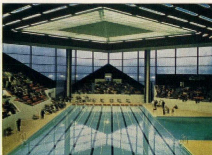
Structural steel for Leeds International Pool—with 3 pools, for tuition, competitive and recreational swimming, diving, water polo. 'Autofab' beams forming the 8 cruciform columns support steel lattice roof. Architects: J. G. L. Poulson in association with Leeds City Architect, E. Weston Stanley. Consulting Engineers: J. G. L. Poulson Associates.
