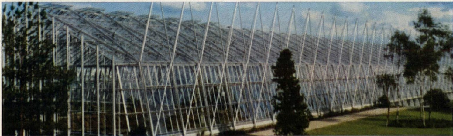
Suspension-type tubular steel Plant House, Royal Botanic Garden, Edinburgh. Visitors can view rare plants in natural settings. 'Inside-out' design will save maintenance caused by corrosive conditions within. High tensile steel portal framing is suspended from latticed tetrahedrons by \frac{1}{4} " dia. stainless steel wires. Designed in the Directorate General of Works, MoPBW. Steelwork by Finch Engineering Ltd.
