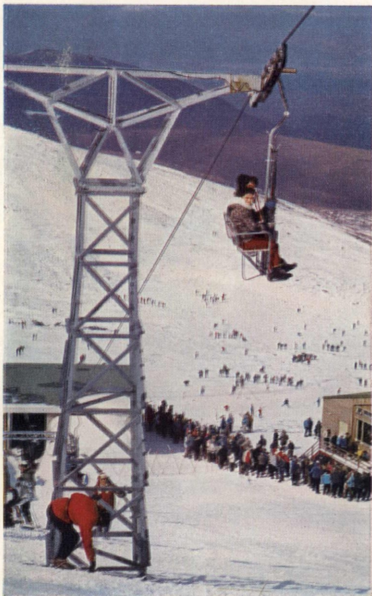
More accessible snowfields. Steelwork for the Cairngorm 'Chairlift', Aviemore, incorporates tubular and angle lattice construction—corrosion-protected by hot-dip galvanizing. Consulting Engineers: Blyth & Blyth. Steelwork by R. W. Hay Ltd, Edinburgh. Cables by British Ropes Ltd.
