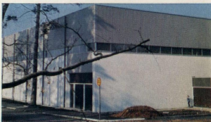
Multi-sport centres reduce costs with shared amenities. Steel-framed Sports Hall at Easthampstead RDC's Bracknell Sports Centre caters for many sport and leisure activities. Galvanized pvc-coated steel sheet vertical cladding by William Briggs & Sons Ltd. Architects: John Rice & Partners.
