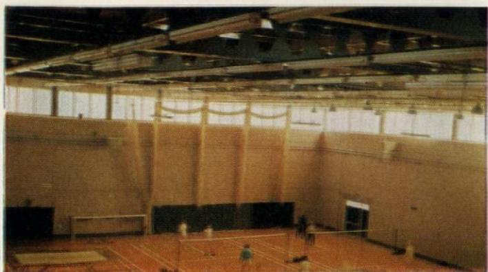
Harlow's 'Sportcentre' (above, and cover). Outstanding example of a purpose-designed community sports hall. Economical steel-frame structure employs weight-saving 'castellated' beams for wide, clear spans. Architects: Frederick Gibberd & Partners. Steelwork: Redpath Dorman Long Ltd.
