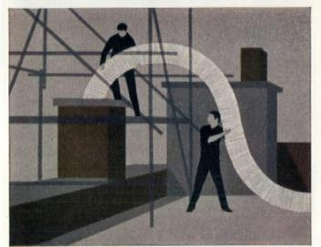
Highly flexible lightweight stabilised flue liners simplify re-lining existing chimneys to deal with corrosive products from oil, gas and solid fuel boilers. Sizes from 3 in. to 12 in. diameter. These rapidly installed flue liners, exclusively of stainless steel, resist heat and corrosion.
