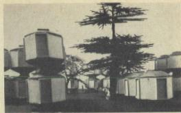
(the main shell of the structure is 1in plastic sandwich panel construction with an insulating core: the floor is single-skin with ribs beneath). The long sleeve of the concrete base fits into the floor/roof connector space, and is capped with single-skin g.r.p. to give a level floor.
