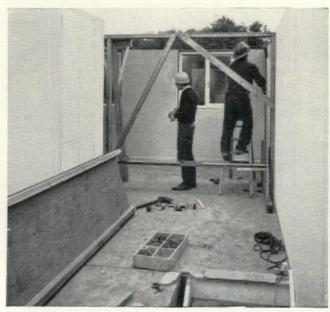
First floor interior with Plywood and C.L.S. T-beam floor.
