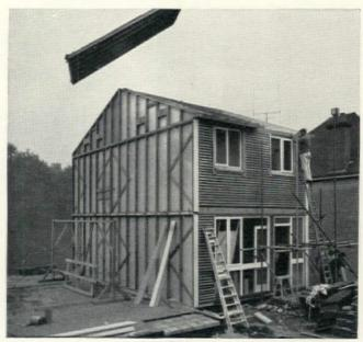
Party wall stud framing in C.L.S. with roof panel being lifted into position.
