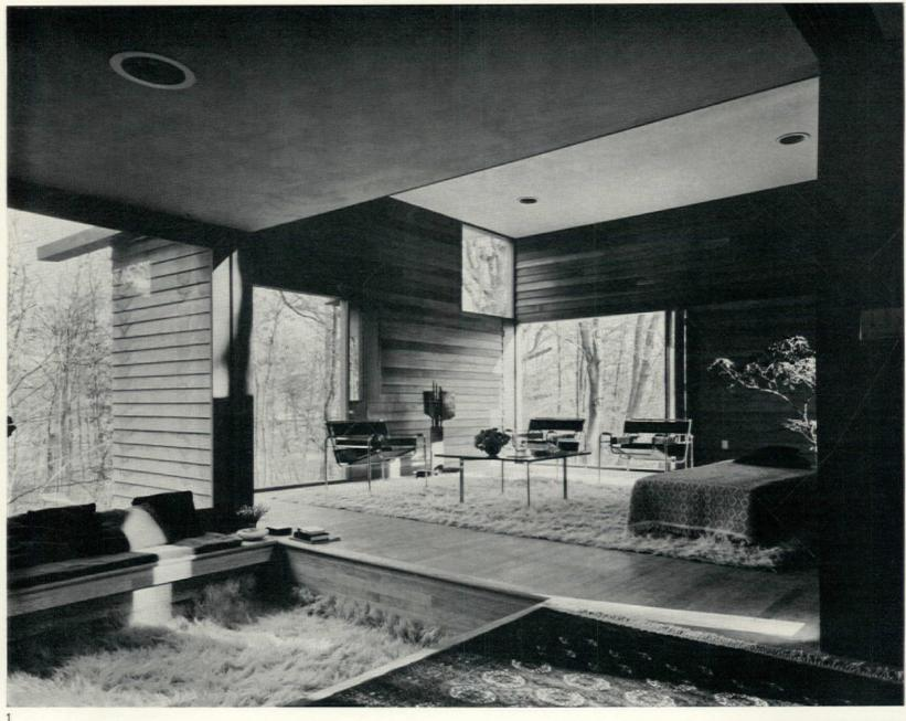
Openings are filled with fixed plate glass. Ventilation is provided by adjoining wooden vents. Where the location of glass and ventilation requirements conflict, heavy wood casements are used. Opening elements are shielded by either overhangs or plywood hoods.
