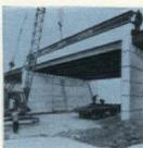
9½-hour flyover! Rapidly erected shortspan motorway bridges and flyovers: Universal beams cut erection times and costs, minimise traffic dislocation. Steelwork for Newhouse flyover (A8, Glasgow-Edinburgh) was erected in only 9½ hours. Larger AUTO-FAB beams in a range from 42 inches and up to 78 inches deep now allow very high safe loads with similar economies.
