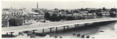
**Steel chosen for Hill Cross flyover** A further elevated section of Coventry's Inner Ring Road is to take shape in steel. Steelwork is planned to proceed quickly on this 672 ft. long viaduct. As with the now completed Moat St. flyover, prefabricated welded box-section beams and stanchions will be transported to site with stud shear connectors welded on. Steel offered lowest cost, including maintenance.
