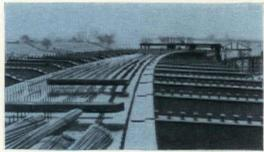
Steel elevated road Fylde Junction Higher Bridge at the 3-level Broughton M6-A6 traffic interchange. This attractively designed welded steel box girder viaduct, supported on steel piers, has a curved length of 1,300 ft. The Structural Deck (above) comprises a 14 ft. wide, 8 ft. deep, three-cell welded spine beam with 14 ft. long cantilevers on each side.
