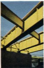
Stylish span Attractively designed steel plategirder motorway bridge. Good clean design is now achieved employing modern welding techniques, resulting in smoothly contoured, aesthetically pleasing steel bridges and other structures. New protective systems also permit choice of durable finishes in colours to suit each bridge site.
