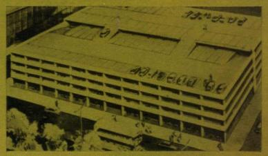
'Multi-park' Steel-framed multi-storey system reduces construction costs by maximum use of standardised structural steel components in its multiple, modular parking grid units. Factory-built sections allow quick erection of one-level, split-level, or sloping-ramp car parks of any height or capacity.
