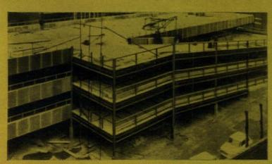
**Versatile Unit-frame System** This 'TemPark' accommodates 152 cars on an urban site for Nottingham City Council and may be re-sited in future. Basic steel units (52 ft. 6 in. x 24 ft. 6 in.) can be used for permanent or temporary car parks of varying height, shape and capacity, at low capital cost.
