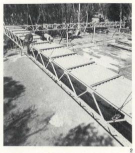
Folded truss deck sections arrive by railroad flatcar and are transferred to truck for transport to the site. Each unit is 70ft long and 5ft wide
