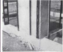
Demonstration corner section of concrete party wall as used on interlocking 'L' shaped plans.
