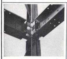
Intersection of main stanchions and main beams showing use of 2-way connector unit.
