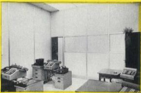
Stramit floor-to-ceiling partitions in aluminium framing sections used to construct a bright and attractive office.
