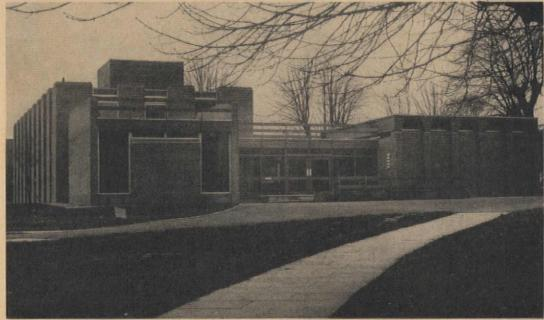
is to the right, the administrative offices to the left. In the offices U-plan brick piers provide structural support, recesses for storage, ducts and a tentative definition of work places for each occupant.
