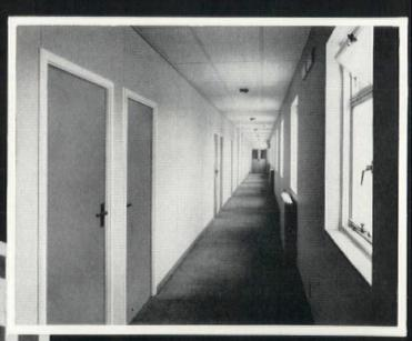
By using large pre-formed sections to construct the outer shells, towering blocks of offices and flats can now be erected in record-breaking time—but what of the interiors? Here, too, the answer is industrialization, and Stramit partitions offer a system of internal sub-division of space that is not only economical but also lends itself to prefabrication and rapid assembly on site.
