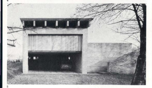
finish of the in situ frames is rough boarded, whilst the precast beams are finished smooth almost like marble. The Siporex floor slabs are 9in. Siporex has also been used for partitions in the bedrooms and bathrooms. Here it is 3in or 4in thick and covered with hessian painted white. The soffit of the floor slabs is painted light grey. This is the only paint used in the house and no plaster whatsoever has been used. Maintenance cost is thus reduced to a minimum.
