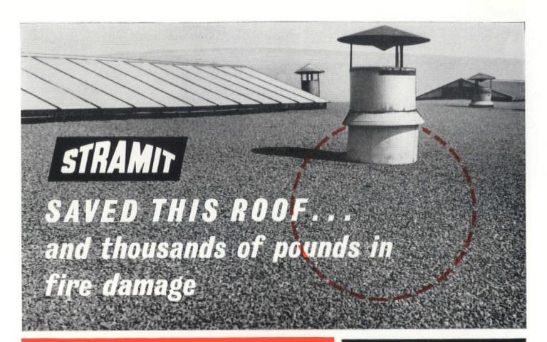
This is the roof of the polishing and spraying shop in a furniture factory, immediately after a fire in which highly inflammable solutions turned the workshop into an inferno. The area outlined was directly above the outbreak, yet the Stramit Class I Roof-Decking, supported by steel-tees, resisted the fire so effectively that the bituminous felt weathering was completely unharmed—not even a bubble was raised!
