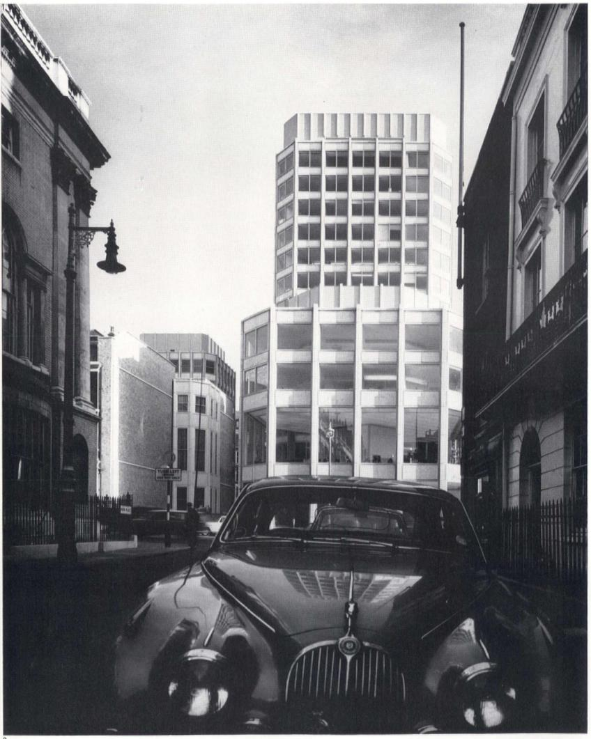
The fourth to seventh floors have one flat on each. Ventilation and lift machinery are on the roof. The escape stair is reached through an open balcony where are located the rubbish chute and dry riser.
