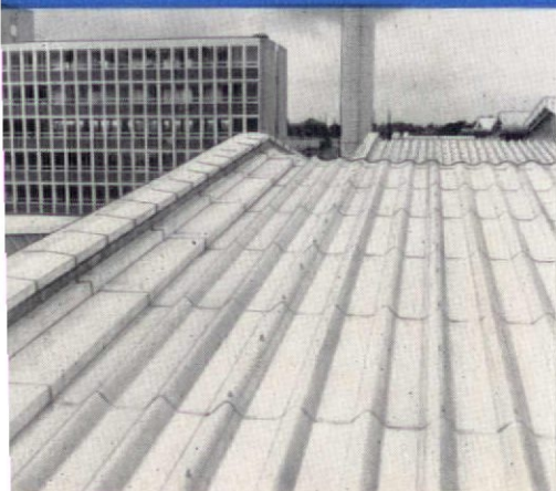
This photograph clearly illustrates the flashing detail against an abutment wall. Note the close nesting of the corrugation and the bold profile of the Fort Sheets.
