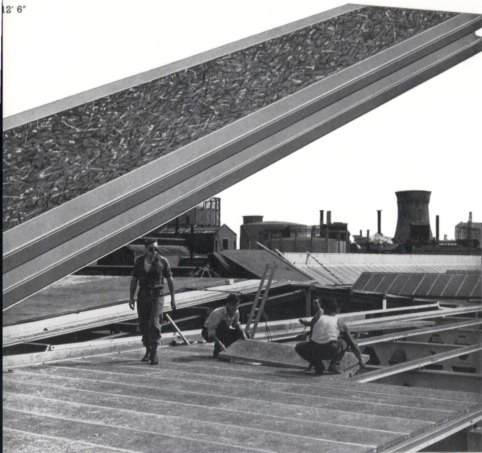
Philips Electrical Ltd. Extension at Croydon
