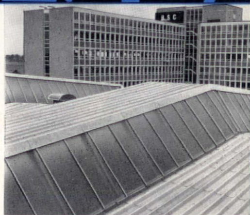
A close-up of one of the monitor units which provide adequate, even light to the extensive floor area.
