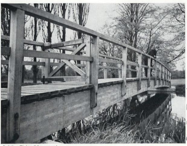
Footbridge at Winchester College, constructed by Laminated Wood Ltd., Bideford.
