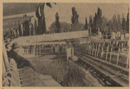
from the entrance 1. In this system entry and exit on to and off the band is via the stationary centres of circular platforms, that have the property of turning slower near the centre than on the circumference. The gradual increase in speed across the surface of these discs enables people to mount or dismount directly on to or off the moving band at the periphery.
