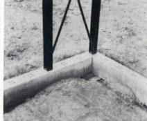
Precast concrete ground beams and braced panel of steelwork.
