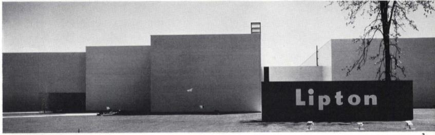
View from the north-west. The two-storey office block with its prismatic skylights. The vertical dark line is a black steel panel to give prominence to the doorway
