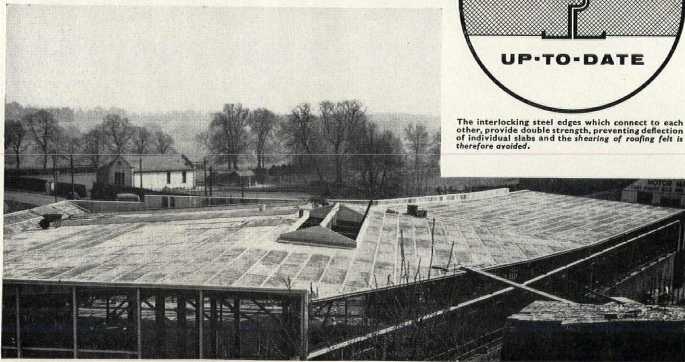
Showing ISERS as Roof Decking before laying Screed and Roofing Felt on Brown's Garage, Hamilton, Lanarkshire
