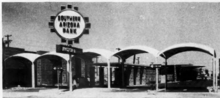
**ARIZONA'S FIRST MOTOR BANK**, designed by William Wilde, AIA, for Southern Arizona Bank & Trust Co. in Tucson, uses adobe brick, tile curtain walls and—for the first time in the country—skin-stressed, thin-shell laminated plywood formed into compound curves. Quartz terrazzo columns support the front entrance. Free traffic flow has been created by three street entrances. Drivers have a choice of four windows while pedestrians are served by a walk-up unit. Total cost of building: \$100,000.
