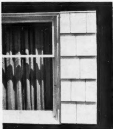
Double-crossed shingles give deep shadow lines. Joints are spaced  $\frac{1}{4}$ " apart.
