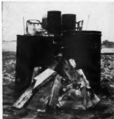
**Water has to be heated for mortar in freezing weather**
