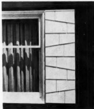
For this design, butts of shingles are trimmed on slight angle; direction changed.
