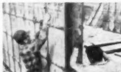
**Set Faster** — finish complete foundations in 16-24 man-hours with 2 men. Patented locking levers, bolted to panels, speed erection!
