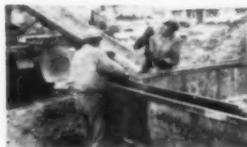
**Pour Faster** — Rigid assembly permits fast pouring. Panels won't shift... adjust to footing. Embossed steel bars on panels prevent deflection.
