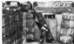
**Strip... Move Faster** — 9-ply panels (2' x 8') weigh only 65 lbs. Easy to handle. Vital parts can't be lost or misplaced... saves stripping and moving time.
