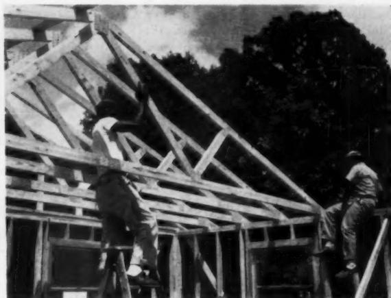
**Roof trusses are lifted and fastened into place**
