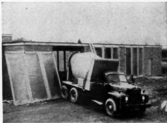
**Shields made with polyethylene film seal off openings to keep crews and concrete warm**
