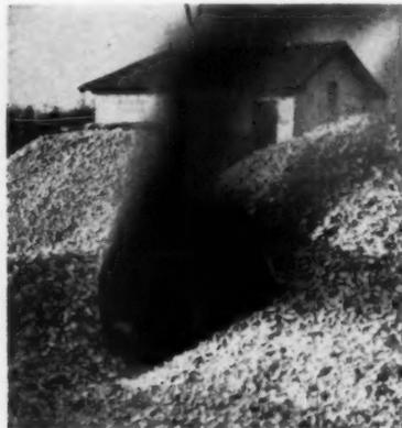
**Oil drums can be substituted for pipe to heat sand**
