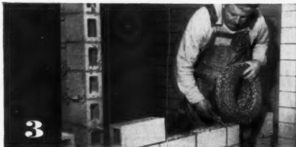
**UNIFORM MORTAR JOINTS . . .** In doing fine tile work (or any good masonry work), uniform, mortar joints are necessary. Only Keywall can be lapped without lumping up the mortar joint. That's why the architects and Crouch-Walker used it on the tile work for the Chicago Fire Academy job.
