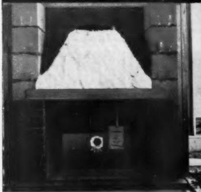
**2** Form wrapped with insulation, concrete block installed to 8" above chimney base, face masonry started.
