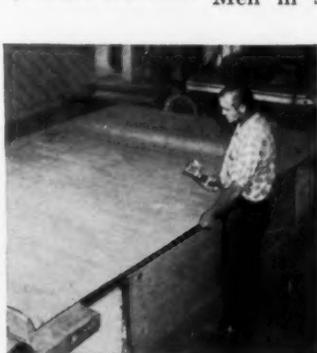
Men in shop staple aluminum vapor barrier in side-walls in a quarter hour. This was a one-hour chore with hammer and nails. At an average of 10 panels per house, builder puts an additional \$16.88 in the profit column on each house.
