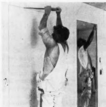
**5** DOORS are cut or placed anywhere you desire. Door bucks reinforced with 1" x 1 1/2" wood strips in space between face panels. See how Pabcowall adapts itself to your most specific construction plans!
