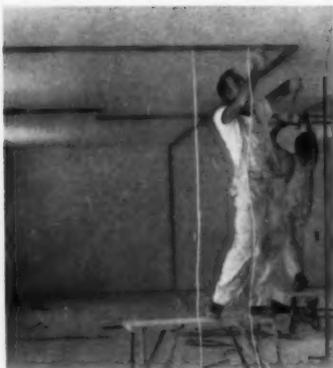
**2** **NAILING STRIPS**, 1" x 1 1/2", are applied to ceilings, floors and sidewalls. Walls are laid out according to blueprint with chalk line and level. Note how interior framing is eliminated.
