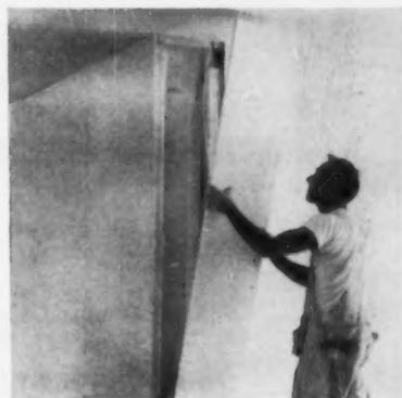
**6** WIRING IS SIMPLE, with conduit coming through ceiling nailing strips and running between face panels to outlets. Note the strong outside corner achieved with 1" x 1 1/2" wood strip.
