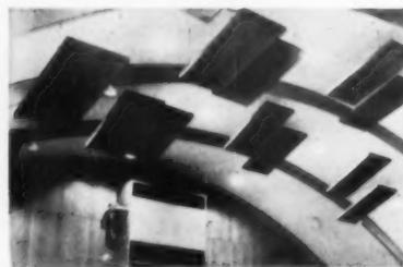
**Acoustical.** Punched Forest Sandalwood Hardboard, applied over batts of Fiberglas, rock wool or wood fiber has proved to be one of the most effective yet economical methods of controlling sound. Send for a special bulletin.
