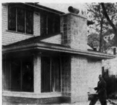
**STACKED BOND** construction gives the chimney an attractive pattern. Builder Gilhorn, at right, checks the completed job.
