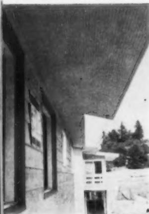
Another smart idea from C. K. Dart: by using 1/4-in. Masonite Pegboard to form his soffits, he gets two advantages: (1) the perforations provide excellent roof ventilation; and (2) the material's surface lends visual interest to large overhangs.
