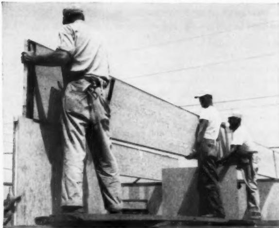
**6 Plywood box beams** act as the main roof support, have  $\frac{3}{8}$ " fir plywood skins nail-glued to 2x4 top and bottom chords and stiffeners. Projecting (or recessed) end stiffeners form tongue and groove joints over bearing partitions. Advantages of fir plywood box beams include high strength-weight ratio, design freedom, dimensional stability, easy-to-finish surfaces.
