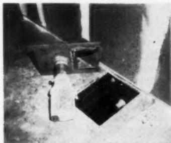
**SEWAGE PLANT** in miniature. One part: grinder installed below toilet.
