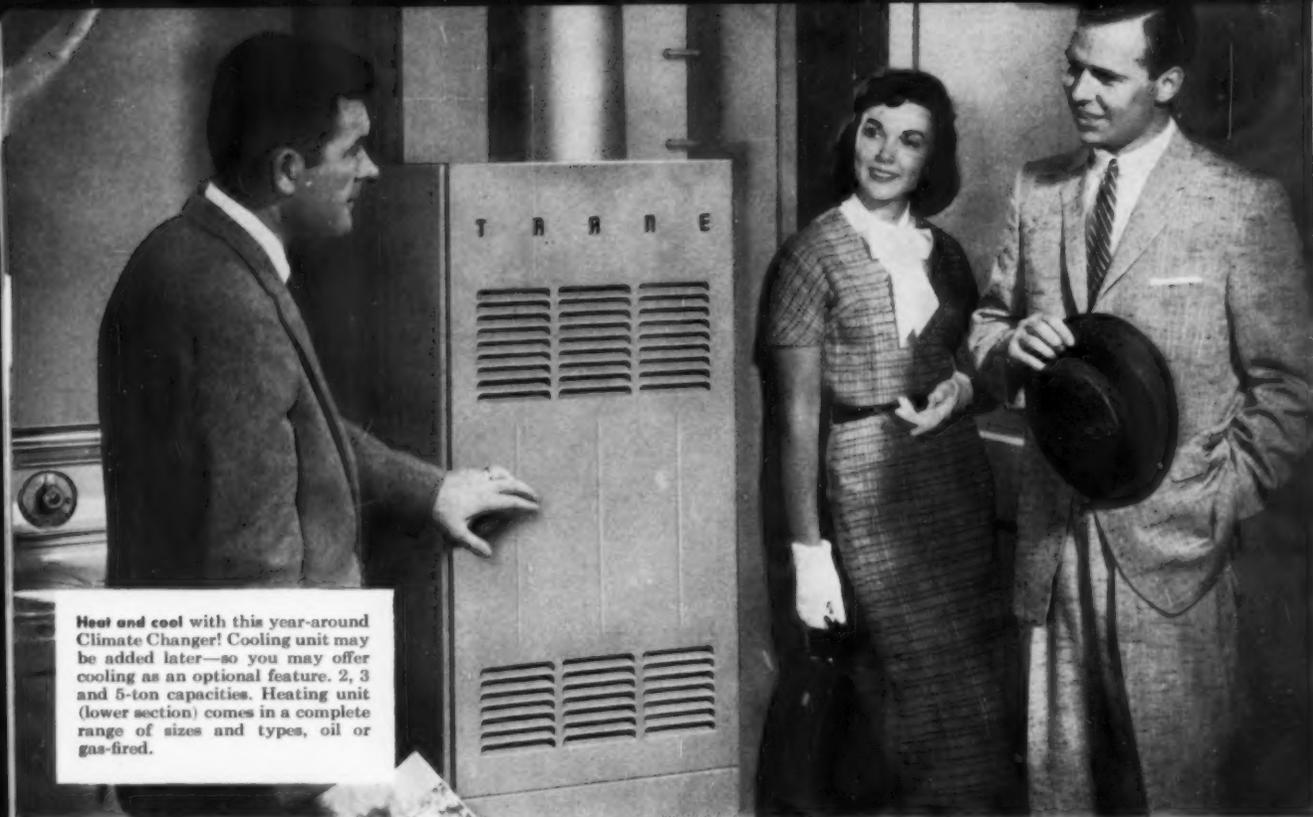
Heat and cool with this year-around Climate Changer! Cooling unit may be added later—so you may offer cooling as an optional feature. 2, 3 and 5-ton capacities. Heating unit (lower section) comes in a complete range of sizes and types, oil or gas-fired.
