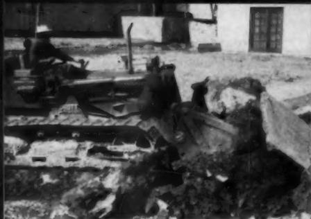
**Skid-Shovel position** applies the tremendous excavating force of pry-over-shoe break-out action—enables the International Drott 4-In-1 to "double" for power-shovel performance on a long list of jobs. This TD-9 4-In-1 is breaking up, digging up, and loading out old concrete walks and masonry curbing for Contractor Ralph Torres, El Paso, Texas.
