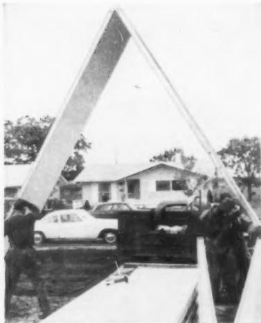
**8 Carport**, built by hinging foam-core fir plywood panels together prior to erection, cost some \$400 less than conventional semi-enclosed carport. It demonstrates cost-cutting advantages of components as well as new building forms they make possible.
