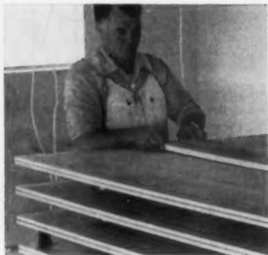
**1** **LAMINATE** strong 1" x 6" gypsum ribs to gypsum board panels. Ribs are attached on center with Pabco joint cement at a rate of one each 60 seconds. Total laminating time is only 40 minutes on average job.
