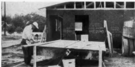
**FIRST STEP IS LAYOUT.** Precut members (these are for a soffit assembly) are placed on the trailer jig. Bed of the trailer is marked off in 8-in. increments, for 8-, 16- or 24-in. centering. This helps minimize measuring errors.
