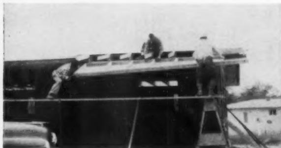
**SOFFIT OVERHANG** is lifted into place by two men. Man on the roof nails the component to walls and truss outlookers. To get maximum efficiency, soffit panels are completed for both sides, and are then installed in one operation.
