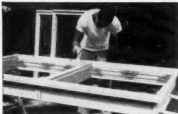
Because sash lift out for separate painting on a bench or easel, painting time can be cut in half. Frames can be primed separately. With sash removed, one man can install any but the largest R·O·W windows.
