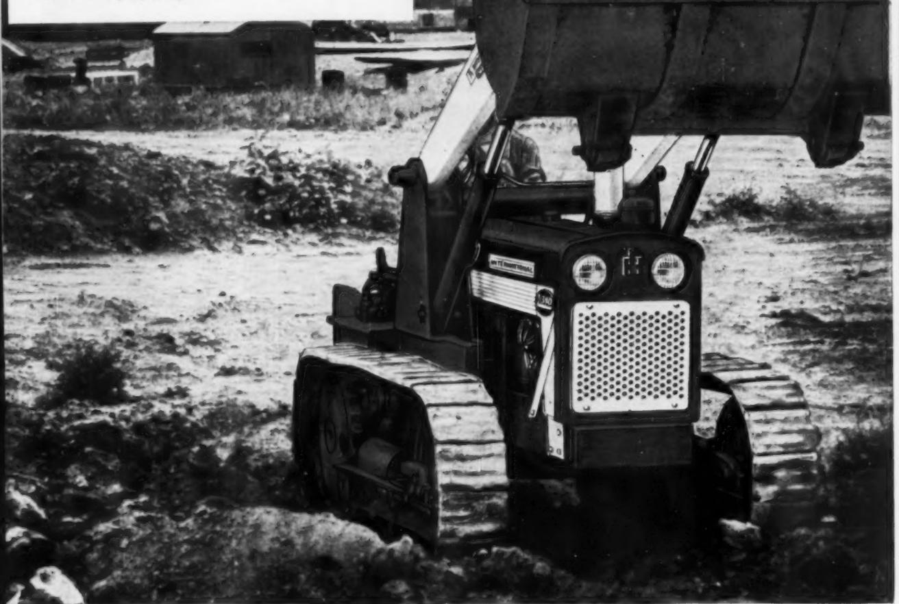
**New International Drott Four-in-One.** Only the new T-340 offers this versatile, high-production unit in the utility crawler field! Left below, showing exclusive clamshell action for "surrounding" materials, or dozing close to green foundations without excessive ground pressure. Right, bottom-dump action provides 9 ft, 6-inch
