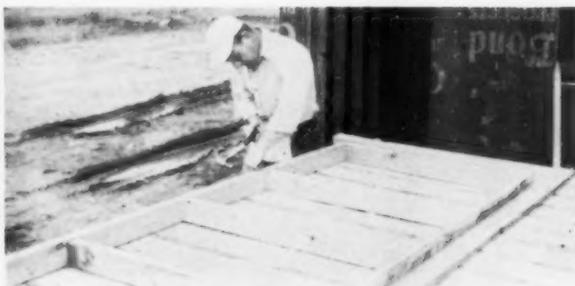
**SECOND STEP IS NAILING.** 2x4 members are placed over approximate mark and nailed up. Note 2x4 backing on trailer bed. It permits one man to nail panels against it. Also note how trailer's height permits man to work without bending over.
