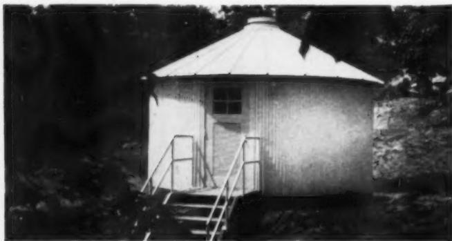
**COMPACTNESS** is a major advantage of the small treatment plant. This housing is all the cover necessary for Dorr-Oliver's 15,000-gallon Complete-Treater unit. The installation is for a small military base.
