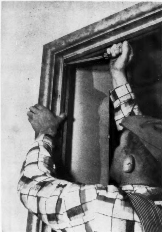
Lock into place by turning screw at top of strike jamb (patented assembly).
