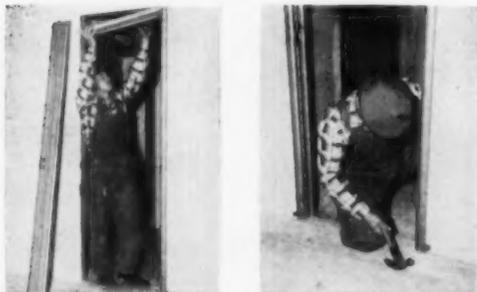
Snap hinge jamb over stud and wallboard. Snap header into opening with hinge jamb. Install strike jamb same as hinge jamb.
