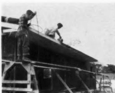
**FINISHING OF THE CORNICE** now involves merely finishing the roof over it. In photo above, one man uses a power hand saw to trim edge of sheathing along soffit. Man nearest the camera is feeding the saw's electric cord.
