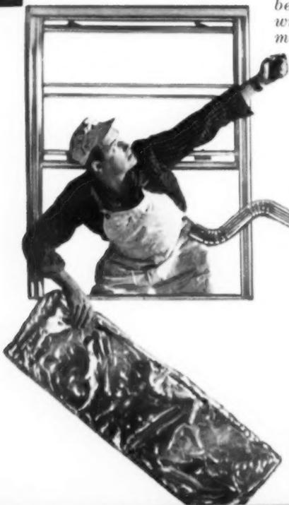
*The downspout and the gutter on the right demonstrate the ease of handling aluminum rain-carrying equipment. Important advantage is freedom from rust — no painting.*
