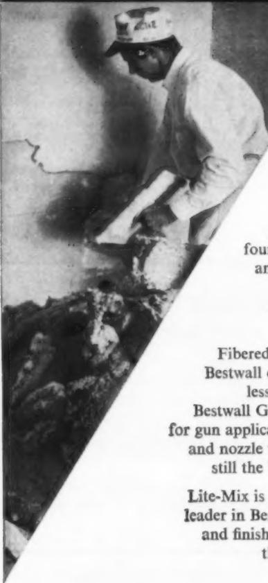
Expanded perlite is mixed at mill to produce Bestwall Lite-Mix, a basecoat plaster that, compared to ordinary sanded gypsum plasters, is 50% lighter, provides four times as much insulation value, and gives higher fire resistance. To use Lite-Mix, add water only. Available Fibered, Unfibered, or Masonry Mix.
