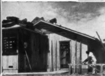
Rowland Van Ness used Exterior fir plywood and batten siding to eliminate all sheathing, bracing and blocking.
