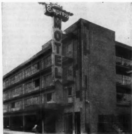
**A**luminum curtain-wall panels enabled the J & L Construction Co. to cut 50 per cent from the wall-erecting costs of this four-story Atlantic City motel. The panels were shipped to the site knocked down, merely had to be assembled and set on the job.
