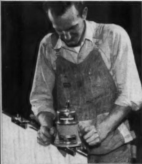
**THE CARPENTER-SIZE ROUTER!** This is one heavy-duty router designed with the carpenter in mind. Easy to handle. Light-weight—just slightly over 5 pounds. Full  $\frac{1}{4}$  hp motor has power to spare. 23,000 rpm spindle speed gives smoothest possible cuts on any routing job. Assures accurate, fast jamb mortising when used with new SKIL No. 17070 Hinge Butt-Template Kit shown.
