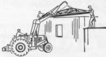
**YOU CAN SWING** wall panels and trusses into place with another type of attachment that will make a crane out of the loader. Booms are available to lift moderate-sized loads as high as 22 feet.
