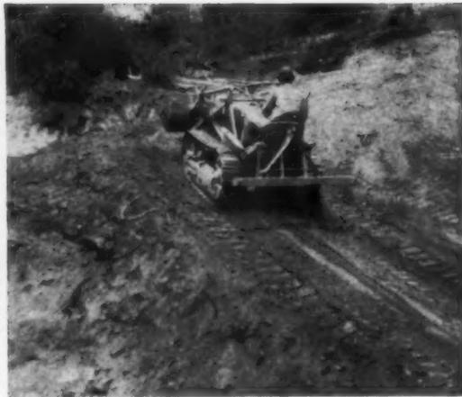
**CRAWLER LOADER** moves up incline to site. Operator can go over very rough ground by moving slowly. On easier ground, a wheeled tractor could do the job faster (see Land Planning, p. 190). Barcus used to rent a crane for this task, saves \$10 an hour with crawler.
