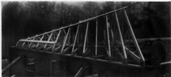
. . . HIP ROOF BEGINS to take shape as succeeding trusses are installed. Trusses are 2 ft. on centers, but are 2 ft. 10 in. apart along the plate.
