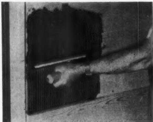
**2 MORTAR IS GROOVED OUT.** It must be spread as thin as the trowel notches will permit. The new material will bridge relatively deep hollows and still provide a firm tile bed.
