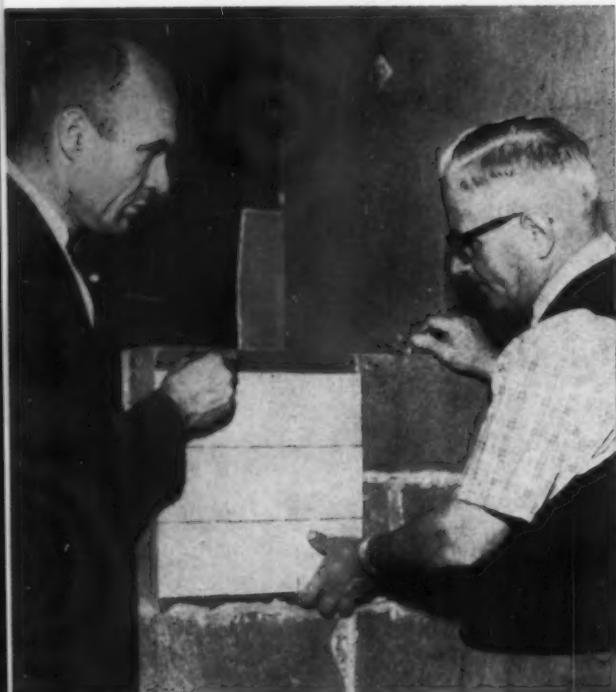
**EVEN A ROUGH-SURFACED** concrete block wall makes a good tile backing with new dry-curing, thin-set mortar. Here editor Lou Vorse learns how to use it from John Stefano, at TCA's research center.
