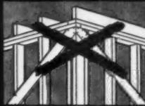
You save on material, labor —with this new USG Sheathing. Vertically applied in 4' x 8' or 4' x 9' panels, it eliminates need for let-in corner bracing... meets
