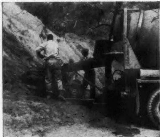
**LOADING CONCRETE** into ½-yd. loader bucket. This is as close to the site as the mixer truck can go. Barcus (back to camera) helps handle the chute. He's not in the habit of doing his own concrete work, but keeps close to the cost and methods used by his subs.
