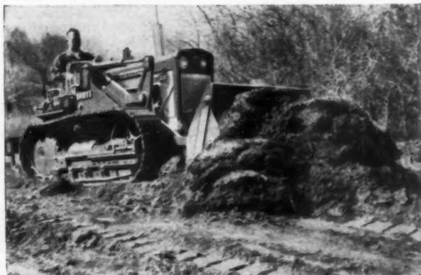
**New International Drott T-340 Four-In-One Skid-Shovel**—combines in one machine a bulldozer, clamshell, carry-type scraper, and  $\frac{3}{4}$  cu yd bucket ( $\frac{1}{2}$  cu yd heaped), all hydraulically controlled.
