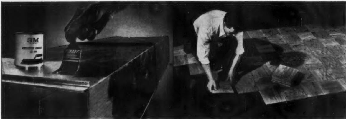
**UNUSUALLY HIGH COVERAGE.** Insulation adhesive EC-104 covers up to 200 square feet per gallon when brush applied. Goes on quickly, easily, uniformly. Provides fast grip even when wet. Open time: up to 20 minutes when both surfaces are coated.
