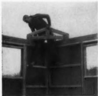
ENDS of first small truss are placed exactly 4 ft. from corner . . .
