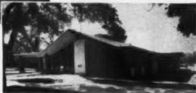
■ The use of Rilco beams for St. Joseph's Catholic Church "was premised on cost factors as well as appearance considerations," states the architect. "We found the Rilco people very cooperative (and) despite snow and wet weather, no delay was experienced in the erection of the arches."
