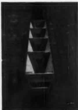
Bearing-wall beam is shaped with this form. Here, rods and vapor barrier are in place, awaiting concrete.
