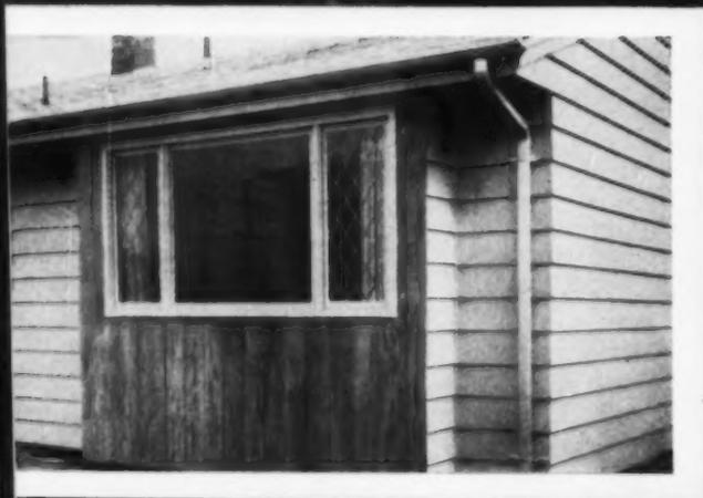
**OUTSIDE**, the bay fits snugly below existing roof overhang. Foundation didn't have to be altered, because the projection sits on cantilevered floor joists. Bay could be added to an existing structure very easily.
