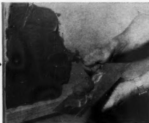
**1 MORTAR IS TROWELED ON**, then spread evenly. Adding one or two parts sand for each part of Formula 756 will increase workability, cut costs, but won't weaken the final bond.
