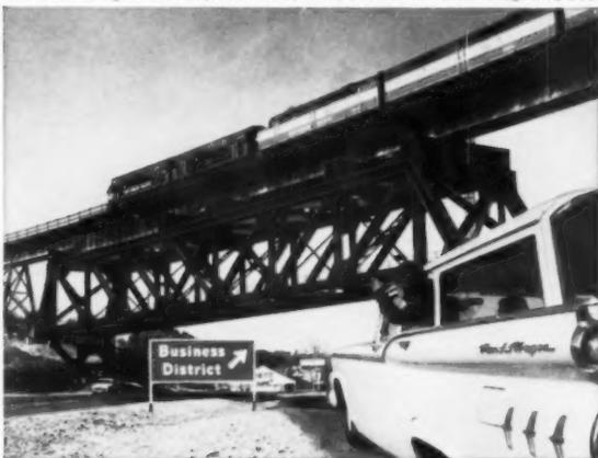
**New Lift for Old Bridges.** A revolutionary new construction idea—a “piggyback” bridge to carry an existing railroad bridge over heavily-traveled Highway 40 at Auburn, California. The new bridge of USS Structural Steel replaces supporting towers and provides a 240' span for uninterrupted traffic flow on the widened highway below.
