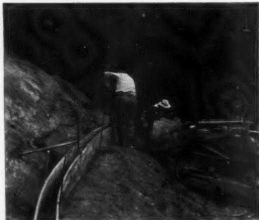
**AT SITE**, concrete is moved from the bucket into the forms for an interceptor ditch. Normally, the concrete is dumped directly into the forms, but in this case, the narrow space between boards made it necessary to transfer the material by shovel.
