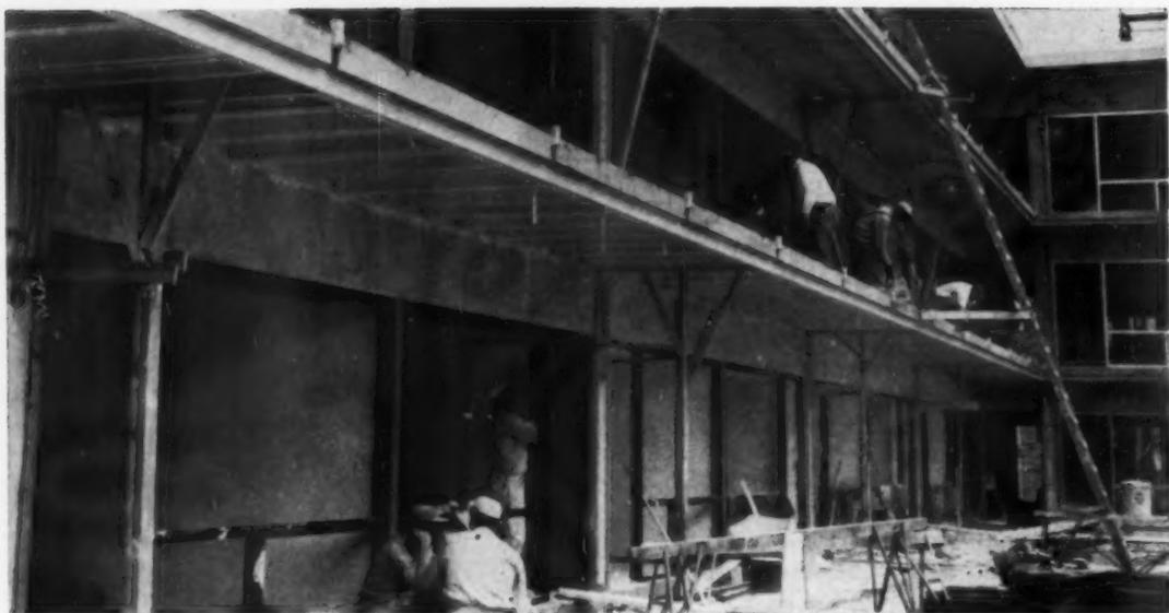
THE EMPRESS MOTEL'S frame is of pre-cast concrete. Here curtain-wall frames are being installed. Doors, glass,
