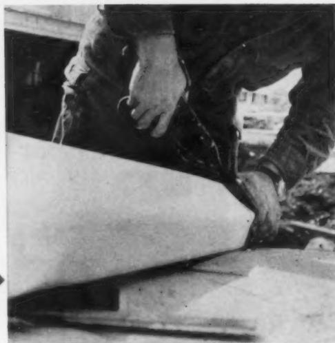
**GUTTER SECTIONS** are cut to proper length with tin snips, as shown, or with a saw. Spout holes are located, then cut, using a template supplied with the kit. System is now ready for installation.
