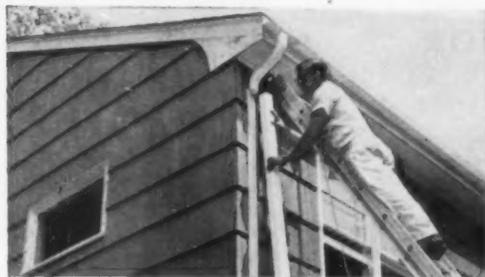
**JOB NEARS COMPLETION.** Elbow is attached to drop outlet, and the base section of the downspout is nailed to the house, as shown. Downspout snaps onto this base section, requires no bonding.
