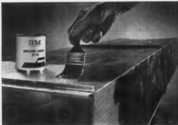
**UNUSUALLY HIGH COVERAGE.** Insulation adhesive EC-104 covers up to 200 square feet per gallon when brush applied. Goes on quickly, easily, uniformly. Provides fast grip even when wet. Open time: up to 20 minutes when both surfaces are coated.
