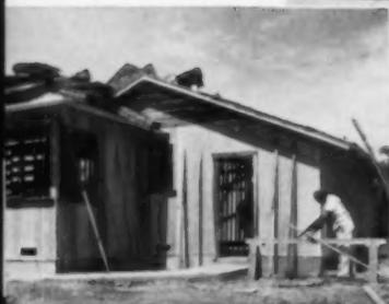
Rowland Van Ness used Exterior fir plywood and batten siding to eliminate all sheathing, bracing and blocking.
