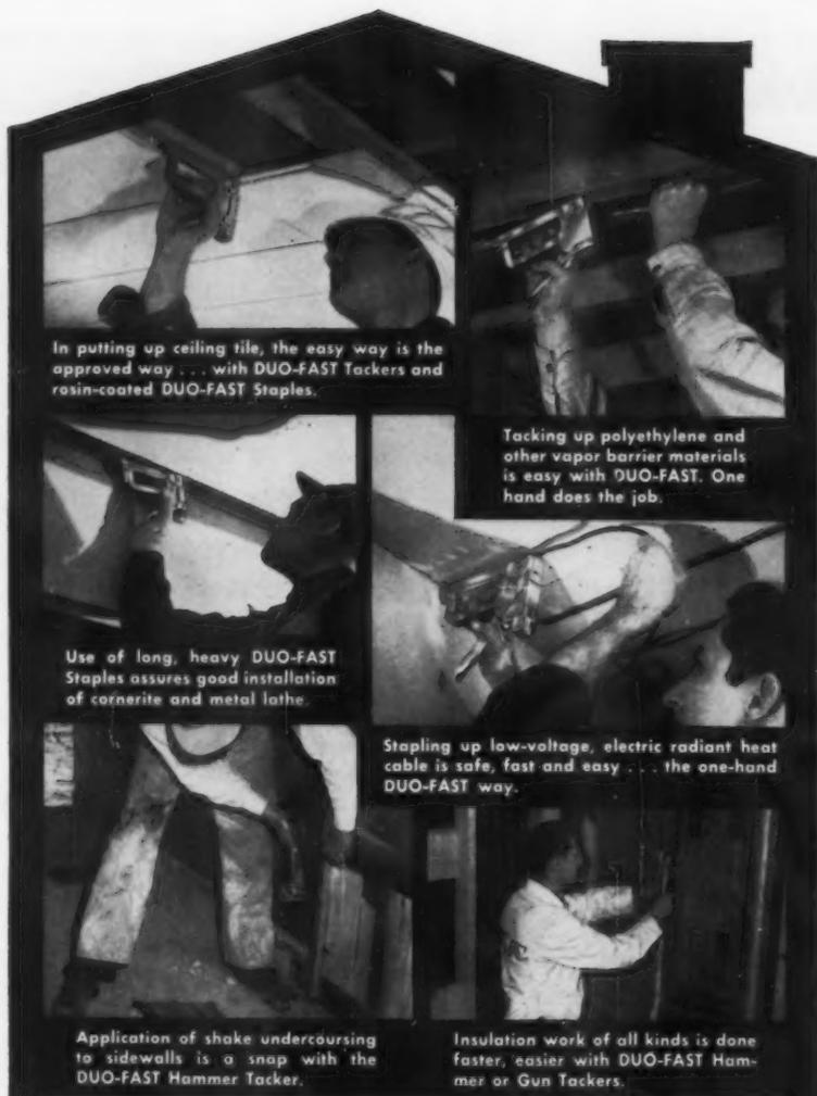
In putting up ceiling tile, the easy way is the approved way . . . with DUO-FAST Tackers and resin-coated DUO-FAST Staples.
