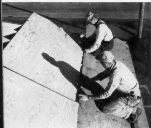
The combination of PlyScord and Plyclips is credited with making possible a 50 per cent labor savings on this 31-building New Hampshire public housing project. Over 160,000 sq. ft. of plywood was used for both wall and roof sheathing.
