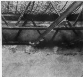
**1.** Galvanized-steel main runners are attached by means of steel clips to the undersides of steel joists.
