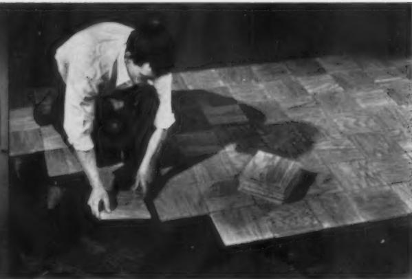
**STRENGTH, DURABILITY.** Adhesive EC-194 bonds wood blocks to above-grade concrete or wood subflooring indefinitely. Suitable for use on radiant-heated floors. Water-resistant EC-194 grips immediately, dries rapidly. One gallon covers about 40 sq. ft.
