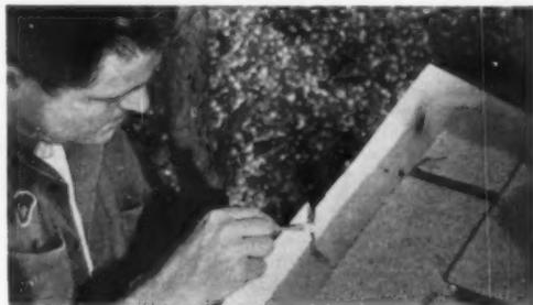
**THE SECTIONS** are overlapped, then joined with a bonding agent. A coupler is supplied for joining sawed lengths. After gutters are in place, drop outlets are bonded into the spout holes.
