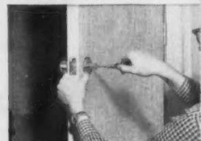
Outside trim slips on easily, pre-assembled screws are quickly tightened, rose and knob into place — and the lock is completely installed.
