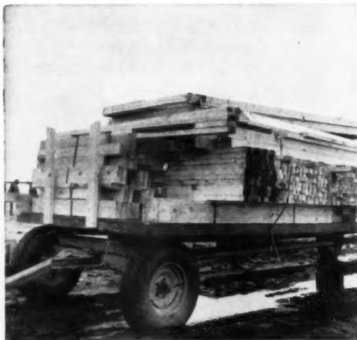
**F**raming is precut and color-coded to reduce site labor, eliminate guesswork in selecting the right piece. It is packed in steel-strapped bundles (trusses are put into special frames). A crane lifts the bundles
