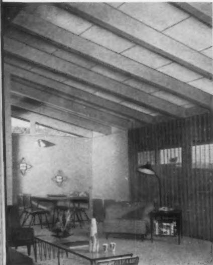
Ideal for modern exposed-beam construction, this one product combines roof deck, insulation, sound-quieting, finished ceiling and continuous vapor barrier. VAPOR SEAL TYPE: 2' x 8' in 2" and 3" thicknesses. STANDARD TYPE: 2' x 8' in 1½", 2" and 3" thicknesses.
