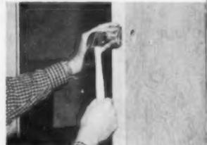
Faceplate marker fits in edge hole and with a hammer quickly outlines mortise for face and strike. This accurate mortise mark eliminates chance of errors.
