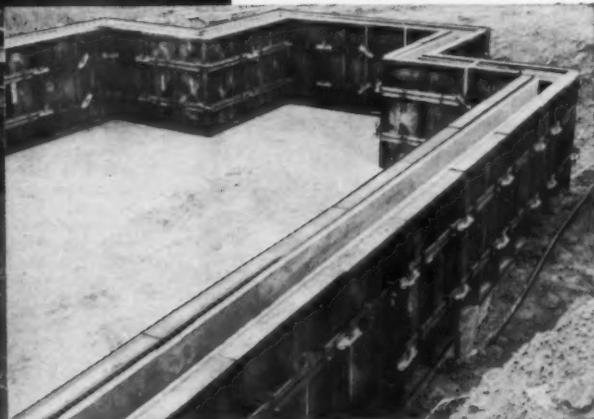
Rocform Systems are easily adapted to any type of forming job. Absolutely no alterations to the standard Rocform panels are ever necessary to form any type angular wall.
