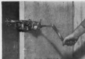
Bit guide clamps on door in seconds, locates cross holes for 2 1/4" or 5" backset, guarantees perfect hole alignment. Chip cutter eliminates splitting on breakthrough. Threads on bit engage bit guide for positive lead of bit through door.
