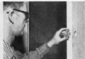
With holes bored and mortise made, latch easily fits into place. And this standard Dexter lock accommodates every type of Dexter lock.
