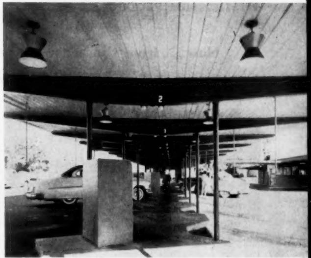
**SIMPLICITY OF CONSTRUCTION** is shown in this close-up of car shelter. Timber-framed canopy was used instead of metal because of lower costs, easy maintenance. Covered walk at right of photo leads to restaurant building. It took less than a month to build this shelter.
