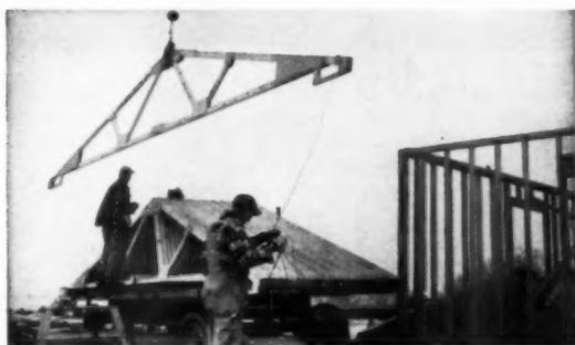
**P**hoto shows a truss being lifted from the trailer. Man at left hitches the crane hook to the truss, man at right holds guide line, which prevents truss from swinging, guides it into exact position. Drawing
