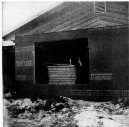
Three man hours per house are saved by putting gypsum wallboard into the house through the rough opening for the picture window. Back filling is carried to wall, truck backs right up to the window.
