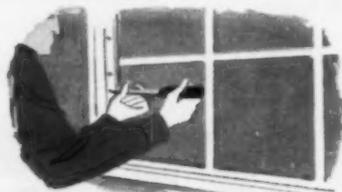
Anchor window in accordance with manufacturer's instructions, providing enough clearance at sill where under-screen operator is used. Care should be taken not to twist or distort window by pulling too much on one side. Sash should be locked in closed position during entire installation.
