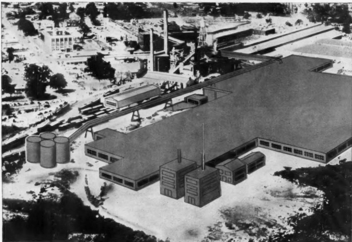
Shown (in color) are the new manufacturing additions to the Masonite plant at Laurel, Mississippi, which include new production lines, a new 26-boxcar loading dock, new research laboratories, new power plant, new office buildings and a revolutionary new raw-materials handling system.
