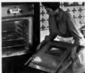
**Removable oven door** makes it easy to reach any part of oven for cleaning. Open door, release safety latch, slide door off. Slides back on as easily.
