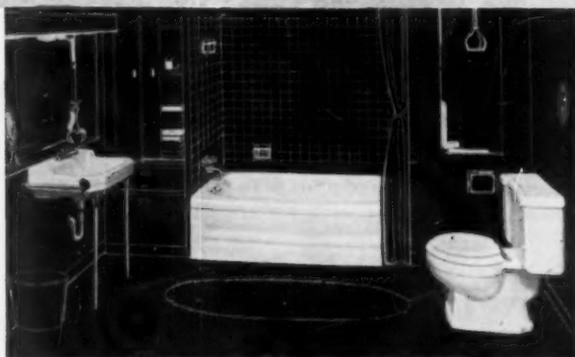
**Bermuda Deluxe Bathroom**, designed and built for The Mighty Middle. Gerber packaged bathroom No. 2. Ledge-type lavatory, No. 380, 20" x 18", has centerset with aerator and pop-up drain, No. 143A. Closet is deluxe unit-type, reverse trap, 12" rough-in, No. 1200. Porcelain enameled steel recessed tub, No. 05, with 3-valve bath and shower diverter, No. E4802, and trip lever drain, No. 181G.
