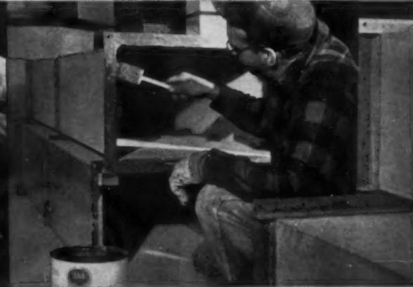
**FLEXIBLE** Sealer EC-800 for heating and air conditioning ducts can be stretched twice its length before breaking when dry. Sets up firmly at duct joints; won't flow out under pressure. EC-800 can be applied with either brush, flow gun or putty knife.
