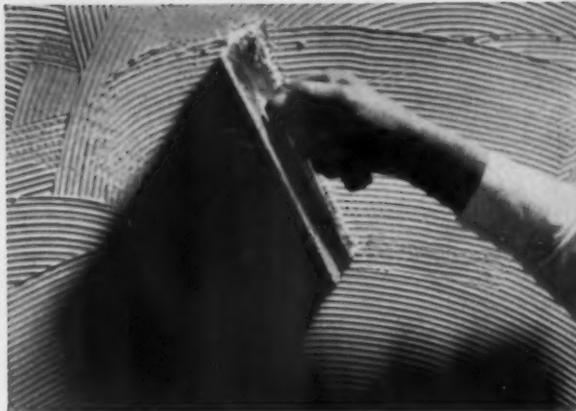
**EXCEPTIONALLY WATER-RESISTANT** ceramic tile adhesives provide fast bond-strength build-up, yet offer ample open time for work at normal pace. 3M tile adhesives trowel like butter, permit grouting on the same day. Test CTA 11 and 12 yourself!
