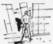
Inner and outer forms are set simultaneously. Tie rods are positioned... locking levers tapped... forms go up "a foot a minute." No other forms set as fast, as easily, as accurately.
