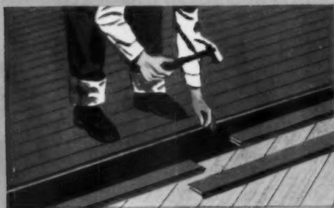
**Simplest of all floors to install, Oak is nailed to subfloor in wood joist construction. Modern Strip Oak Floors are precision manufactured in a variety of sizes and grades to suit any building requirement.**
