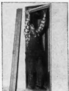
Snap hinge jamb over stud and wallboard. Snap header into opening with hinge jamb. Install strike jamb same as hinge jamb.
