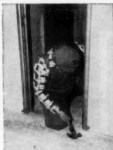
Nail bottoms of jambs at strap anchors . . . only 4 nails required (baseboard covers strap anchors).
