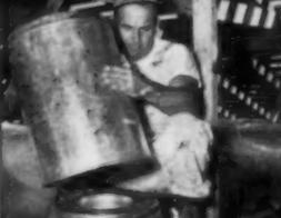
Simple "Twist-Lock" Coupling Eliminates Screws, Cement, Mastic
