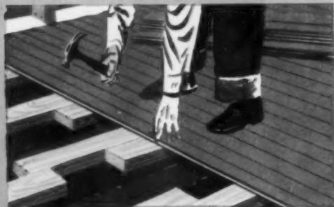
**Screeds laid in mastic provide nailing surface for installing Strip Oak Floors in homes built on concrete slabs. Write National Oak Flooring Manufacturers' Association for free installation manual.**
