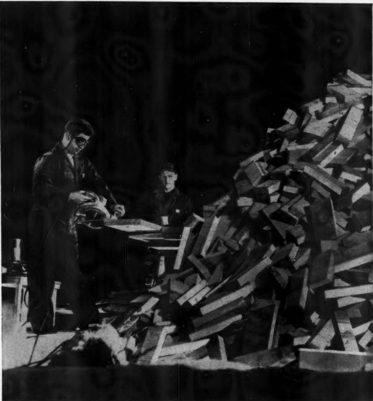
**Test continues through the night:** After twenty-four hours of on-the-job service, the saw was still in top operating condition. It was then put on laboratory testing machine to continue this grueling ordeal for another 6 days and nights. Entire experiment was under impartial supervision of the United States Testing Company, Inc.,\* a leading independent laboratory. \*Report No. 37135, Nov. 27, 1957
