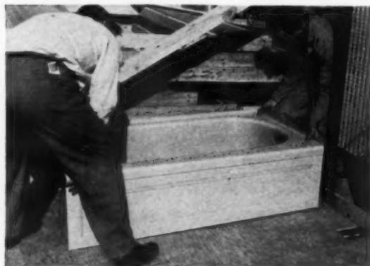
**4** TUB SLIDES into place. Vertical flange around edge goes behind tiling lip, which hangs below wall board.
