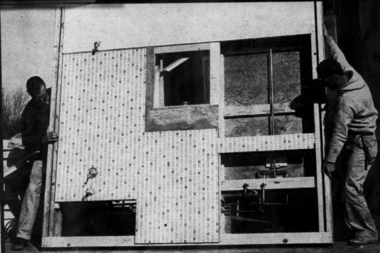
**3** CORE of the bathroom package is this wall, which holds all the rough plumbing for two baths. Other
