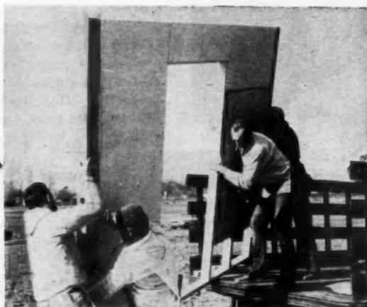
**2** FRONT WALL is unloaded. Open area under tiling is where tub will fit; rest of panel is dry walled.
