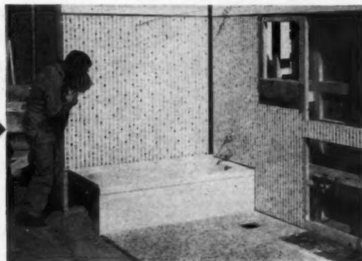
**5** BACK WALL is put up. Note that tiled floor has been set; it also arrived in one pre-tiled piece.
