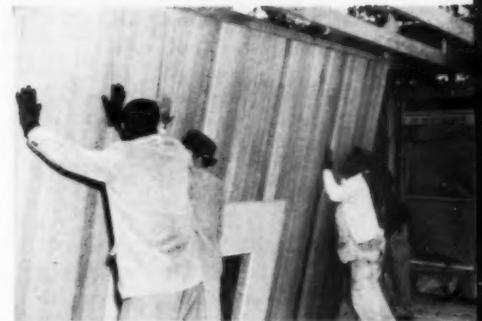
PREBUILT paneled wall with fireplace opening is set up in front of the shell and the furnace unit.
