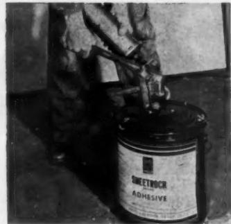
**CAULKING-TYPE** gun is loaded from 5-gal. can with an Alemite pump. Nozzle of gun is cut at 45 degrees. Angle determines position of gun while workman applies adhesive.
