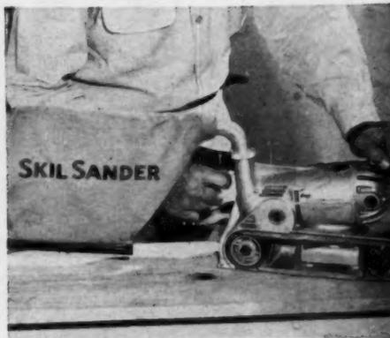
**PORTABLE HAND SANDER** can go anywhere on the job or be used on the workbench. Above, a Skil model with bag (No. F53, p. 124). Rotating floor sander is another "standard" tool.
