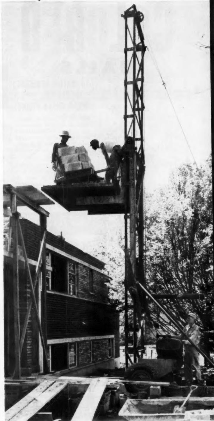
**HOISTING MACHINE** reduced man-days from 37 to 13½ on third level of second building Ulrick built. Third level of first building was built by carrying building materials up a ramp.
