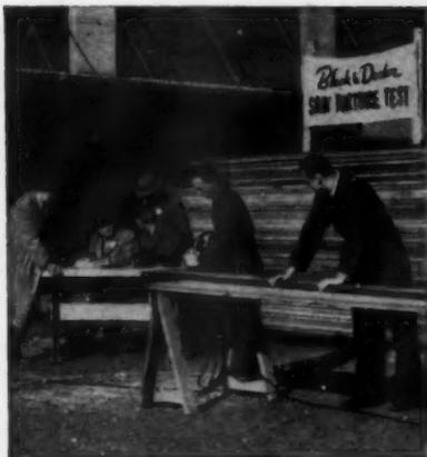
10:05 A.M. The test begins. Making a variety of cuts, the Black & Decker Saw will get rugged, continuous on-and-off use in 2" lumber.
