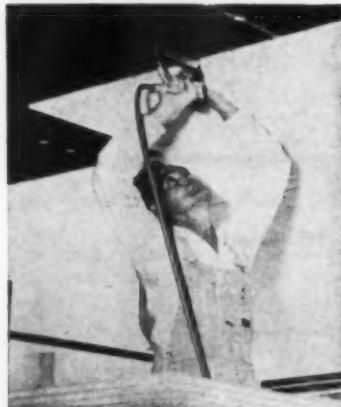
**ACOUSTICAL TILE**, wallboard and a hundred other materials are secured quickly, firmly with a power tacker. Here, a compressed air tacker, from Fastener Corp. (No. F54, p. 124).
