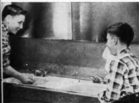
**WASHING CONVENIENCE** in this bathroom from Universal Rundle's new twin-bowl, one-piece, Dulavoir lavatory. (No. 5048 on page 132.) One-counter opening and single mounting frame take this compact 45"x17" unit. Other conveniences for the bath: ventilating fans, sun and heat lamps, more mirror space.
