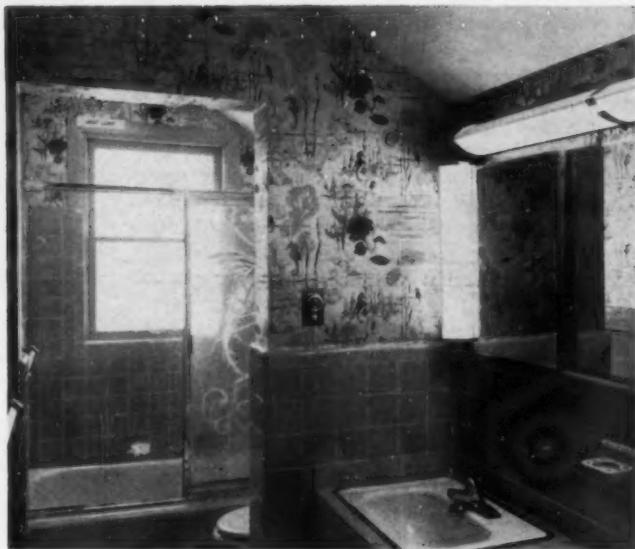
**AFTER:** The new compartmented bath. In the shower ceiling: light, heat, a fan. Over the basins: new fluorescent lights.
