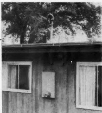
**WEATHER-CONTROL SYSTEM.** This outside thermostat, which is really an "anticipating" control, is only part of the electric heating system. This versatile house has five different applications of heat. Each technique has been placed in its particular place for its suitability and use. All are controlled from a master switch. This outside thermostat is connected to an inside unit, and acts as a steady temperature regulator for the house in winter and summer.
