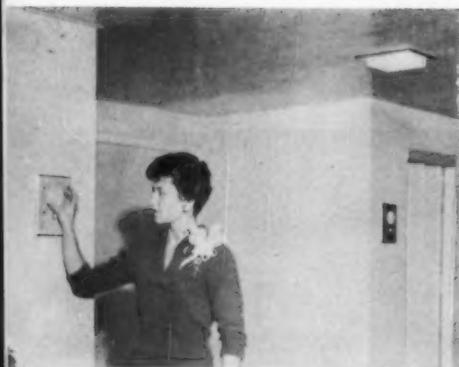
**A SURE-SELLER** for any house is specially designed lighting. The master control, besides being able to turn the lights off and on throughout the house and yard has another feature—a dimmer control by Luxtrol. By turning a dial this control can produce various intensities of light from very dull to reading levels. It works for the valance lighting in the living area. In the kitchen, lights were designed to be completely shadowless, so work could be performed with ease.
