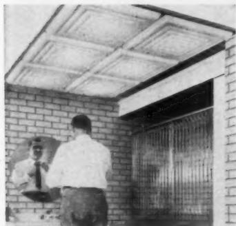
**MODULAR LIGHTING** in panels of 2'x2' or in complete Sunshine Ceiling package for standard 5'x7' and 5'x8' bathrooms. Ceilings "float," do not touch walls, allow ample air circulation. Electrical channels attach to structural ceiling with grid to hold diffusers. Wakefield Co., Dept. AB, Vermilion, Ohio. (No. 5003, p. 132.)
