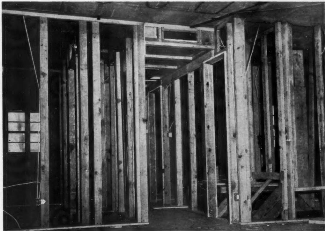
**WIRING IS ROUGHED IN** and dropped to proper location before outside walls receive insulation and rock lath, and ceiling receives lath and radiant-heating tubes. Room partitions and hall plenum for optional cooling, and
