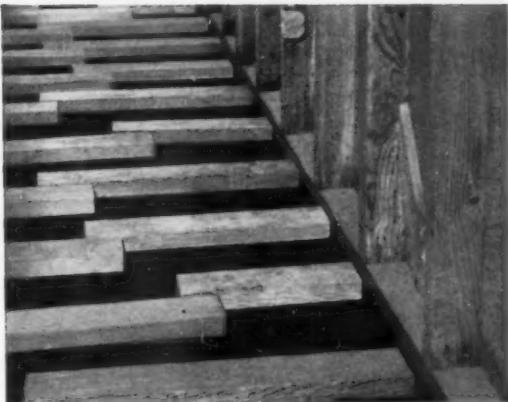
**Random-length screeds** are laid in a staggered pattern. The asphalt mastic anchors them permanently to the slab. Flooring is nailed to screeds and sanding and finishing follow in usual manner. Prefinished flooring may be used.
