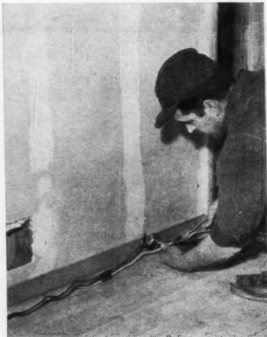
◀ **JOB STARTED:** Baseboard-style electrical strip assures a flexibility of outlet location for homeowner. Going in here: Plugmold system, used by Allen Construction Corp. near Harrisburg, Pa. First photo (left) shows Plugmold base fastened to wall; electrician splicing feed wire to run from control panel to Snapicoil. Outlets every 60 inches.
