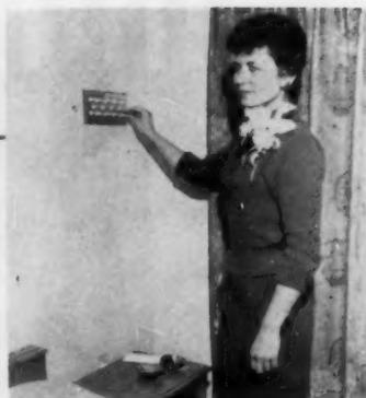
**ONE GIMMICK BUYERS GO FOR** is a master control panel. This one in the Electri-Living house is located in the master bedroom and has a Remcon low-voltage light control wired into it. A flip of the switch turns lights off or on in other parts of the house or yard. A dimmer switch, wired to the control, can produce several light levels. The panel works off the 400-amp center. Throughout the house, lighting was planned to be functional, and to enhance the decor.
