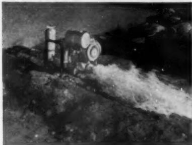
**Carryable Diaphragm Pump . . .** This self-priming, 120 pound diaphragm pump will handle water in the thickest sand, muck, or mud. Capacity: 5,000 g.p.h. Size: 3". Complete line of centrifugal pumps are also available in sizes from 1½" to 3".
