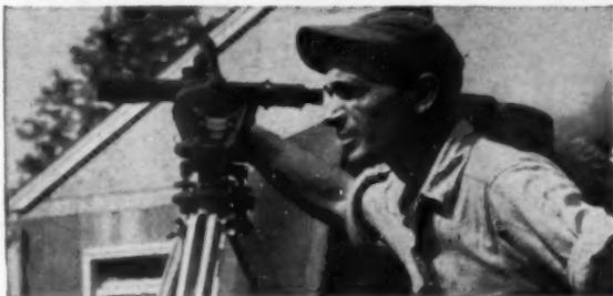
Newly designed optical system in this latest model Berger Convertible produces clear, sharp image over long sights as well as at close distances. Internal focusing 10½" telescope with 22-power coated optics views image *right side up*. Sensitive telescope vial *plus* plate level vial assures accurate leveling. Verniers read to 5 minutes on horizontal circle and vertical arc; leveling, clamp and tangent screws are dust protected. Sturdy brass and bronze construction.
