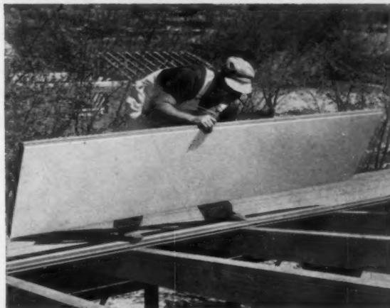
**For commercial buildings**, like this economical warehouse, showroom and office, Insulite Roof Deck saves real money, speeds construction. Crossley applied beams and Roof Deck to this 6,000 sq. ft. building in just 72 man hours, held cost of the building to \$6 per sq. ft.
