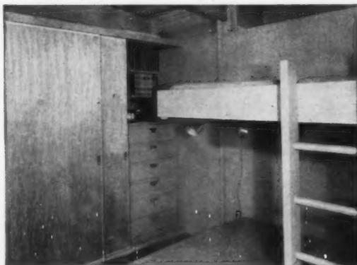
*Carport storage* makes up for lack of bulk storage area in garage or basementless homes. Exterior plywood lockers for garden and patio gear fit trend to outdoor living.
