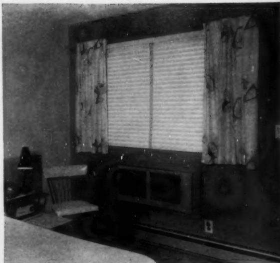
**BASEBOARD HEATER** permits full carpeting. Basic unit is 32" long, 8½" high, 3" deep, with 600-watt capacity, operating on 120 or 240 volts. Air conditioner fits into sleeve under window.
