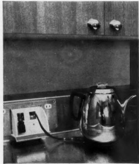
**6** **START YOUR COFFEE** from bed—outlet and retractable cord panel in GE kitchen unit can be turned on from master bedroom which controls switches outside, in garage, hall, etc.
