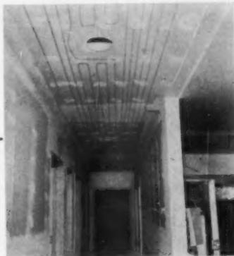
**HEAT CABLES** in the ceiling provide electric radiant heat for the hallway. They are only one segment of the house's system. Wall thermostat, connected to outside thermostat, and the master control are also located here. Besides the hall, the family room, kitchen and living room are warmed by ceiling units. Other heat applications are found in the three bedrooms which have baseboard units. For quick concentrated warmth, the baths have wall heaters.
