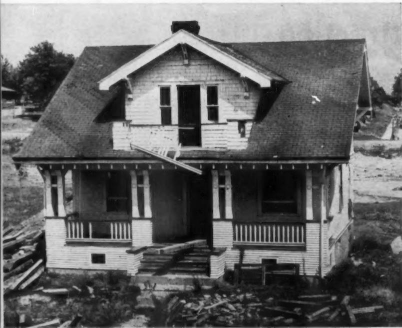
**BEFORE:** This house is an unfortunate example of the early 1900's. The picture and the plans show its obvious deficiencies; what isn't visible is the heating system (there wasn't any central heating) and the electrical system—a 15-amp, four-circuit antique that was just barely enough to handle the lighting.
