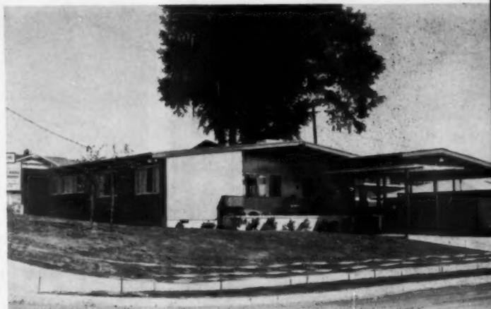
**LOW-SWEPT LOOK** is achieved by continuous eave lines of rear and front elevations. Back and front have an 8' overhang which offers weather protection. The interior, 1,470 sq. ft., was planned to provide efficient living. Note the wiring system.
