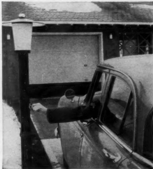
**2** GARAGE DOOR OPENS at turn of key in Genie Lift-a-door switch (\$100 installed). Latticed gate opens on patio-carport.
