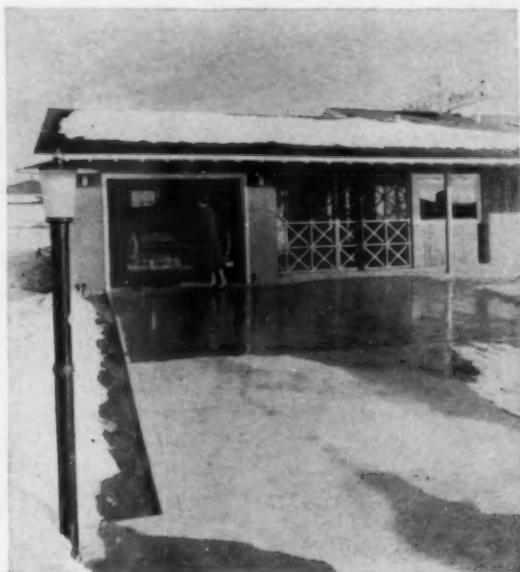
**1** DRIVEWAY has snow-melting 800-watt Electro-mode cable (\$45 for material and labor). Garage has fire alarm, time-set auto-motor warmer.
