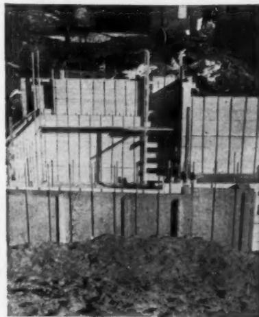
Foundation plans for this brick tri-level specified 19 different elevations and many wall irregularities. To form the tricky foundation easily and economically, Morris Bros. Construction Co., Denver, Colorado, used Gates Vertical Rod High-Wall System, with a unique combination of 3/4" plywood panels for the exterior and S4S sheathing for the interior.
