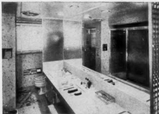
**HEATING PLUS LIGHT** for this bathroom comes from Nutone's Heat-a-Lite installed in ceiling over the vanity area. Builder Ray Nelson of Cincinnati, Ohio, also includes a Nutone ceiling ventilating fan as part of his bathroom package. Nutone Inc., Dept. AB, Madison and Red Bank Rds., Cincinnati 27, Ohio. (No. 5013, p. 132.)
