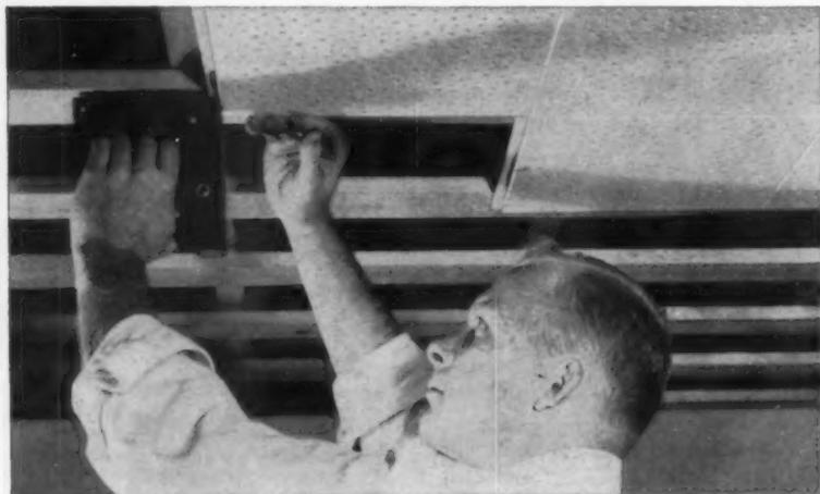
In one fast installation, Cushiontone provides modern Sound-Conditioning and a beautiful ceiling. Sturdy T & G joint speeds nailing, stapling, or cementing and insures a level ceiling.
