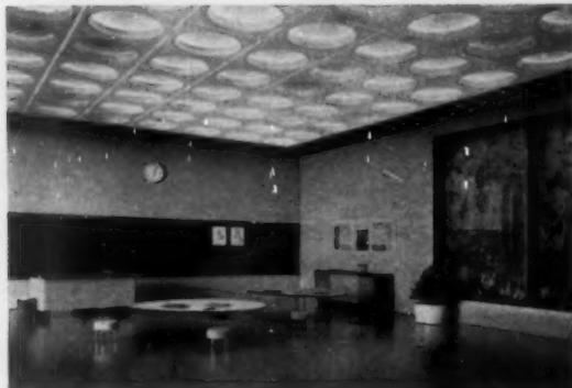
▲ **WALL-TO-WALL CEILING** of fluorescent lighting, "Sylva-Lume," is modular, interchangeable plastic panel system. Variety of panel patterns, colors, styles. Extruded aluminum track system, 3 ft.-square vinyl plastic diffusers, acoustic wedges or baffles. Sylvania Electric, Dept. AB, 1740 Broadway, New York 19, N.Y. (No. 5001, p. 132.)
