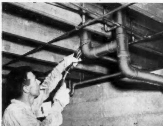
**Fast, dependable connections:** Solder joints are easy to make and they stay tight. The circular torch shown is a big time saver on a large job like this. (Water lines are also copper.)
