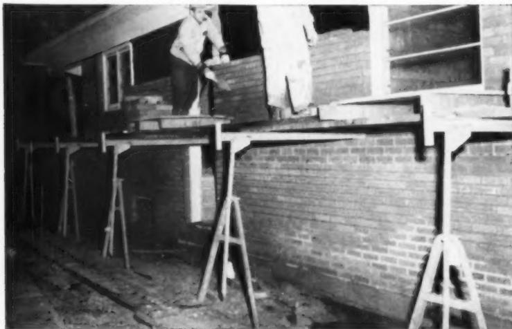
FOR FAST MASONRY CONSTRUCTION, mason contractor L. Hubbard of Euclid, Ohio, uses new "Trouble Saver" Putlog Trestles on a project for Joe Miller Homes Co. The new Putlog Trestles are 5'-long and provide nine height adjustments, ranging from 4' to 6'. Masons set each Putlog on the top course, then brick is laid over them. Putlogs are pulled out of the wall and adjusted to new height as the job progresses. When a pin is removed, the new Putlog Trestle swings down flat for easy storage or shipping.
