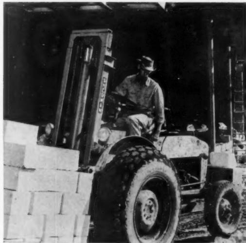
**75 BLOCKS** on one pallet with Sherman fork lift speeded Orlando, Fla., Colonial Shopping Center job by R. M. Thompson Co. Load went direct from delivery truck to mason's platform. **Circle No. 1006** on reply card, p. 134.
