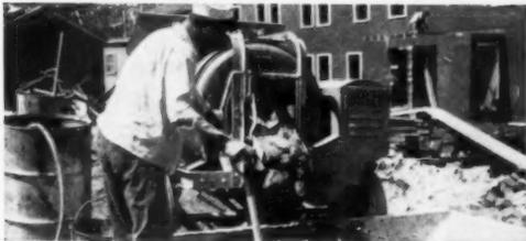
Get up to 15 extra yds. a day from the same labor with a Jaeger 3 1/2 S Auto-Loader, the fastest half-bag mixer built, because you load as you mix and measure as you load. Power-shaker action charges drum in a flash; extra big bucket and flight blades mix thoroughly, discharge rapidly.
