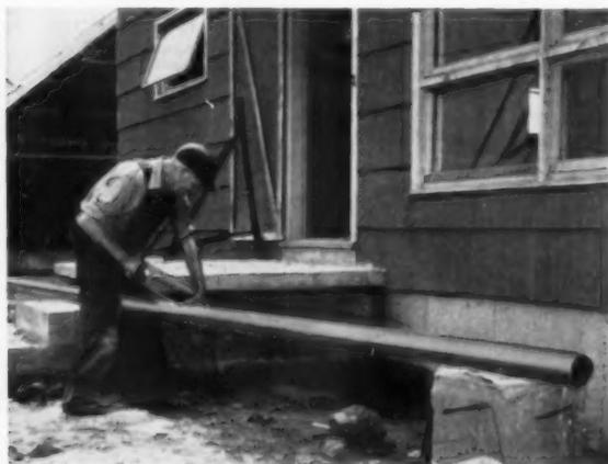
**Fewer joints and fittings:** Copper tube comes in standard 20' lengths. A 20' length of 3" Type M weighs only 53 pounds. Easy to cut, too.
