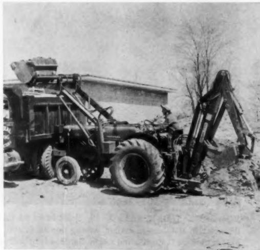
**COMBINATION** backhoe and loader by Ottawa is shown here on new International Harvester W-400, is also available for W-600, W-300. Common frame for both units is designed to cut strain on tractor frame. **Circle No. 10003.**
