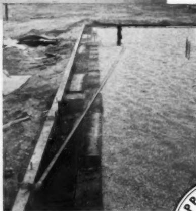
(Above) Here you see a 1½" Revere Copper Water Tube, Type "L" drainage line running from the kitchen sink before concrete slab was poured. Note how builder took advantage of the single, long, light, straight lengths of Revere Copper Water Tube . . . no extra joints, caulking or thread cutting here. In addition the builder had no fear of copper rusting when buried in the concrete slab. Revere Copper Water Tube also was used for service lines and internal water distribution.
