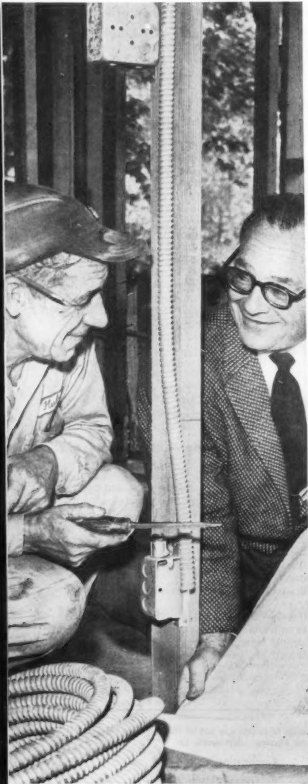
**PASADENA ELECTRICIAN** Harold Hubbard shows Pacific Electric's John Wynn how conduit is brought into outlet box for built-in telephone service. Wire is fed through conduit from outside.
