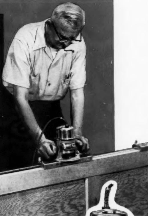
Here's the perfect answer to every contractor's or carpenter's routing needs! New SKIL Model 297 Router is lightweight, easy-handling, smooth-cutting...delivers more than enough power for routing out sink tops, grooving in shelves, dadoing, beading, rabbeting, mortising, veining, and cove cutting... handles a wide range of decorative
