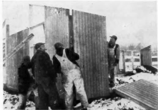
**COMPONENT SECTIONS** enable the builder to erect walls and roof quickly. Tricky work like measuring and cutting, hard in awkward mittens, is done in the shop.
