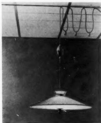
**TRAVELLING FIXTURE** by Lightolier. Shallow parasol shade fixture called "The Traveller" is suspended by a counter-weighted cord, glides across ceiling on slim brass track as far as 72". Fibreglas shade ribbed with walnut strips. About \$72. From Lightolier Inc., Attn. J. Levine, Dept. AB, 346 Claremont Ave., Jersey City, N.J. (No. 10034 on page 154).
