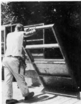
**WINDOW FRAME PANEL** is tilted into place. This one has one operating sash, one fixed pane, costs \$63.75.
