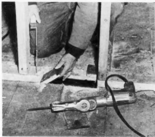
**FOUR MINUTES** to cut warm air duct opening (including 2x4 plate and direct cut into floor without starting hole) with B.C.S. Super Saw. Instant removal of saw from drill is made possible by a patented type of lug drive that provides a positive connection between the saw and the  $\frac{1}{4}$ " electric drill. **Circle No. 10009 on reply card.**
