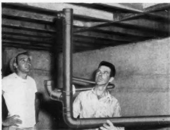
**Easier, faster handling:** The section, comprising about 13' of copper tube and 5 solder-joint fittings, weighs only 35 pounds, is handled by one man.
