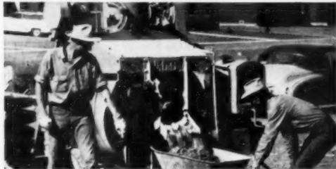
Pours 60 yds. a day with Jaeger 6S Speedline mixer. Mixer and 7 man crew (3 loading, 3 wheeling, 1 operating mixer) averaged a batch every 1 3/4 minutes pouring footers and floor slab. Famous "Skip Shaker" loader speeds batch into drum in 5 to 7 seconds. Discharge is just as fast. Criss-cross double mixing action assures uniform quality concrete.
