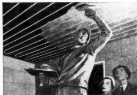
*Longer-lasting radiant heating installations are economical, quick and clean when made from Chase copper water tube. No worry about leaks or repairs—can't clog with rust!*
