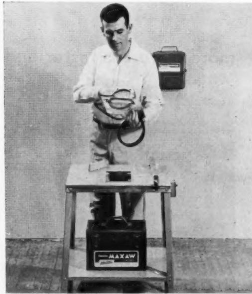
**LEFT OR RIGHT** hand saw table No. 777 by Maxaw for saw models 717, 737 or 747, permits all bevel, depth, miter and ripping adjustments. Saw is removed quickly. Capacity is 2 1/8" at 90° and 1 7/8" at 45°. The saw shoe fits flush with the table top, which is 24" wide, 20" deep; legs are 34" long. **Circle No. 10011 on reply card.**
