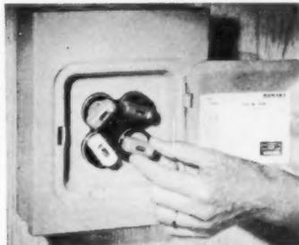
**TAKING RISK** out of replacing burned out fuses, especially in darkness, are these Sightmaster fuses, which have tiny built-in neon light that glows in dark. Fuses need not be removed; you simply turn them, dial-like, to next click. No need to worry about matching amperages. Fuses have six lives, are made in 15 to 30 amp sizes.
