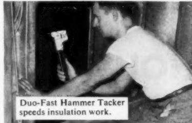
Duo-Fast Hammer Tacker speeds insulation work.
