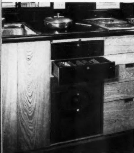
Black-topped counters and stainless hardware harmonize with the shiny black molded phenolic drawers, set off the finish of wood panels. And, they clean with the wipe of a damp cloth.
