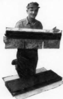
The exclusive Flintkote aluminum strip retards the action of the adhesive *until it is needed*. In addition, this aluminum strip keeps the shingles free in the bundle... they do not have to be broken apart on the job. A SEAL-TAB roof is quick and easy to apply, guarantees greater customer satisfaction.
