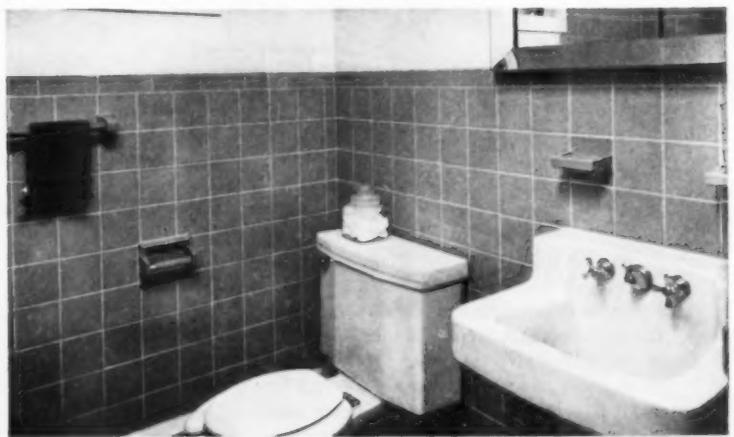
The adhesive method was used to apply ceramic tile to the bathroom walls and in the inviting shower enclosure. Alert use of progressive new techniques like prefabrication and adhesive installations help to sell homes at a fast—and profitable—rate.
