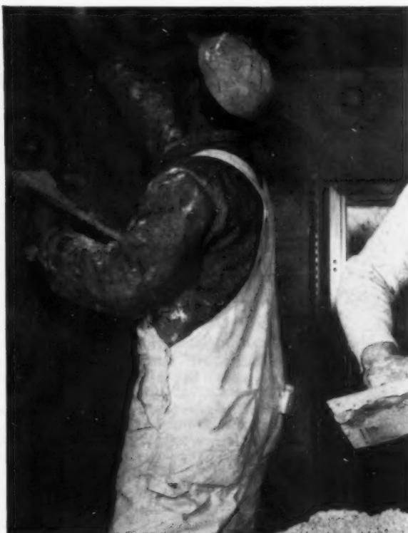
**QUALITY AND VALUE** are evident to prospective home owners when you feature plastered walls and ceilings. **RED TOP\* STRUCTO-LITE\*** perlite-gypsum basecoat plaster is mill-mixed, requires
