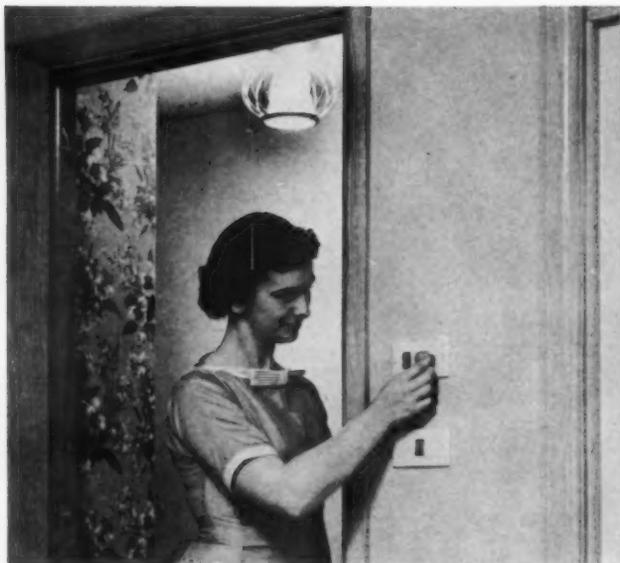
**G. E. LOW VOLTAGE REMOTE CONTROL** wiring system in Appleton, Wis., house has master selector switches in bedroom and kitchen for controlling all lights. System has 25-volt transformer, nine circuits.
