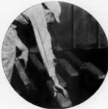
2. Lay short lengths of 2x4 on 12" centers. Lap joints.
