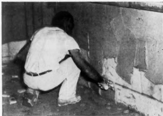
**4** **PLASTER** keys directly to Styrofoam without lathing!
