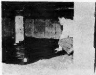
**New vapor barrier for floor waterproofing**
