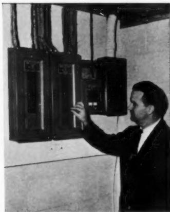
**BUILDER DARREL HOLCOMB** shows circuitry in his 100 amp service panel: 18 general circuits, 6 special appliance, 2 water heater, 4 spares.
