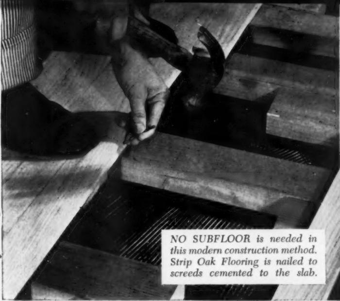
**NO SUBFLOOR** is needed in this modern construction method. Strip Oak Flooring is nailed to screeds cemented to the slab.
