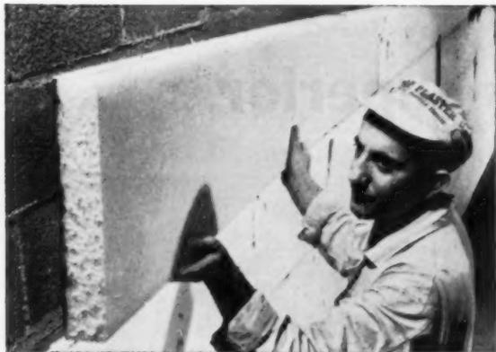
**3** **STYROFOAM** adheres readily to masonry without furring!
