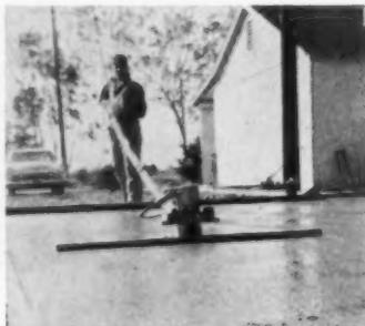
This builder converted a hand bullfloat into a power model by mounting an oscillating sander on top of the float. The resulting machine, he claims, runs down the aggregate and works up the "fat" much faster than if it were used without the vibration. The electric cord for the sander is run up the handle to keep it out of the way.
