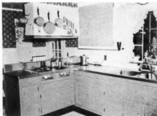
NEW JERSEY. Mr. Morehouse's Short Hills kitchen has Caloric built-in burners for main cooking, with new controls and hypodermic pilots; Roper griddle; Gaffer & Sattler grease collecting pot with full-up signal light.
