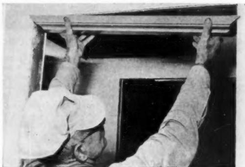
**1 ADJUSTABLE** door jamb and trim is redwood. Here, workman is placing the head but does not nail it in place. Head is screwed in place later.
