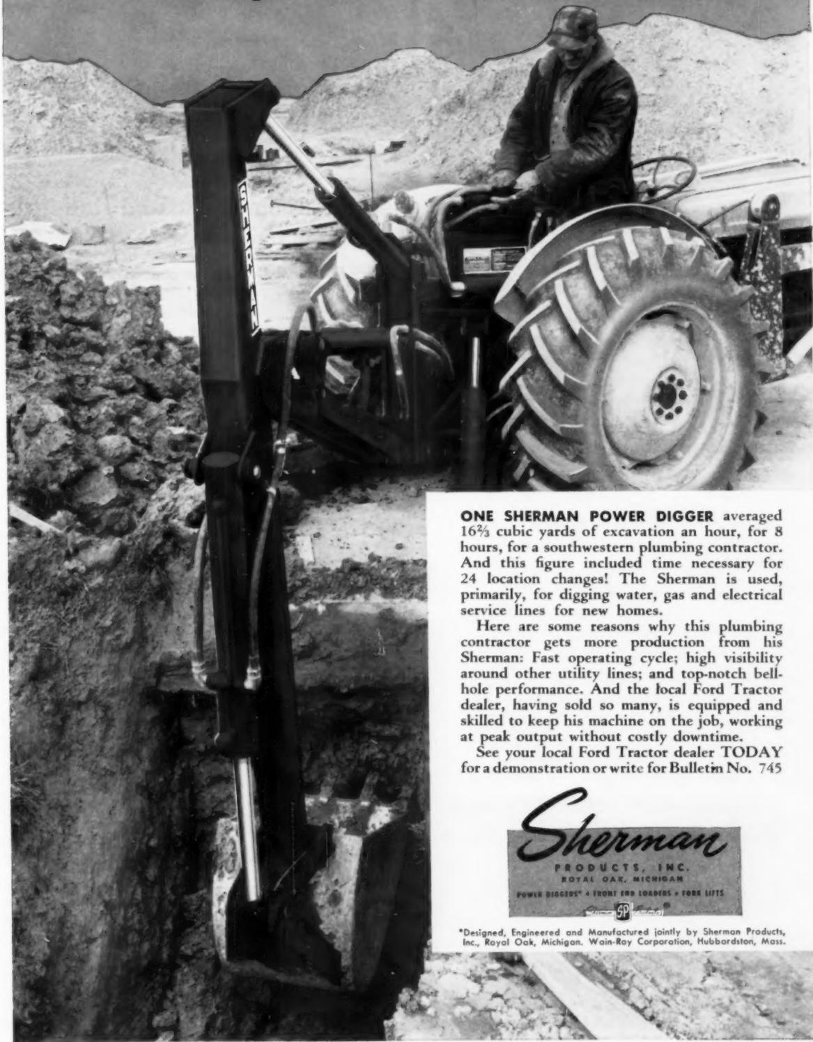
**ONE SHERMAN POWER DIGGER** averaged  $16\frac{2}{3}$  cubic yards of excavation an hour, for 8 hours, for a southwestern plumbing contractor. And this figure included time necessary for 24 location changes! The Sherman is used, primarily, for digging water, gas and electrical service lines for new homes.
