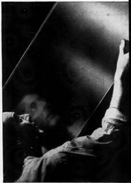
**BUILD, INSULATE, CONTROL MOISTURE** in one low-cost operation with Insulating ROCKLATH\* plaster base, applied to outside walls and top floor ceilings. Aluminum foil backing provides a superior vapor barrier, protects framing from damaging moisture condensation. Properly installed, it reflects 95% of sun-generated heat rays, keeping rooms up to 15° cooler—an important sales feature.
