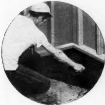
1. Spread mastic over surface of waterproofed slab.
