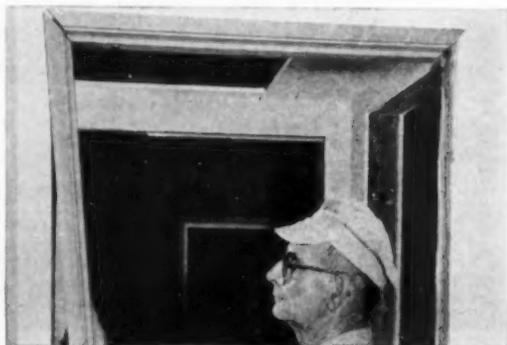
**3 PLUMB AND SET** hinge side. Use shims under hinges. Plumb and set opposite side. Apply shims here too if necessary. Pull head down and fix.
