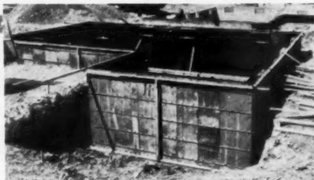
This photograph shows foundation forming with Gates Horizontal Rod Forming System. Gates Horizontal Rod Panels are versatile, lightweight and reusable. Waling is held to a minimum, and erection and stripping time is reduced, to show substantial savings and profit on every job.
