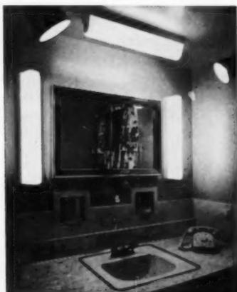
**THREE FLUORESCENT FIXTURES** at shaving mirror easily give more than 40-footcandle minimum required. Note two sun lamps.
