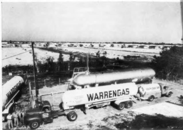
**STORAGE TANK** with 30,000 gal. of LP gas is being filled by large Warren supply truck. Smaller truck taking on gas will service outlying developments. Subdivision's sewage plant and water tower are inside the same fence enclosure.
