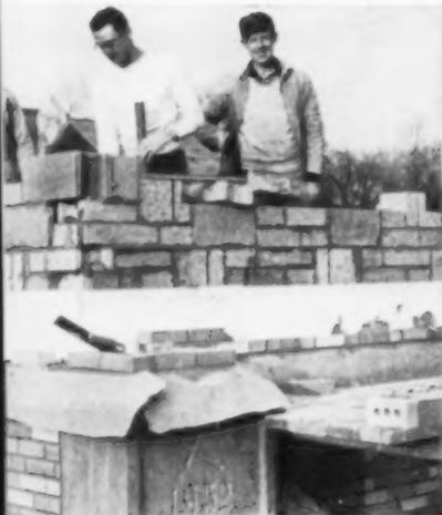
**CAVITY WALLS** may be constructed with air space on either side of Styrofoam.
