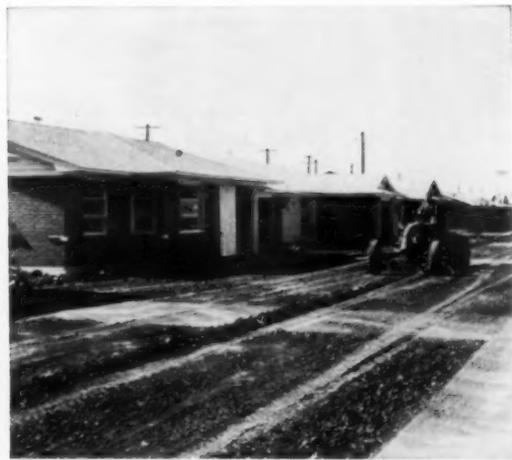
**20** FINAL YARD GRADING is done by a small Allis-Chalmers "maintaining" machine. Several houses are finished at once in large developments like this, but such a machine saves money on a single job as well.
