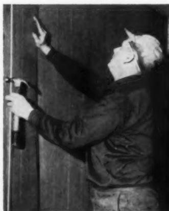
**4 FITTING** the piece into place. There can be no second guesses, for the cement grabs. Or place a paper buffer between panel and wall; slide it out after the panel is aligned. Then panel is pressed to the wall.
