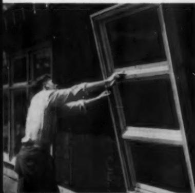
Ventilating sash of Flexivents opens wide to supply complete ventilation all through the home. Can be left open during rains without fear of damage to interior.
