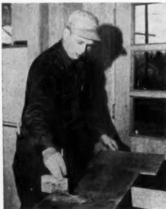
**2 COATING** the back of the piece with contact cement. Before this, the cut edge was planed and back-cut slightly to make a better butt joint. Various plywood manufacturers give instructions on use of own cements.
