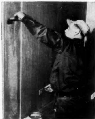
**3 COATING WALL.** Each panel must be fitted and prepared separately for application at right degree of tackiness. The wall surface must be clean, bare and flat so adhesive will not pull away. Furr out plaster walls.
