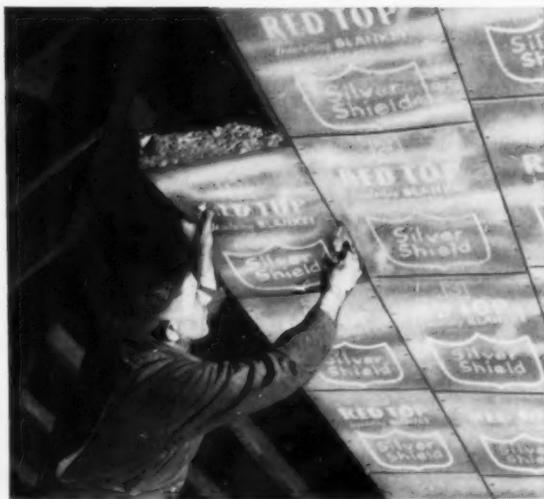
**YOUR REPUTATION FOR QUALITY HOMES** will be thoroughly protected when you provide added comfort with USG Insulating Sheathing. It insulates more than twice as effectively as nominal one-inch wood sheathing; "k" value is 0.33. Sheds water, repels wind, weather. Light-weight, yet so strong that FHA requires no corner bracing when the 25/32", 4-ft. width board is used. Saws on studs, saves valuable time.
