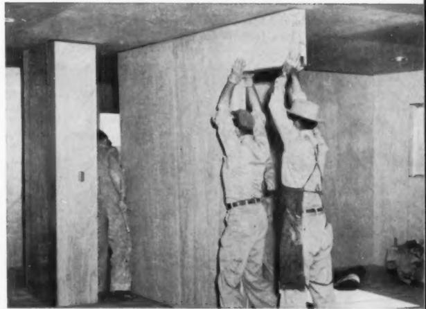
**5** **BEDROOM WALL** section is moved into place by 3 men. Built-in sliding door is already in place, complete with all hardware. Shop-built components such as these make better product possible at lower cost.
