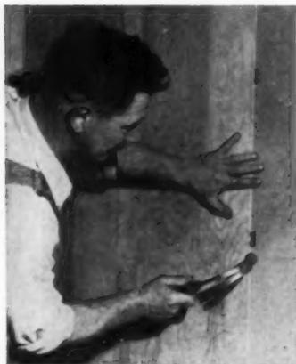
**7 CLIPS,** developed by various manufacturers for specially grooved panels, hold panels to wall and join them together. Clips are held by nails, which must go through drywall, as in photo, to studs or furring.
