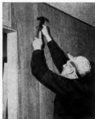
**6 NAILING** with 4d finishing nails to plate and sill and along the stud to reinforce the cement bond. Nail holes are countersunk and filled with matching putty. In unfinished panels, fill holes after applying first coat.
