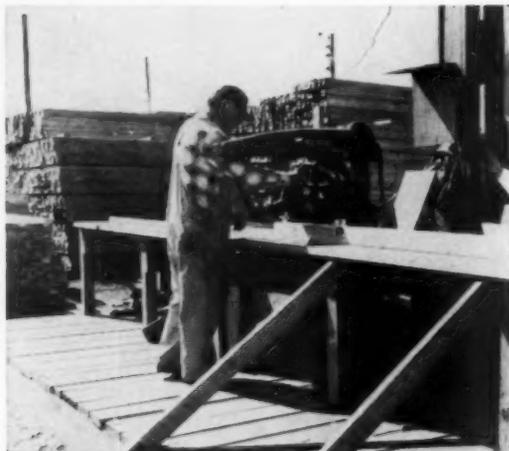
**10** **RADIAL SAW** is workhorse of precutting operation. It can cut large numbers of studs and rafters at a time, makes angle cuts and birds' mouths. With it, in effect, a shop cutting table comes to the site.
