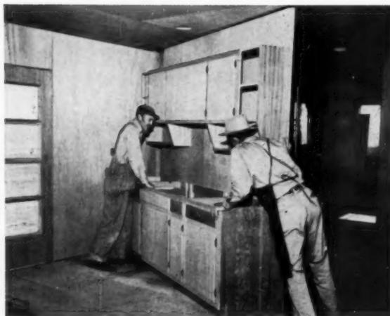
**3** **COMPLETE KITCHEN WALL** section is shoved into place on Bates job by two workmen. Philippine mahogany cabinets and wall surfaces have furniture-like finish. The entire unit takes only a few minutes to install.
