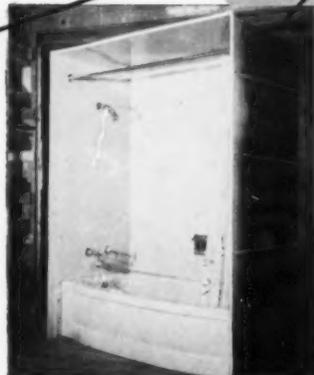
**TUB-SHOWER** and wall section of pressed steel comes as one unit, eliminates costly on-the-job labor.
