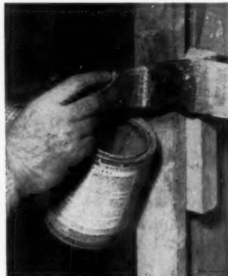
**3 APPLYING ADHESIVE.** A better bond is achieved if one coat of cement is applied to the strips and allowed to dry, and then another coat is applied. Without adhesive, the panel may bow and make the nails pop.
