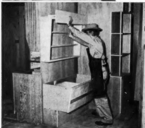
**2** **BATHROOM VANITY** wall section goes into place easily, reduces need for skilled labor in building separate parts on job. Tutt Cooper predicts greater future use of built-in furniture in houses also.
