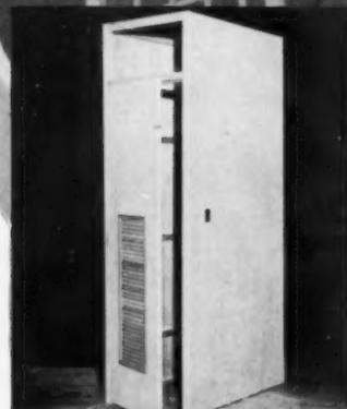
**HEATER CLOSET** has louvered door, is planned to accommodate compact systems designed for small homes.
