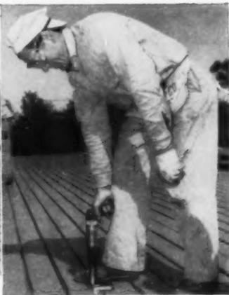
J. S. Stephens and Sons, Tampa, Florida contractors, used DRIVE-IT tools to speed the installation of the steel decking used as the roof of the Dunedin Shopping Center. Mr. Stephens used two model 330 DRIVE-IT tools to drive over 4,000 drivepins to anchor the steel decking to the steel roof trusses. Installations of this type average about 75% savings over drilling and other outmoded fastening methods. If you fasten *anything* to concrete or steel—you can save with DRIVE-IT tools.
