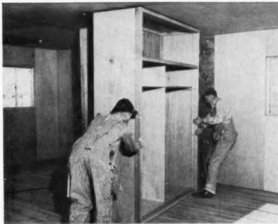
**4** **WARDROBE COMPONENT** also acts as room divider, is set into place after finished floor is laid. Workmanship on unit is far more polished than is possible with small town local labor. Costs also are less.
