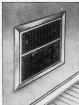
**Simple but decorative trim frame adds a final touch.** Notice that this  $16\frac{1}{2}$ " unit does not project into the room. It's practically flush with the wall.
