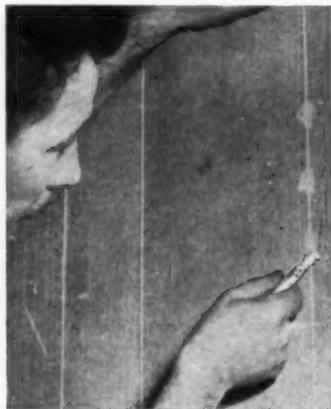
**8 PUTTYING.** Prefinished panels come with putty sticks of the right color for filling nail holes. In unfinished paneling, nails should be set and holes filled after applying first coat, usually primer or sealer.
