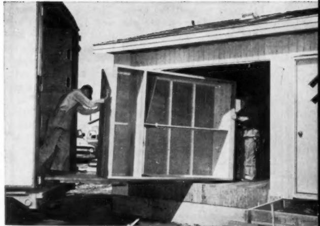
**1** **SIX FOOT** storage wall section is moved into Pan-Ama house in Amarillo through front picture window opening. Firm builds in small towns, usually constructs less than 40 houses in a group.
