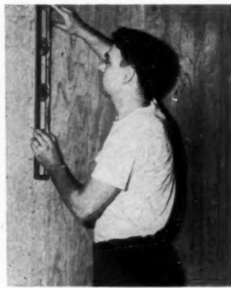
**9 A WARNING:** keep checking for plumb. Shim out furring strips or fill hollows of walls. Keep a level on deck for true up-and-down. Molding will take care of irregular meeting with floor and ceiling.
