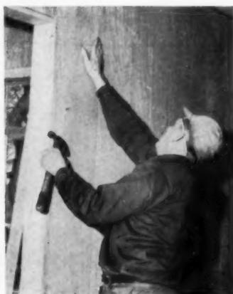
**5 PRESSING** the whole piece to the wall. Here the random grooved plank effect offers some relief from need for perfect butting or matching of grain of adjacent panels. Grooves are spaced to occur at 16" intervals.
