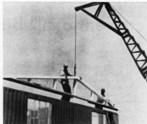
**CRANE**, standard equipment on H.B.C. trucks, speeds truss placement, permits use of utility core and . . .
