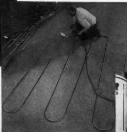
**ONE OF THE MANY DESIRABLE FEATURES** of enduring Revere Copper Water Tube is that it can be prefabricated in the shop, requires fewer fittings, which when properly brazed or soldered assure tight, non-leaking joints. Completed, prefabricated panels are then shipped to the job and installed, using separate circuits for each room.
