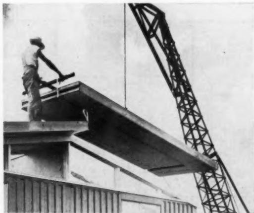
. . . large roof panels, which are positioned by H-bar and steel straps fastened to sections at factory.
