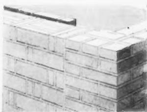
**DETAIL OF HOW** Rancho Ventura brick walls were laid. Note resemblance to standard Flemish bond. **TWO-TEXTURED BRICK** house has 1,518 square feet of livable area and two ceramic-tiled bathrooms.
