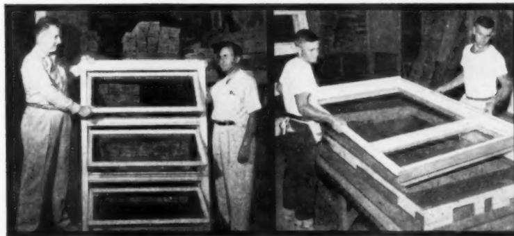
Robert Cutts (left) and Carl E. Swartz demonstrate 3 high Flexivents stack specially designed to fit perfectly in Lu-Re-Co panel system of construction.
