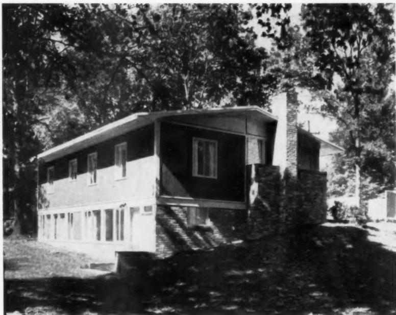
**FRONT AND SIDE** elevations of National Homes' Hollybrook model, by architect Charles Goodman, were left "as is" by builders of this part-prefab, part-custom built house. Photo directly above shows lower level that was added to package and built "conventionally."
