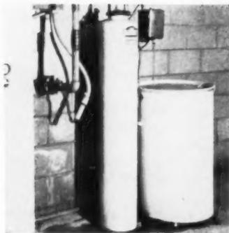
There are two recommended systems for installing a water softener. System A provides complete softening of both hot and cold water at all outlets. The only exception is hard water for lawn sprinklers which by-passes the main incoming line before it enters the softener. System B softens both hot and cold water, with the exception of water for toilet flush tanks and outside lawn sprinklers.
