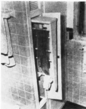
**BUILT-IN** lingerie dryer has heating duct at floor level. Warm air circulates around clothing and out at register provided at top. Racks slide out.
