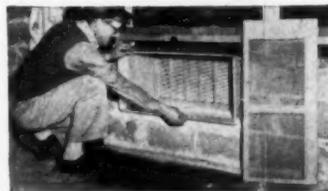
**NO DUCTS! NO PLUMBING!** Install the shell anywhere in any outside wall, slide in cooling unit.
