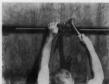
By tapping the lever, forms are locked into place. A minimum of bracing is required
