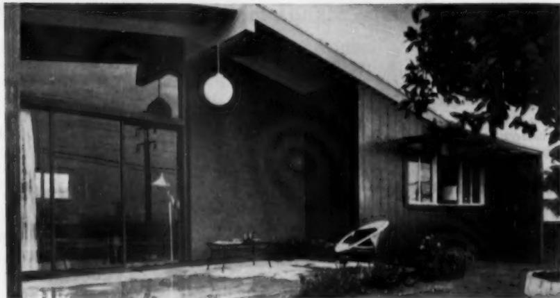
**4-FOOT ROOF OVERHANG** shields glass area and terrace. House is built of concrete block with plank-and-beam roof construction. It cost \$16,500 in Las Vegas, Nevada
