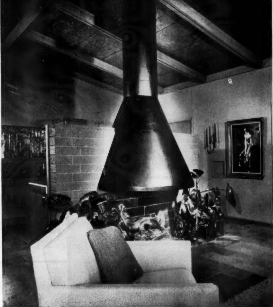
**CONVERTIBLE FIREPLACE** has a sunken hearth that is used as a goldfish pool in summer. Metal hood and 24-inch pipe are supported by 5-foot-high wall separating living and kitchen areas. Water in pool is recirculated by pump
