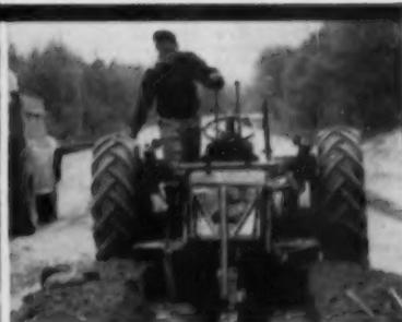
**LOWER TRENCHING COSTS**—Ford Tractor and trencher digs up to 800 lineal ft. per hour. Widely used for gas and water lines, sewer systems and electrical conduits.
