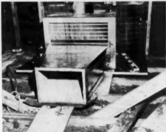
First section of return air duct attached to unit. Duct material is of 3/4-inch sheets of Fiberglas shipped flat-sized and scored for use. It can be cut with a saw or heavy knife
