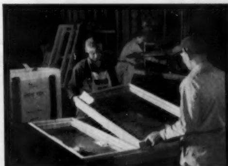
Extreme ease of assembly is readily apparent as workmen slip Flexivent Window Units into place in Lu-Re-Co panel jig at shop of Northern Indiana Lumber & Coal Co.
