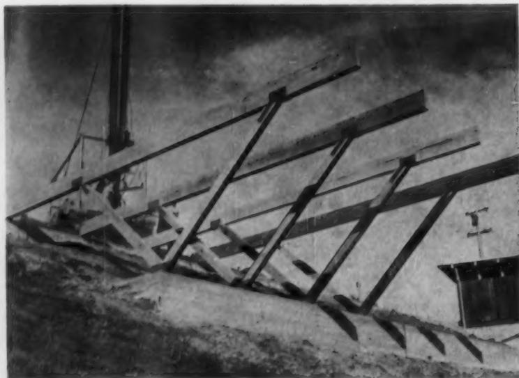
Trusses with 4x12 beams, 4x6 struts, are placed by gin pole (rear)
