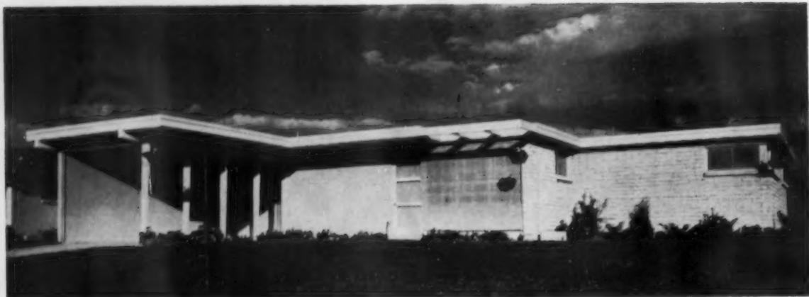
Wide overhang of carport shields walk to main entrance. When converted to garage, obscure glass lights are installed between upper part of 3x10-inch tapered posts
