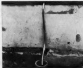
Copper tubing from the integrated unit carries off the condensate to drain tile outside the house. Provision for draining can be varied to suit the structure
