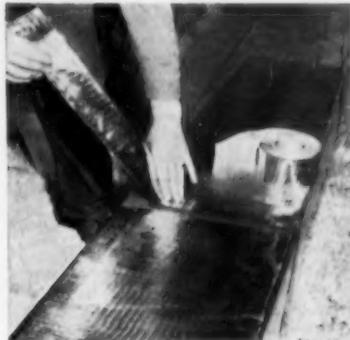
After cement is properly spread on duct work, the foil-faced reinforced fiber tape is applied around joints
