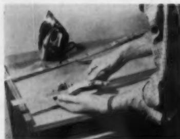
Woodtape's protective paper backing is removed and the material cut to length with a pair of scissors
