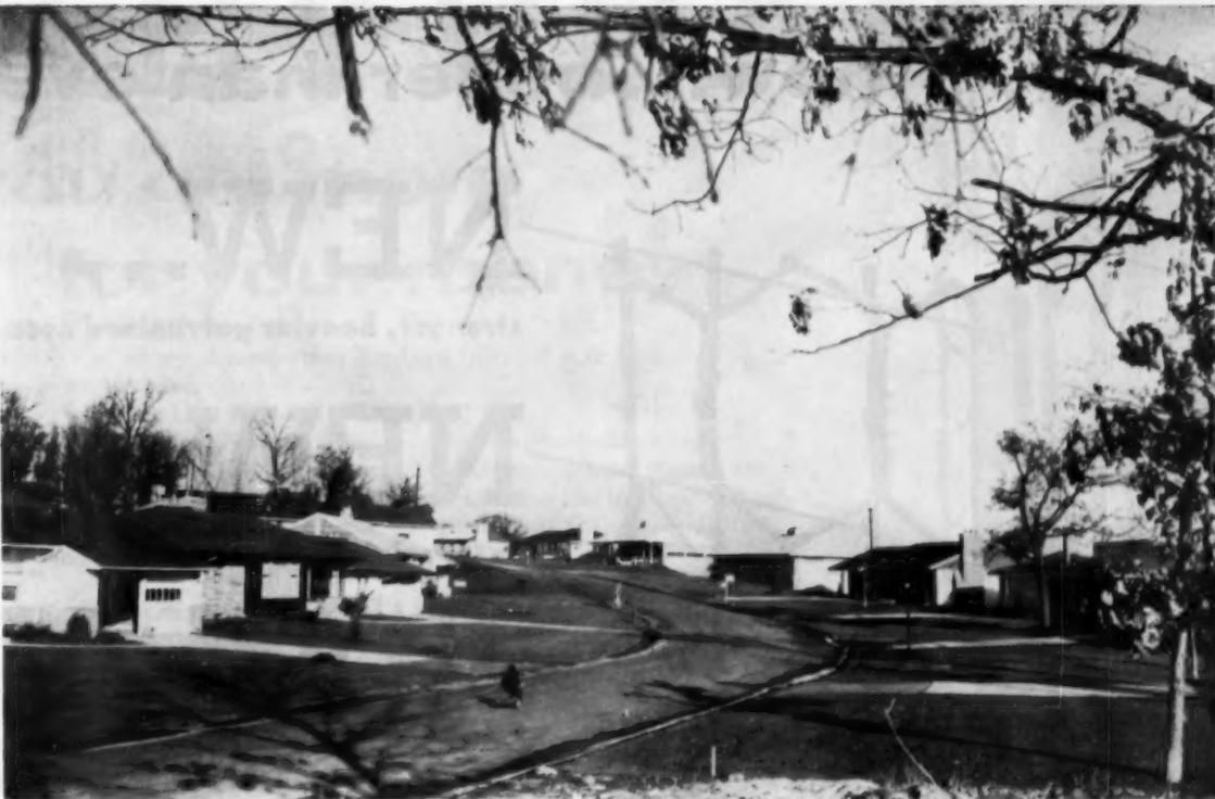
This is a good example of contour planning—the street pattern being made to fit the existing topography
