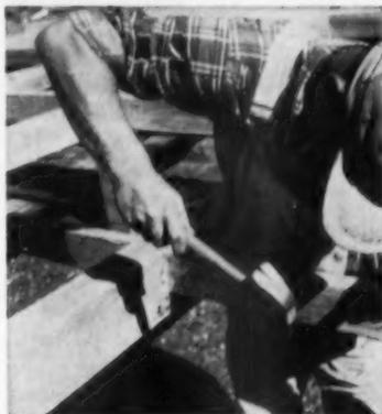
BETWEEN JOISTS is a 2x4 nailer, also on 4-foot centers . . . Nailers are positioned with Teco framing clips for strength and speed of installation
