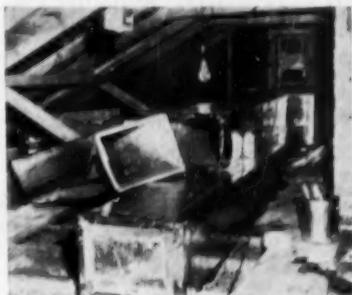
Return air duct completed. In this case it opens into center hallway for return air supply. Cold air duct is here shown in process of assembly. Cold air duct is 10x14 inches (inside measurements)
