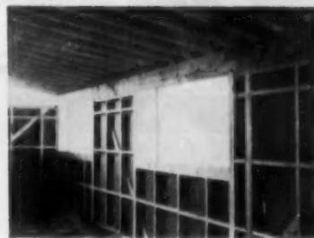
Interior view of wall at left shows the insulated sheathing. Note diagonal bracing for stability
