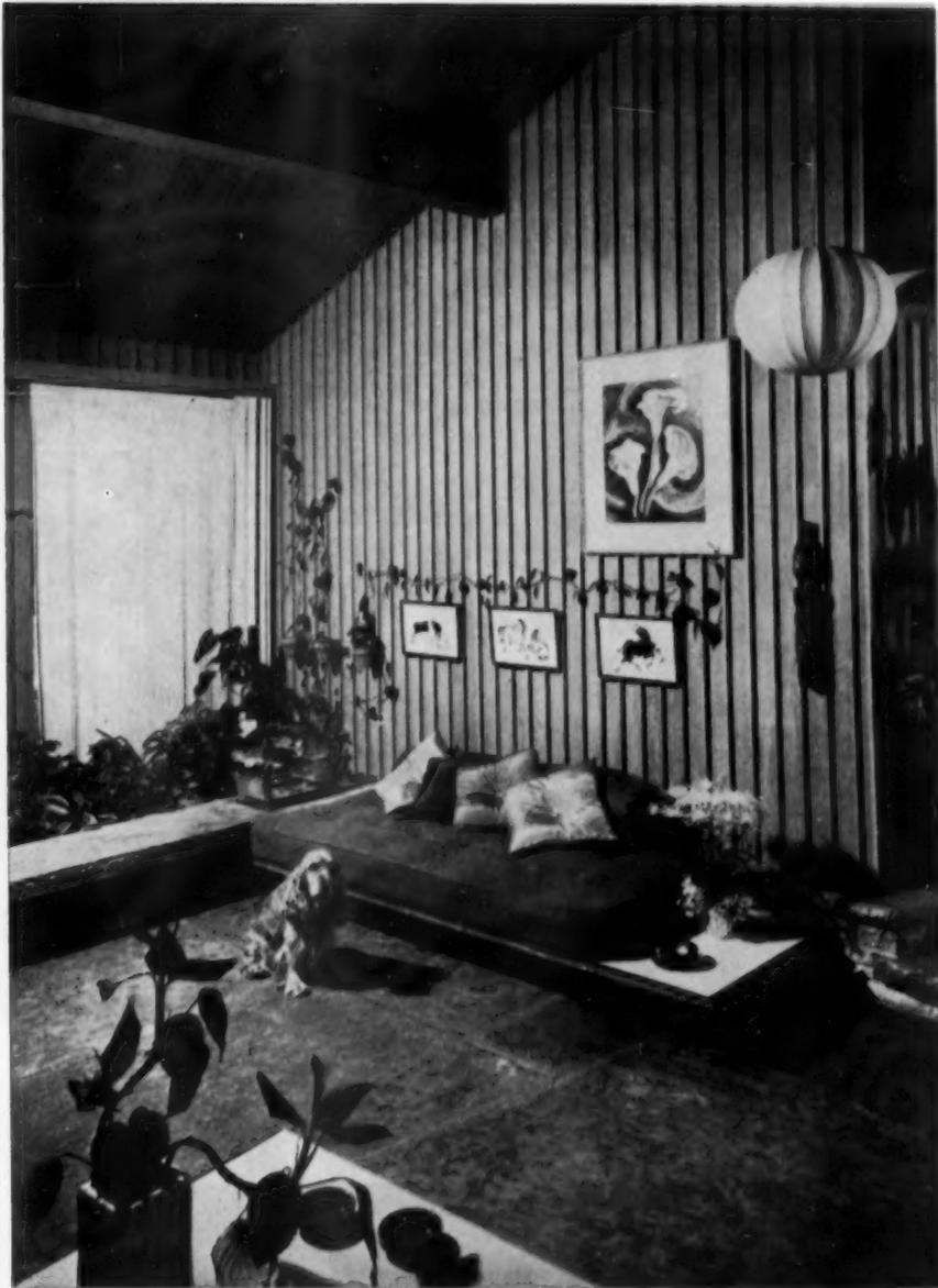
**DRAMATIC PATTERNED WALL** is achieved by nailing vertical  $\frac{3}{4}$ -inch by  $\frac{3}{4}$ -inch battens over the plywood
