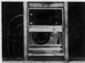
This integrated unit measures 14 $\frac{3}{4}$  by 17 by 4 $\frac{3}{4}$  inches and can be installed between standard stud spacings. Here the unit is installed over a basement. All piping may be concealed in the floor and walls
