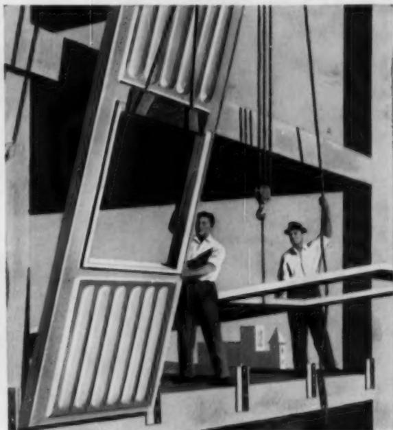
**6. WALL PANELS** prefabricated with Kaiser Aluminum are light in weight, easy to handle, economical to erect. Can be fabricated in various handsome exterior designs. Narrower wall section may be used—increasing interior floor area.
