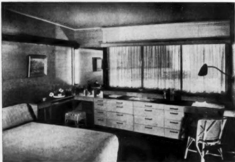
**HORIZONTAL SCORED PLYWOOD** is used on this bedroom wall. The scoring is another way to hide the seams, also gives the room illusion of greater width
