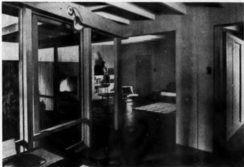
**HALF-ROUND BATTENS OVER PLYWOOD PANELS** on two-foot centers. Battens hide the seam of the butt edges of the plywood
