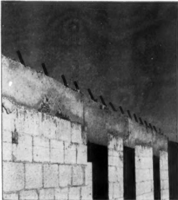
These effectively hold down prefabricated roof trusses. Design will resist hurricane winds
