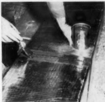
The two pieces of duct work are then joined. Cement is applied to the joints with an ordinary brush
