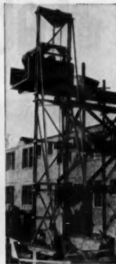
**Cut placing costs**—Jaeger Self-raising "Hoister" Tower makes quick work of material placing, saves labor. Assembles easily in 10' sections to 67'. 1-ton capacity. Available with material cage or 14' bucket. Easy to move. Positive automatic safety device.
