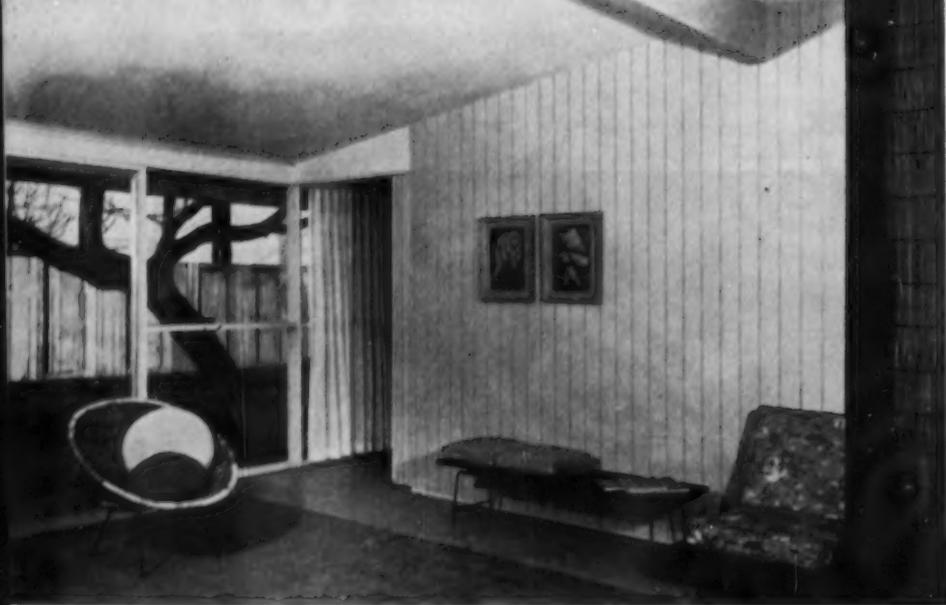
**VERTICAL PANELING** in this living room wall is large sheet Texture 1-11. This material is quickly installed, gives a pleasing effect and avoids seam problems
