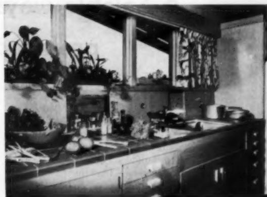
**STORAGE CABINETS** with sliding doors of plywood are tucked into the area between counter top and window. They provide handy storage for wide variety of kitchen items, are attractive in appearance, easy to use
