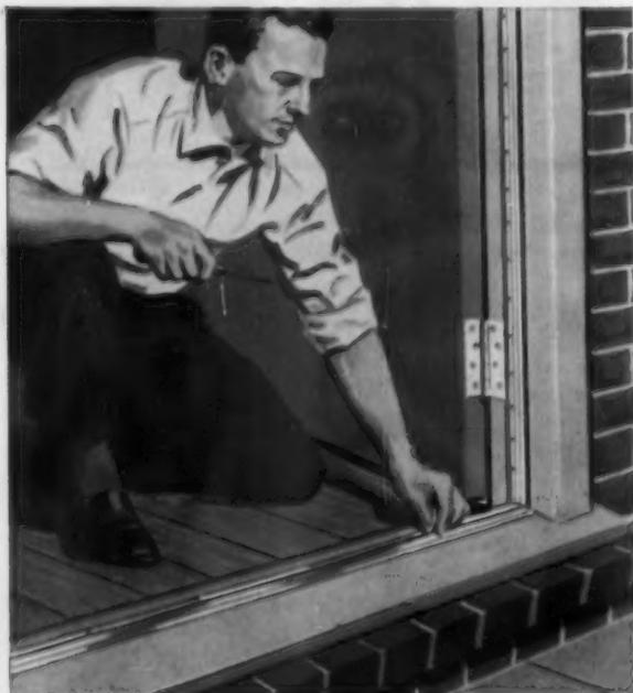
**3. WEATHERSTRIPPING** and thresholds made with Kaiser Aluminum give more economical protection against dirt, dust, weather. Non-corrosive, and won't rust. Aluminum weatherstripping retains spring tension after years of continuous use.
