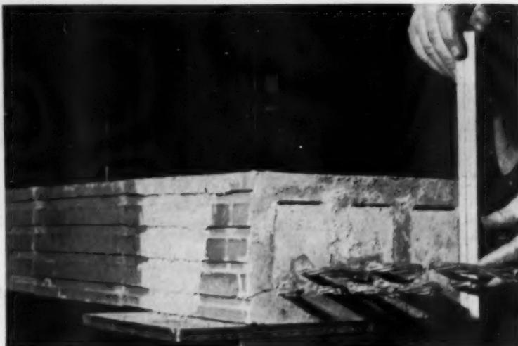
**PRESTRESSED GIRDER** is made of hollow clay tile units butted together. Strand wire is tensioned in cells of the tile, by use of a hydraulic jack. Grout holds the steel in tension. The steel strands are of 1 1/4-inch diameter and 3/8-inch diameter. Tile is 12 by 12 by 6-inch
