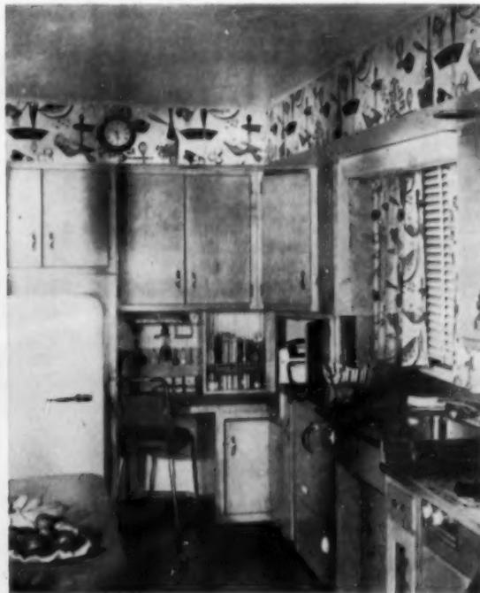
**GROUP WORKING UNITS LOGICALLY** in relation to one another. This food preparation counter (at 30 inches) is flanked on one side by the refrigerator, on the other by revolving corner cabinets and mixer. Facing is handy midway cabinet and pegboard. Note that the range unit (extreme right) is built to the 33-in. height best suited for ease of working with all types of utensils.
