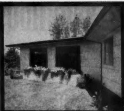
**PLYALOY OVERLAID PLYWOOD** provides the finest and most durable paint base of any siding on the market today. It takes paint easily, evenly. Eliminates grain raise and checking. The smooth, durable overlay is a medium-density resin-impregnated fiber permanently fused to Exterior fir plywood in modern hot-plate presses. Pre-cut to standard 12", 16" and 24" widths; 8' long; lower edge beveled for drip. Comes packaged by the square, complete with wedges and shadow-line furring strips.
