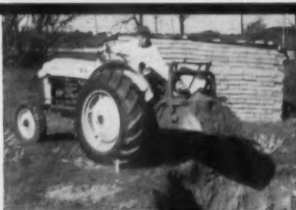
**LOW-COST EARTHMOVING**—Ford Tractor and reversible scoop save money on small yardage jobs. Useful for carrying bricks, sand and concrete blocks. Lifts and lowers hydraulically.
