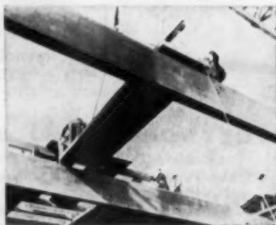
**CLAY TILE DECKING** of 5x20-foot prestressed slabs has four tiles side by side with a 4-inch space between. In the void was placed 3/8-inch steel strands for prestressing. The void was then grouted. Crane lifts decking into place. Strand ends protruding from end of decking key the grout that is poured between decking members
