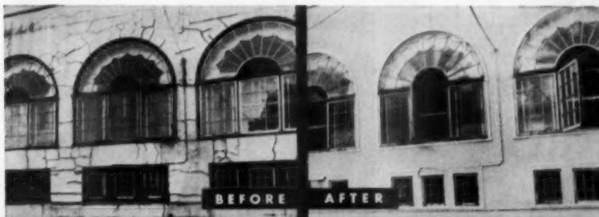
SPRAYED ASBESTOS RESURFACER
