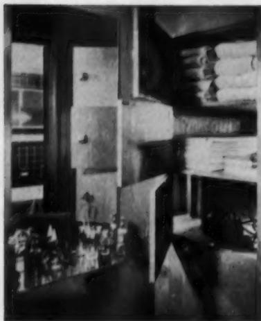
**PASS-THROUGH CLOSET** connects laundry and bathroom. Handy doors make it easy to feed towels and linen through. Three-way telephone has 20 foot cord
