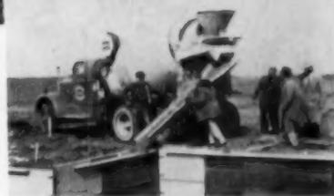
Gates Engineering Department designed one set of Horizontal Rod Panel Forms that could be used for all four plan variations in this development. They were manufactured of plastic-surfaced plywood in 32" widths—for maximum speed in erection and stripping. Delivered to the job at noon one day, the forms were set up, ready for pour, by 9:30 the next morning.
