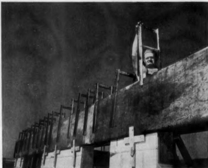
**REUSABLE 3/4-INCH FIR PLYWOOD FORMS AND OVER-SIZED CLAMPS** are cutting 12 per cent on materials and 20 per cent on labor cost in building reinforced concrete tie beams
