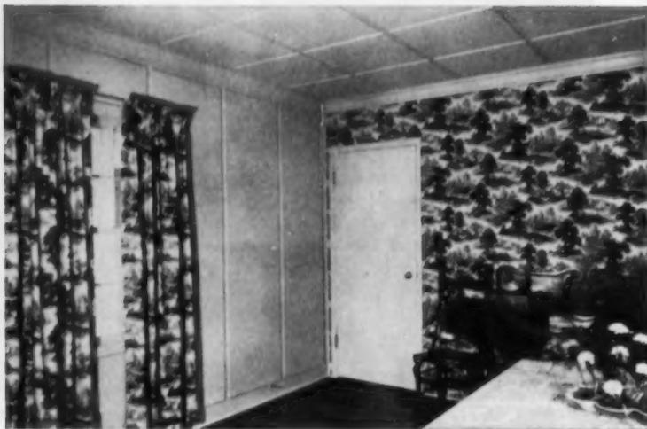
**PLYWOOD SQUARES** are applied here over plywood stripping. The result is "something different," and also avoids edge seams
