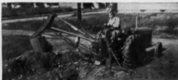
Another Oliver handy for trenching is the multi-purpose Super 55. Built-in hydraulics on this tractor operate a variety of front-, side- and rear-mounted equipment. The Super 55 is available with gas or diesel engine.
