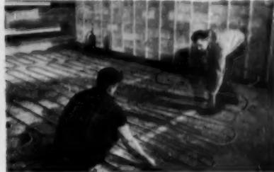
**HEAT FOR THIS** basement game room will be provided by 1/2" PG's embedded in concrete. For floor or ceiling installations the pre-formed Anaconda Panel Grid offers many economies.
