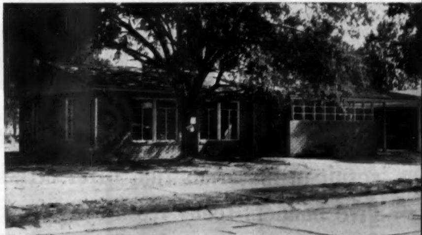
Brick veneer all over is combined here with a trellis-brick screen to give character to facade
