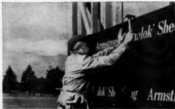
**Has high nail holding power** To pull a piece of Temlok Sheathing sideways from a nail driven  $\frac{1}{2}$ " in from the edge takes a force of 187 pounds. Most other insulating sheathings give way at about 120 pounds. This extra strength is one of the big reasons for the growing popularity of Armstrong Temlok Sheathing with builders.
