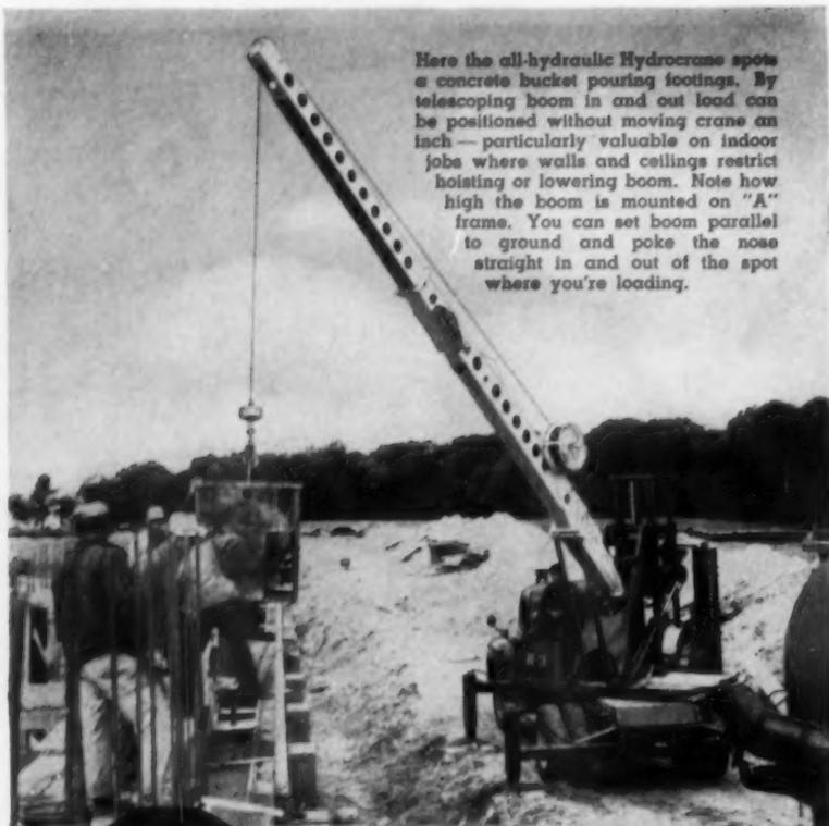
Here the all-hydraulic Hydrocrane spots a concrete bucket pouring footings. By telescoping boom in and out load can be positioned without moving crane an inch—particularly valuable on indoor jobs where walls and ceilings restrict hoisting or lowering boom. Note how high the boom is mounted on "A" frame. You can set boom parallel to ground and poke the nose straight in and out of the spot where you're loading.
