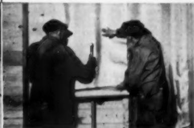
Using Sisalation to insulate walls. "Row-in" between studs allows maximum reflectivity.
