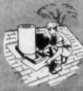
Assemble leak-proof flashing on roof at base of flue. Install housing around completed flue.
