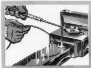
**It can be soldered . . . with ease and economy—**Long-lasting, water-tight joints are assured when standard soldering techniques are applied to Chase Copper Roofing Products.
