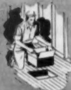
Place chimney support in prepared opening and nail iron supporting straps to floor joists.
