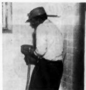
Holes are drilled in ceramic tile wall with an electric drill making 450 r.p.m. with a carboly-tipped bit
