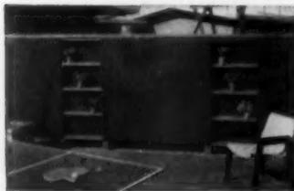
Equally effective for patio fences, gable ends and soffits, T 1-11 contrasts well with masonry and other materials.
