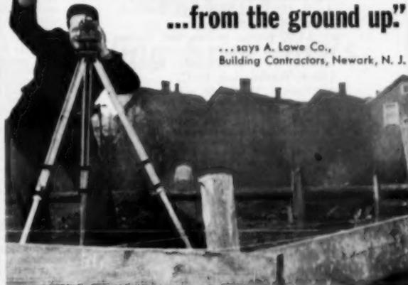
"One day you'll see it at work laying out a new factory site, marking batter boards, checking elevations for excavating and grading. Or it's measuring elevation of concrete piers for the steel columns of an office building, setting lintels, aligning and plumbing structural steel. On another job, we'll have it picking up elevations for finished floors, measuring hung ceiling heights, setting door bucks, and checking all other stages of construction."
