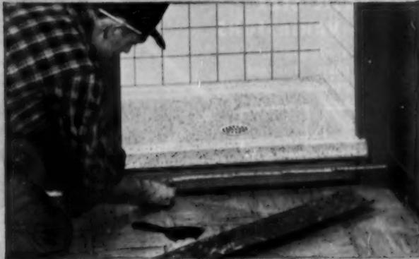
**3** The modern Precast floor provides perfect drainage permanently. Not fastened to framing or bonded to floor, the FIAT floor is never damaged by building settlement. Shower walls are finished over tiling-in flange to complete an economical, attractive and absolutely leakproof shower.
