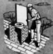
Cut housing panels to desired pitch and slide them together to form locked housing.
