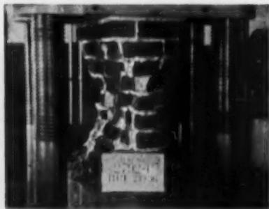
The strength of Brixment mortar is more than adequate for any type of brickwork. The strength of
