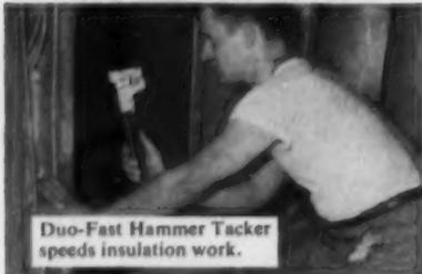
Duo-Fast Hammer Tacker speeds insulation work.
