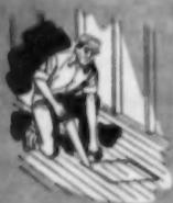
Prepare opening in floor, ceiling and roof. No clearance to wood members necessary.
