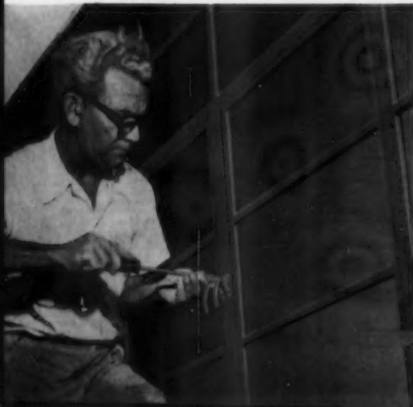
Mr. Joseph Fay, ornamental steel worker, shown as he secures the window lock on a double frame steel casement window.
