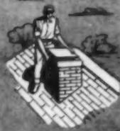
Set "Deluxe Housing Cap" assembly over housing to complete Van-Packer chimney installation.
