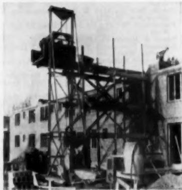
**Save hours of placing time**—Jaeger Self-Raising "Hoister" Tower places materials faster, safer, for less. Goes to job on truck or transporter. Readily assembles on the ground. 17-hp hoist raises it to 37 ft. Extensions to 67 ft. can easily be added. Hoists 1-ton loads. Material platform interchangeable with  $\frac{1}{2}$ -yd. concrete bucket. Positive automatic safety device.
