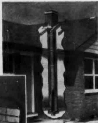
**ALL PARTS PACKAGED.** All materials for complete installation are provided in the packages — even flashing and acid-proof, leak-proof joint cement.
