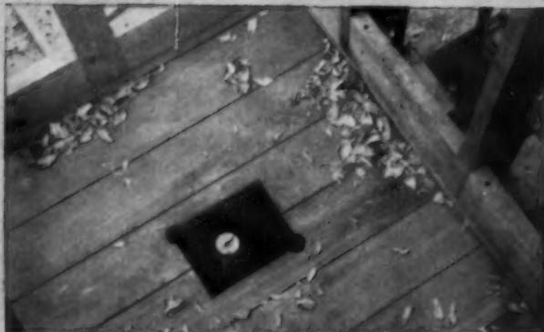
**1** No special construction or added support needed. Sub-floor is laid in regular manner, cutting small hole for drain connection. No need for lead pan, sub-layers, mortar etc. Savings of on-the-job labor makes installed cost substantially less than built-up floors.
