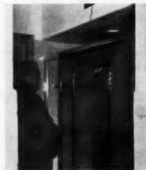
Final check is made on sliding doors. Top rail member holds doors and is supported by the two jamb members
