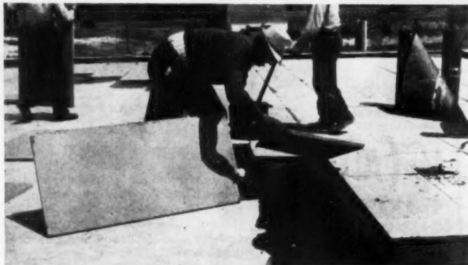
If mechanics are unable to complete the application of insulation board in a fixed working period, they then seal off the end of incompleated portions with strips of roofing felt. This serves as a water-stop and protects the installation against possible damage by a sudden rainfall
