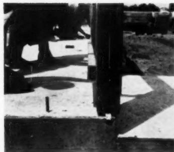
Showing the relationship of the wood framing to masonry foundation and floor; also use of strip mastic seal in between
