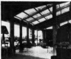
Resolite is a rugged structural sheet of Fibreglas-reinforced resin plastic, flat or corrugated for added structural strength. The material is unaffected by weather extremes of heat, cold or moisture. It will not rust, oxidize, mildew or rot. It is simple to apply with screws or nails and with ordinary tools and skill; it is easily adapted to roof, wall or partition.
