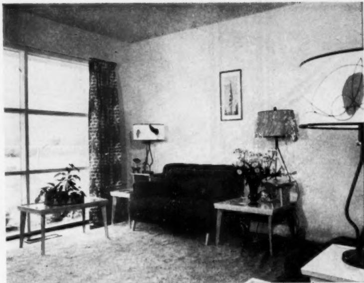
Vertical and horizontal grouping of single sash unit makes up the picture window, which extends to floor of the living room
