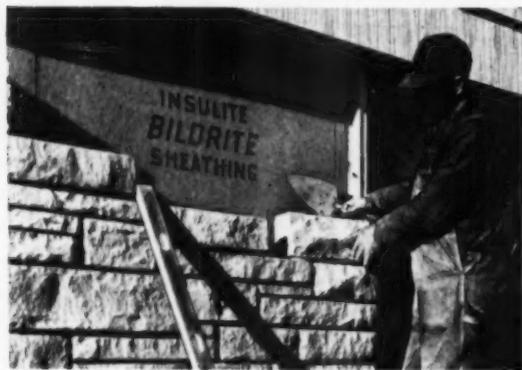
**2. Eliminates building paper.** Since Bildrite is waterproofed throughout with asphalt, there's no need for felt. Bildrite protects against moisture, yet is highly permeable to allow vapor to escape from inner wall areas.
