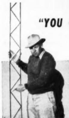
Across the nation the building industry is hauling butt-weld Dur-O-wal. This superior reinforcing member utilizes architecture's oldest reinforcing principle . . . trussed design . . . for both vertical and horizontal reinforcing. Electrically welded of premium quality steel (strength 100,000 p.s.i.), Dur-O-wal handles fast, lays flat, cuts time and costs. Write nearest plant.
