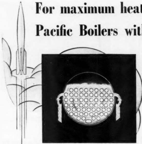
**Jet-action Circulation** is created by Pacific Circulating Connections. Their special design forms hot water and steam from the water leg into a jet stream trained directly on heating tubes. Insulating steam bubbles on the tubes are swept into motion producing a state of turbulence that provides maximum heat transfer.
