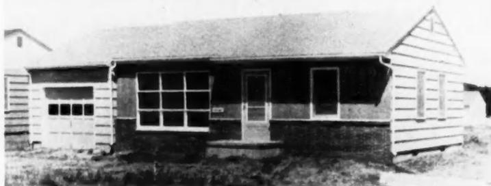
A house of any size can be produced by factory-built modular sections. (Top) The success which Jim Bradfield had with homes like this, built to individual buyers' specifications, led him into speculative building of houses like the one at left. This is the 864 square-foot house Bradfield sells for \$11,500
