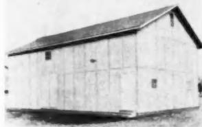
Here's a picture story of the rejuvenation of a 70-year-old barn near Monica, Illinois, which, before remodeling, gave the impression of being hopelessly dilapidated. The framing lumber was still sound, however, so the owner had the building straightened. He then covered the sidewalls with large sheets of asbestos-cement board.
