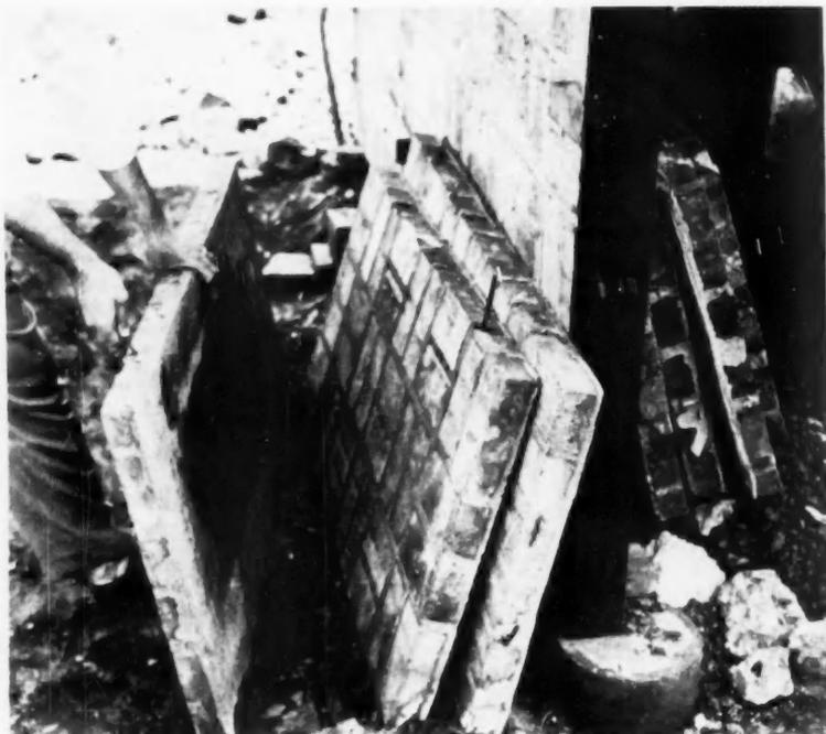
A solid layer of grout covers the "inside" surface of the panel. Rods used primarily for handling purposes can be seen protruding from the horizontal and vertical sides of the panels. Brick is Chicago treated common brick in basketweave pattern.
