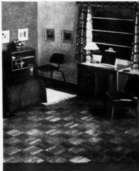
2. Bradley's penetrating primer, superior transparent finish and heavy-bodied wax are mechanically applied and buffed with precision uniformity. Costing less than sanding and finishing on the job, this formula and method bring the natural figure of oak into clear relief and provide a floor of rich luster and matchless decorative beauty.
