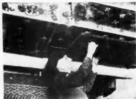
Plaster applied over wire and cork which has been attached to aluminum ducts using MIRACLE ADHESIVE and MIRACLE SPINDLE ANCHORS of John Hancock Mutual Life Insurance Co. Building, Boston, Mass; ARCHITECT: Gram and Ferguson. BUILDER: Turner Construction Co.
