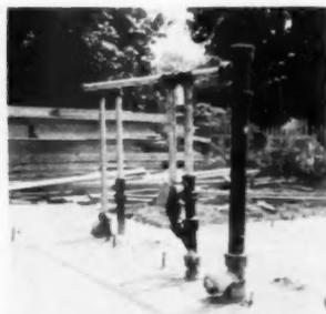
All Lucky Homes have a 4-inch termite-proof, damp-proof concrete floor finished with asphalt tile. This shows a slab under construction, with pretab plumbing tree set in.
