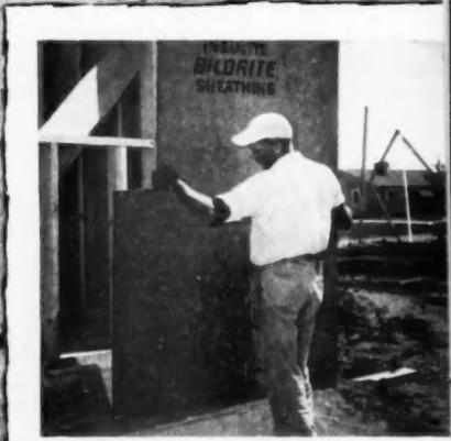
**BILDRITE GOES UP FAST.** One carpenter can sheath 1,000 square feet in six to eight hours and cut labor costs as much as 53 percent! What's more, carpenters like to work with Bildrite because it's clean and easy to handle, easy to cut and easy to apply.
