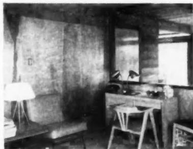
Office window is the only glass area facing the front of the structure. Heavy beam construction can be seen at the top of the side wall. Plywood panels cover all walls
