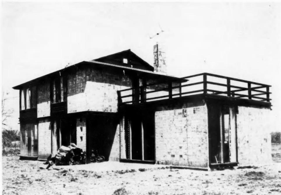
House in Northfield, Illinois, uses precast brick panels both for exterior walls and some of the interior partitions. Cost of the house averaged \$7.72 a square foot
