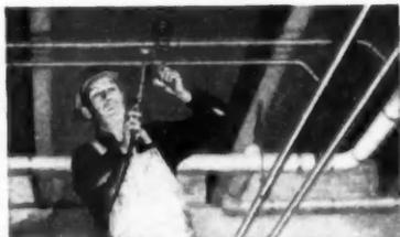
What could be better than long-lasting Chase Copper Water Tube for domestic hot and cold water lines! It is made in hard and soft temper...straight lengths and long coils. Type L hard temper is especially suited for new construction. Soft temper comes in 60 and 100' coils that can be snaked behind walls and under flooring for replacement jobs.
