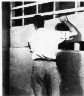
Applying panels horizontally over furring strips above studs. Nails placed in the  $\frac{3}{8}$  inch tongue are covered over by the joining panel, leaving no marring of the surface
