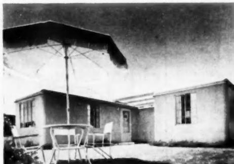
Windows are steel casements, equipped with roto-type hardware and screens. A terrace roof is provided, made of Corrugulux and mounted to a beamed construction. A wide choice of interior and exterior finish color is available
