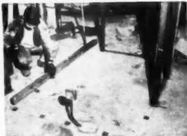
WOOD RUNNERS installed on concrete floors with MIRACLE ADHESIVE and MIRACLE ANCHOR WALLS to support 2" solid partitions. Washington Circle Apartments, Washington, D.C. GENERAL CONTRACTOR: Charles H. Tompkins Company.
