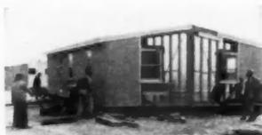
FOR SEVERAL years the Mobilhome Corp. of America, of Bakersfield, Calif., has been producing houses by production line and moving them intact to the owner's lot. To simplify the hauling problem, the company has now developed a split house design which makes it possible to haul a house in two sections measuring only 14 feet each in width.
