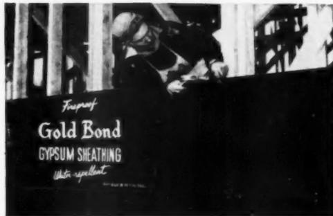
Fireproof Gold Bond Gypsum Sheathing gives extra strength, too. Racking tests prove these big knotless panels give greater structural strength than other commonly used sheathing materials. And the core of gypsum rock is asphalt-treated for increased moisture resistance.
