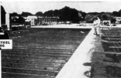
Virginia Square Shopping Center in Arlington County, Va., uses Stran-Steel joists on the first and second floors and roof. Roof construction includes poured Pyragyp deck plus built-up roofing.
