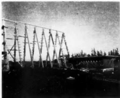
Laminated beams made up of 12 thicknesses of 2x7-inch Douglas fir form the skeleton and are set on 8-foot centers. They are left exposed on interior. 2x6-inch hemlock tongue and groove boards are applied over beams and form the base for metal foil insulation
