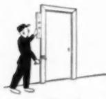
Check plumb, shim, and nail first half to wall.
