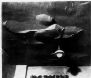
If you want to avoid blister-type failure in plaster finish coats, do not use regularly hydrated (normal) dolomitic lime established that this type of failure resulted from the use of plaster made with regularly hydrated (type N—normal finishing) dolomitic lime.
