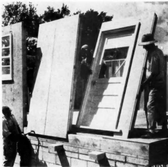
Plywood sheathing on sections is engineered to overlap level of the finished floor, providing a weather-tight seal
