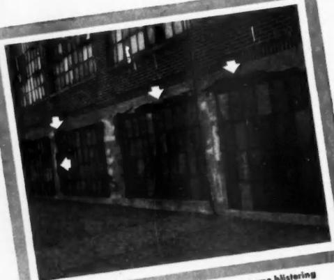
Above photograph shows extreme blistering and spalling of concrete spandrel beams and columns of Pilgrim Badge Building, Boston, Massachusetts which is now entirely protected and further deterioration arrested.
