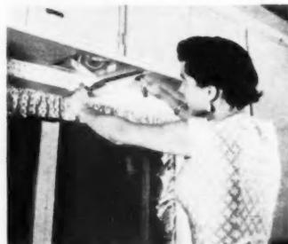
"Snap-up" fronts make Fry-Lites the easiest-to-clean recessed fixtures available. Whether installed in the ceiling or in a soffit cabinet, as shown here, the fronts merely pull down for dusting or relamping.
