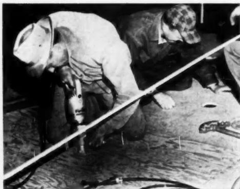
**PORTABLE TOOL EXPERT** from Skilsaw, Inc., uses Skill drill with hacksaw attachment to make pocket cuts for outlet boxes
