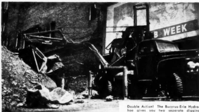
Double Action! The Bucyrus-Erie Hydrohoe gives you two separate digging actions: the first is the conventional dragshovel action of the dipper moving through its digging arc; the second, a separate horizontal stroke, obtained by telescoping the boom. Unit is available with both 18- and 12-in. wide bucket.
