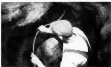
For underground installations there's nothing better than Chase Type K, Copper Water Tube. Type K in soft temper can be easily bent around obstructions...it moves with the earth and settling won't harm it. Long lengths up to 100 feet in coils make few fitting connections necessary. Chase Copper Water Tube resists corrosion, does not clog with rust.
