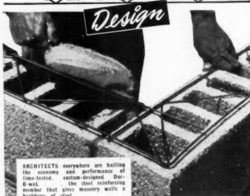
ARCHITECTS everywhere are hailing the economy and performance of time-tested, custom-designed Dur-O-Wal, the steel reinforcing member that gives masonry walls a backbone of steel.
