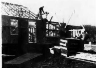
Airplane-type roof trusses are spaced 24-in. on center
