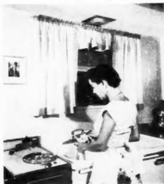
To clean the Bio-Fan electric exhaust ventilator, you simply loosen one part by hand, and the grille and motor assembly are easily removed. Washing with soap and water cuts all grease off the parts.
