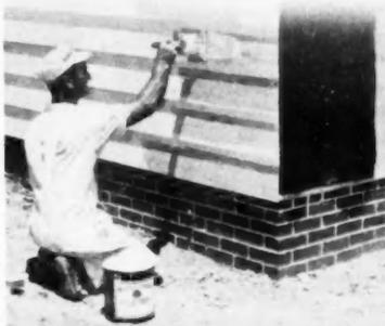
Priming penetrates the resin-free fiber and becomes integral with it.
