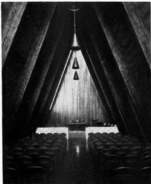
Inside surfaces of the hemlock boards were kerled every inch, thus hiding joints and giving acoustical value. Light comes not only through glass panels over chancel but also from glass panels at rear of nave. The building has radiant heating from copper tubes imbedded in the concrete floor
