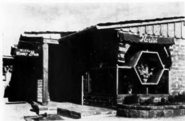
Used brick or rough unpainted lumber comprise the material surrounding the store fronts. Adobe is also used. All buildings rest on concrete slabs. The casual way in which the materials and joints are combined contribute to the charm and atmosphere of the center
