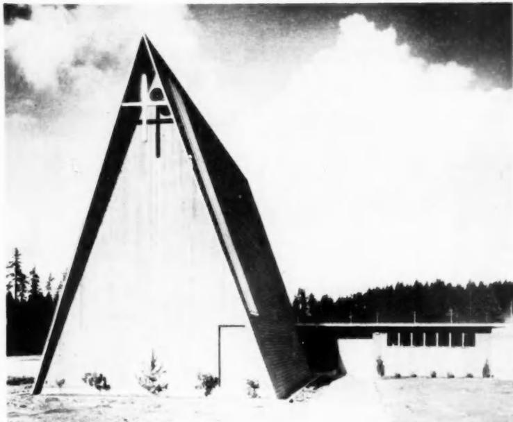
Roof (?) or walls (?) are covered with cedar shingles. Redwood boards applied vertically enclose the other two sides. Offices and Sunday School room are in the low flat-roofed wing
