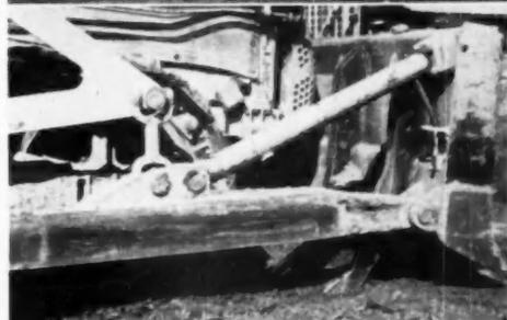
(TOP) EASY MANEUVERABILITY of this two-bladed Fordson tractor fine-grades lawns economically. (Bottom) ripping claws attached to the blade of a Caterpillar dozer is an invention of the Denver concern. The close-up photo shows how reversing the machine rips the earth and makes dozing in hard or frozen ground easier. Normally, claws are in a raised position
