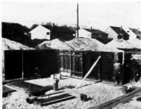
**SETTING UP FORMS** faced with 4x8 sheets of  $\frac{3}{4}$ -inch plywood for the pouring of a 10-inch concrete foundation. During the winter, about four foundations can be poured daily; in warmer seasons, the rate can be doubled or trebled
