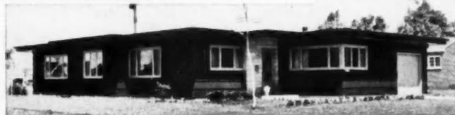
**FOAMGLAS** is used to insulate the roof of this modern home, protecting the occupants from excessive summer heat and winter cold. Since this new home is of the basementless type, **FOAMGLAS** is also used to line the outside of the foundation wall, below grade, and the inside of the recessed hot air ducts under the floor slab. This makes it easy to maintain desired indoor temperatures . . . assures the occupants of a comfortable floor at all seasons.
