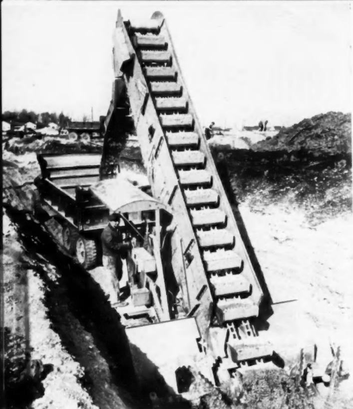
**BIG. POWERFUL TOOLS** such as this expensive loader are found to quickly pay for themselves—if kept busy and cared for properly. Spinning teeth at the bottom break up large chunks of packed or frozen earth into a “fluffy” mass before placing it in the buckets
