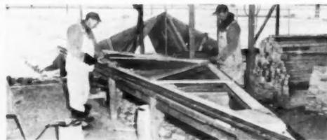
**TRUSS SHED**, adjacent to the cutting shop, receives cut lumber from the shop, makes it up on jigs
