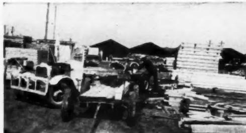
**PRECUT LUMBER** is sized and then loaded at the centrally located yard. Saw is a Comet Clipper radial arm. Lumber is loaded on the trailer in the foreground for delivery to the site. A model A Ford moves the trailer mounted saw
