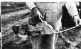
**OPERATOR PULLS TAPE THROUGH MACHINE** to start operation. When enough drag has been established the machine feeds tape as it is drawn along seam
