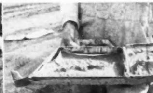
**OPEN MACHINE** shows how tape is run over the joint cement. Pressure against the cement coats the tape
