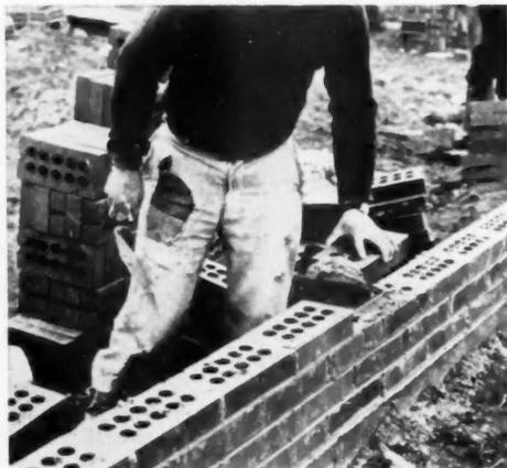
**UNDER NORMAL** conditions, a mason can easily lay 450 SCR brick per day, or 100 square feet of wall. The hole size and arrangement were selected to duplicate the grip and finger spread used by masons in laying 4-inch brick. SCR brick is laid with 1/2-inch mortar joints, turns corners nicely and builds jambs or openings without special additional units
