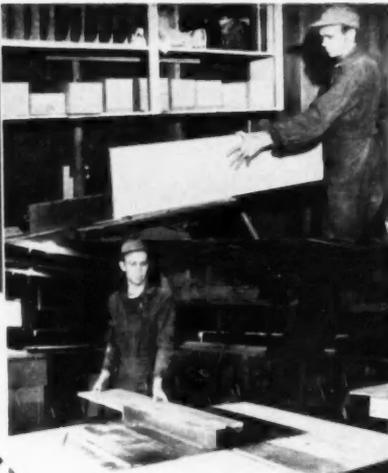
**A 12-INCH TABLE SAW** (Davis and Wells) is used in the mill shop. Note table extensions made by the builder
