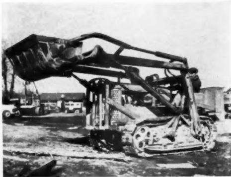
**CLETRAC**, equipped with  $\frac{3}{4}$ -yard bucket, used where the going gets too tough for the “scoopmobiles.” It also has a blade attachment so that it can be used like a bulldozer for light grading work
