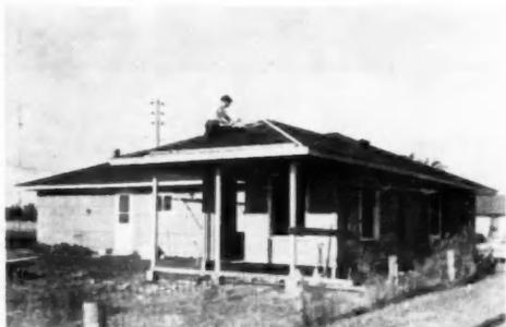
**A 6-FOOT PORCH** and a 2-foot roof overhang give the new addition the length needed to tie in harmoniously with the house. Windows were framed into each of the three walls to give as much natural light as possible. A louver was installed to help insure proper ventilation above the ceiling.
