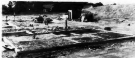
SLAB FOUNDATION encloses pipes for radiant heat. After footing and foundation wall are poured, slag fill is poured in and leveled off. A dampproof asphalt paper is laid over the slag, and the heating pipes are laid on top of the asphalt paper. After testing the pipes, the foundation is covered with reinforcing mesh, the sill is bolted and the concrete is poured. Using a trencher makes possible pouring footing without forms.
