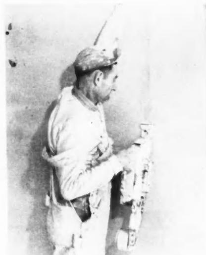
**WALLBOARD TAPER** reduces taping costs approximately 50 per cent in a 1,000 sq. ft. house. Builder claims that a better job is done as the correct amount of joint cement is used. Later joint finishing is easier
