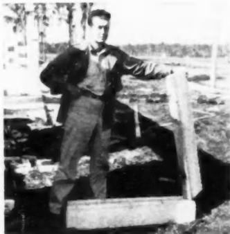
**PRECAST LINTELS:** They are in two pieces in reduce the weight and enable the masons to handle them easily. The void between the lintels is wedged for the aluminum jalousie windows. R. D. Mahoney, construction superintendent, is pictured with the reinforced half lintels
