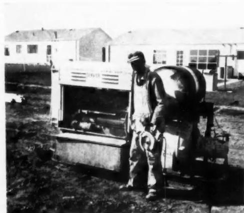
**ENOUGH POWER TO OPERATE** 8 power handsaws is delivered by a 37½ K.W. Buda generator. The rig is mounted on skids to be pulled along the ever moving building line
