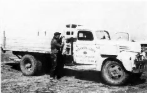
**HEAVY LOADS** are trucked to the site. A Ford stake truck delivers floor joists and subflooring prior to the arrival of the carpenters
