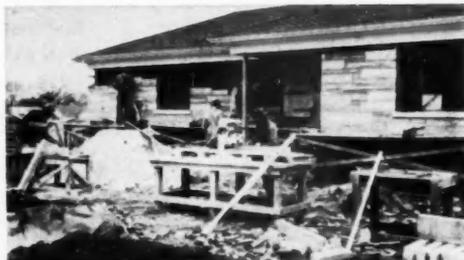
STONE VENEER being cut and laid with aid of radial saw equipped with special cutting wheel
