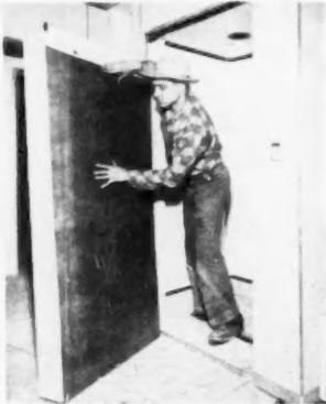
**METAL SHOWER CABINET** is sound-proofed with backing of Masonite tempered hardboard. The usual metallic sounds caused by water spray are said to be deadened by the hardboard. Application is with mastic; here, workman presses board in place to assure a good bond. Shower unit is a product of Fiat Metal Manufacturing Co., which recommends sound deadening in all recessed residential installations
