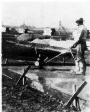
**FLOATING** and finishing floor slab. Whiteman Model J machine weighs 105 pounds, has small trowel diameter for operation on small crowded areas and around obstructions. For small contractor
