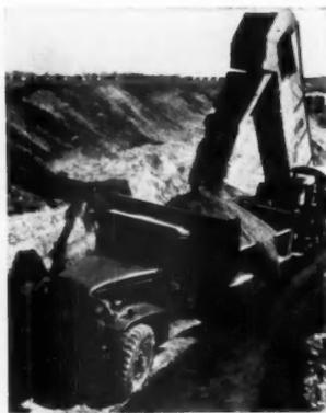
**FIVE-TON DUMP TRUCKS** team up with the loader to move sand and dirt. This sand pit was discovered on the property after the project got underway
