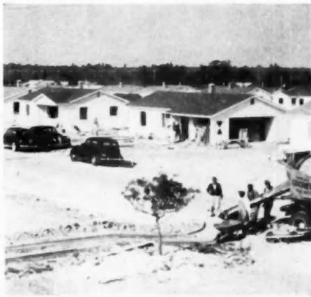
**TRANSIT MIX CONCRETE** is loaded into wheelbarrows for construction of the ribbon driveway. The overall view of the project shows roof lines and many house variations
