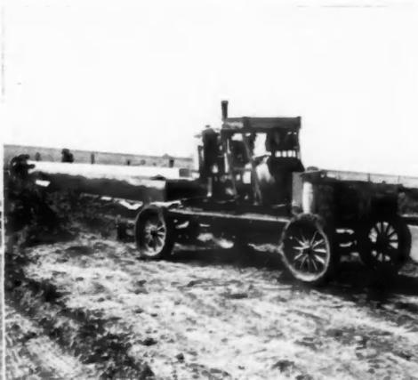
**PORTABLE GENERATOR** is assigned to the crew that lays floor joist and subfloors. The trailer mounted generator is a 7½ K.W. Hobart
