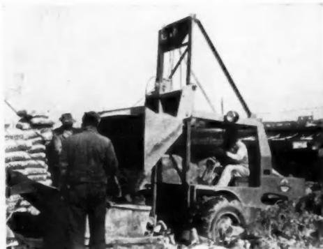
**WAGNERMOBILE SCOOP**, dubbed "scoopmobile" by the builders, pouring aggregate into one of the mixers. Three of these are on the job and each is estimated to save the labor of three men and do the work twice as fast
