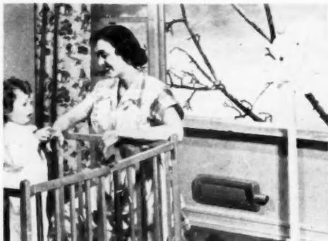
**AUTOMATIC AIR WALL register installation.** Warm air is delivered upward along walls in fan-like pattern
