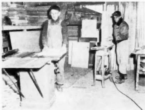
**RABBETING AND DADOING** with a Delta table saw, and a joiner for straightening, are indispensable tools for Precision's cabinet making. Boards for cabinets are bought precut
