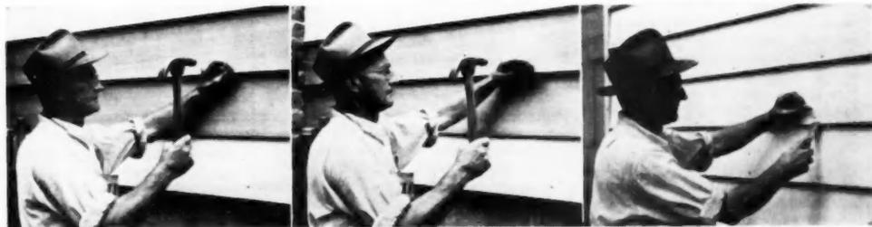
**SIDING SHOULD BE NAILED** both top and bottom to prevent curling. Exposed nails should be countersunk and puttied for best appearance and service, after the primer goes on. When the putty has dried, the siding is ready for the finish coating.
