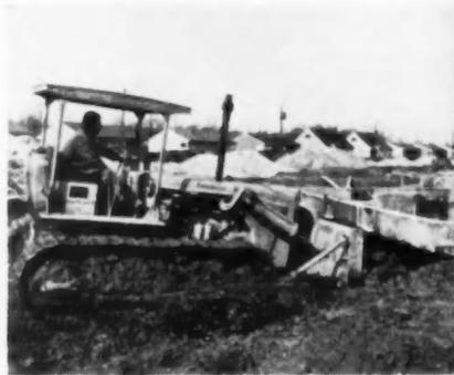
**CATERPILLAR D-6** diesel-powered bulldozer, at work on backfill. This machine is also used for preliminary leveling of the home sites, digging and grading
