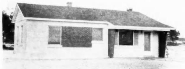
**MASONRY:** The concrete block exteriors are laid with horizontal joints raked and the vertical joints struck smooth. Variations of the exteriors are accomplished by the use of slump and other brick
