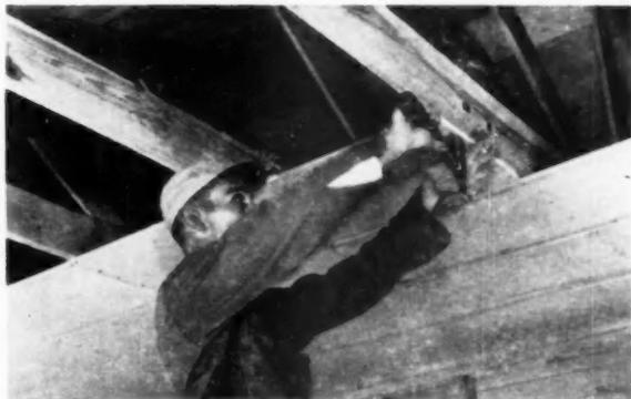
**PLASTER:** Special 2x4 foot gypsum lath is nailed to underside of truss as plaster base. An accelerator was mixed with the plaster to speed drying before the lath became saturated and sagged. This method permitted 24-inch truss spacing
