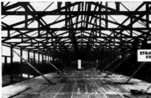
Non-combustible Stran-Steel framing members were used for exterior walls, interior partitions, roof trusses, and floor joists in New York State Conservation Department building at Sherburne, N. Y.
