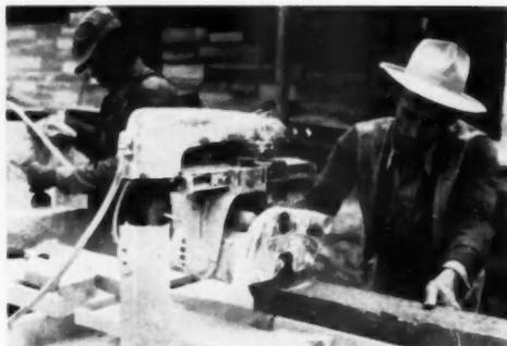
ABRASIVE stone wheel makes clean, fast cut
