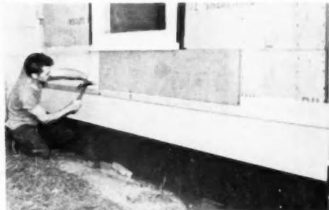
**COMPLETE INSULATION** is an essential feature of a job like this. Mineral wool batts were used. Insulating sheathing was used as well as an insulation board shingle-backer, instead of low grade shingles as under-courting.
