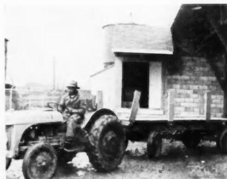
**2** ONE PER CENT—This Memphis builder figures about one per cent saving by using trailers to haul materials instead of trucking and dumping on the ground. In round numbers the savings amount to \$90 per house. The advantages as stated by the builder are not easily determined
