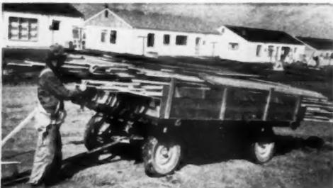
**LOADED TRAILER** of framing lumber precut and pre-marked is ready for the carpenters. 1x2's in the load are used for shingle nailing under the insulated sheathing. Window and door units arrive in pre-fabricated sections
