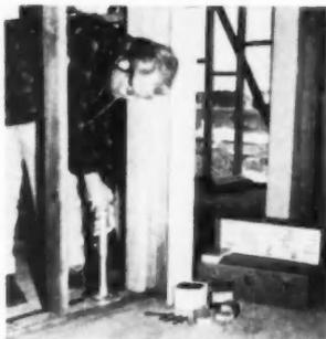
**FASTENING** partition plate to concrete floor with Drive-It. Avoids costly guessing about where bolt should go, placing in wet concrete, and finishing around by hand. Drive-It uses 3/8-inch case-hardened bolts, sinks two inches in concrete, costs 27 cents a shot, fires about 100 in an hour
