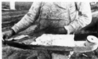
**TAPE ROLLS OFF BACK SPINDLE** through the box which holds joint cement. Machine has built-in knife to press the tape against the seam
