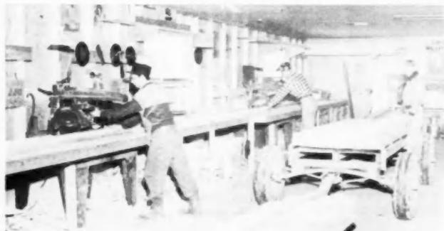
**IN CUTTING ROOM,** two DeWalt table saws, of 220 volts, carry the work load. Lumber for each house is cut, loaded neatly on a trailer and bound with steel tape by means of ratchet and steel binder. This package is then delivered to the individual site
