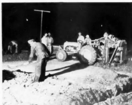
**3** 75 PER CENT—Power trenching in which footings and trenches for gas, sewer, and water lines are dug save 75 per cent in labor cost when compared with using hand labor, was a statement of George Young, vice president in charge of construction
