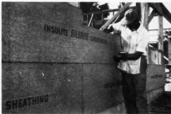
**BILDRITE GOES UP FAST.** One carpenter can sheath 1,000 square feet in six to eight hours and cut labor costs at least 25 percent! What's more, carpenters like to work with Bldrite because it's so clean and easy to handle, easy to cut and easy to apply.
