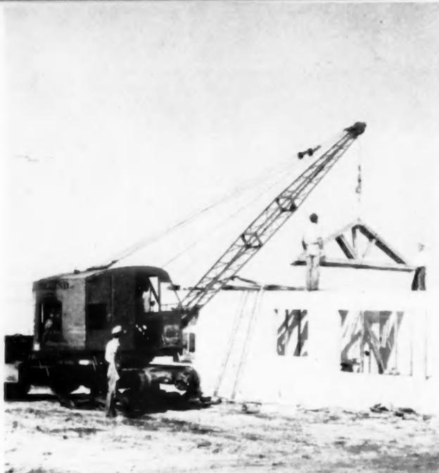
**SCHIELD-BANTAM CRANE** lifts three roof trusses to the carpentry crew at one time. The machine is mounted on a U.S. Army surplus half-track. The crane can be fitted with a  $\frac{3}{8}$ -cubic yard drag line
