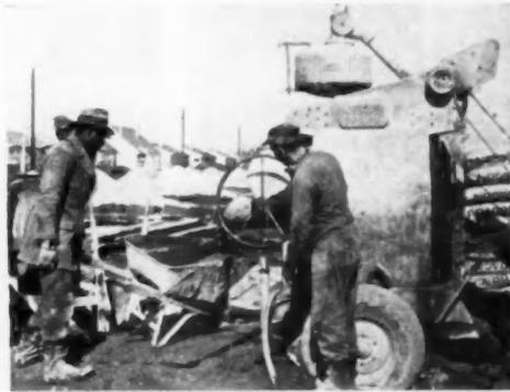
**CONCRETE MIXER**, which keeps a crew of three men busy pouring foundations. Two of these machines are used at each site. A third is set up in advance for the next foundation. A fourth mixer services a flatwork crew
