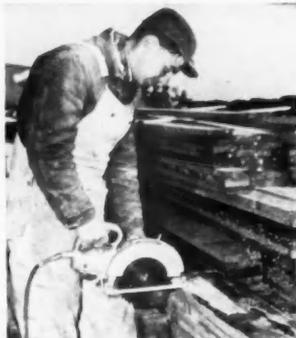
**ELECTRIC SAW** poised to do a quick job of cutting 2x8 joists. A generator supplies the power whenever an outside source of electricity is unavailable
