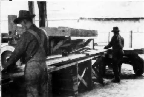
**1** 30-60 PER CENT—Using a centrally located precut operation Johnson saves thirty per cent over a site power tool operation and sixty per cent over a hand tool operation. "In other words," stated Johnson, "we can cut one of our codes (code H—openings, studs, corners and tees) for \$1.75 labor cost in the shop against \$8.75 if it were done with hand tools on the job."
