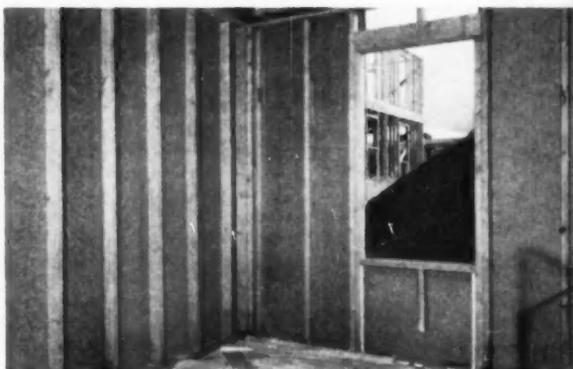
**ELIMINATES CORNER-BRACING.** 4-foot Bildrite without corner-bracing has more than twice the bracing strength of horizontal wood sheathing. Bildrite's tremendous bracing strength is actually greater than that of diagonal wood sheathing.
