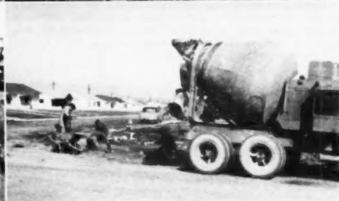
(TOP) THE FRONT-END LOADER is pulling a sheepfoot roller compacting street fill. Front-end loader is a L.I. Case tractor. (Bottom) crawlspace construction requirements are 30 inches. Builder uses International TD-9 to push out for crawl space and foundations. Later machine will be used to backfill
