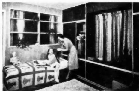
**A PATTERNED GLASS PARTITION** was framed into the wall which divides the new room from the old. An opening was left at the top to allow cross ventilation. Three-quarter-inch factory finished insulating was used on the walls. Tempered hardboard in its natural brown color was used as facing on closets and drawers of storage wall.
