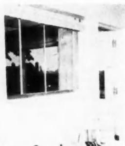
MANUALLY CONTROLLED sliding window, partially opened, showing screen attached to right edge of window
