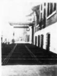
**AB12185 — COLORUNDUM FLOORS**—A. C. Horn Co., Inc., Dept. AB, 10th St. and 44th Ave., Long Island City 1, N. Y. Colored concrete floors and sidewalks with a wear-resistant topping are achieved by this product. Colorundum is a dry powder which is trowelled into the fresh cement finish. Not a paint or coating.
