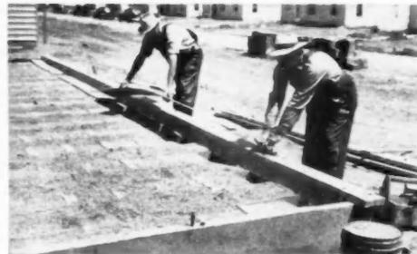
WITH TILE and fill in place, central duct is covered. Note concrete bottom, sloping up and out, is poured after side forms are removed. Steel reinforcing rods over trench support sheets of impregnated fibre board insulation
