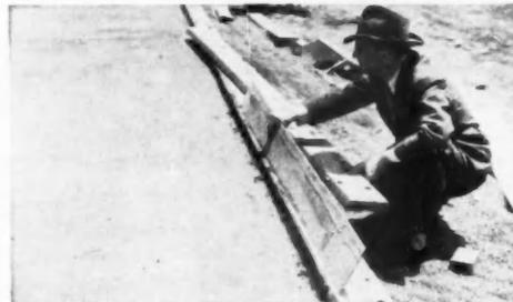
CLOSER VIEW of two-part form used to protect warm air discharge trench. In completed system a slotted baseboard runs full length of trench at an angle between the wall and floor. Wood and sheet metal forms are removed after slab has set
