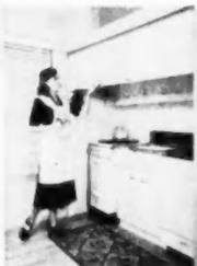
**AB12193 — ROLL-UP KITCHENETTE DOOR** — Orchard Bros., Inc., Dept. AB, 63 Meadow Rd., Rutherford, N. J. An aluminum door which is a space-saver in kitchenette and closet closure. Made of interlocking slots, it operates from a counter balance spring roller at the top. Comes ready for installation on plastered or unplastered walls.
