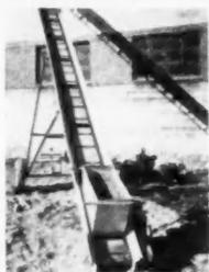
**AB12169 — ELEVATOR-MORTAR BOX** — Sam Mulkey Co., Dept. AB, 1621 Locust, Kansas City, Mo. The new Mulkey mortar box, pictured here on a 40-foot Mulkey elevator, will lift 10 wheelbarrows of gravel or concrete to a maximum height of 28 feet in just 15 minutes. For return, box is simply inverted and slides down the flanges.
