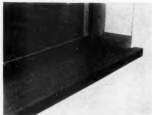
A MAHOGANY patterned Formica sill installed in a casement window is shown after the trim is applied
