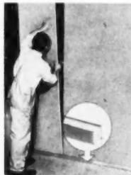
**AB1282 — GYPSUM LATH PARTITION**—National Gypsum Co., Dept. AB, Buffalo 2, N. Y. Cold Bond partition can be used without studs in any type of building where non-load-bearing partitions not exceeding 12 feet in height are specified. Plastered on both sides to two-inch thickness. Has metal attachments. Booths 205, 206, Stevens.
