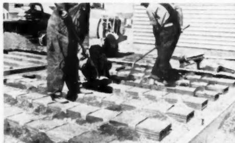
JOINTS ARE SEALED against wet concrete with strips of vapor barrier material. Strips are obtained by cutting roll of material in desired width. A spadeful of gravel on each end holds material while space between courses is filled with gravel
