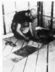
**AB12455 — ALUMINUM FOIL INSULATION** — Reflectal Corp., Dept. AB, New York City. Expressly for insulating spaces 1/4-inch deep. ALFOL Type IA has a pure aluminum foil surface which expands to a depth of 3/8-inch. This enables Type IA to pack the tight 1/4-inch space with two reflective air spaces. Comes in 250 square foot rolls.
