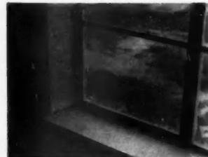
**INSTALLED SILL** is now ready for the finished coat of plaster. All voids will be pointed up by the plasterer
