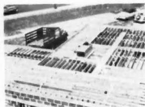
ROOF CONSTRUCTION is 2 x 10 inch joists 12-inches on center. Heating unit is shown installed on roof
