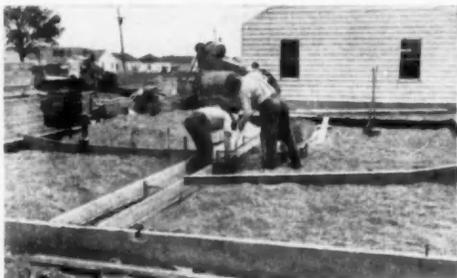
THE LAYOUT of heating system begins with the formation of central trunk duct. Concrete and curb is trowelled in against form for walls of duct. Bottom of duct slopes up and out from center toward edges. Fill is pea gravel
