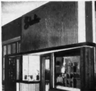
**KAISER ALUMINUM ROOFING** makes an attractive, modern store facade. Used as a remodeling material, it gives older buildings new sparkle, fresh appearance. Lower in cost than most architectural specialties, it needs minimum of maintenance because it's *solid* aluminum, not clad or veneered.
