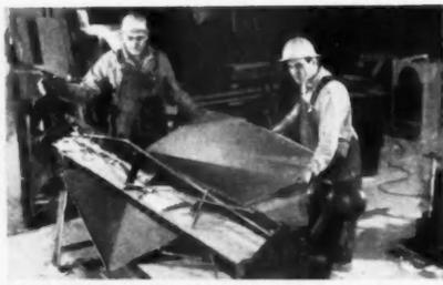
**FABRICATING KAISER ALUMINUM** into ductwork is so simple the contractors set up shop right on the job—and eliminated several steps in handling, trucking and storing assembled sections. Kaiser Aluminum is less wearing on shop equipment, can be fastened with rivets, by welding or with sheet metal screws.
