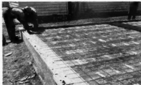
WITH FORMS in place, reinforcing mesh is placed over entire slab. Approximately 300 to 350 tile are required for the average two or three bedroom house. The system can be installed in about 60 man hours including furnace and slotted baseboards
