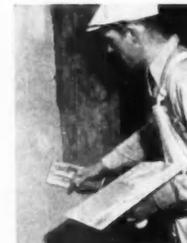
**AB12129 — BONDING PLASTER** — Nu-Wall Mfg. Company, Dept. AB, 923 N. 19th St., Milwaukee 3, Wis. Plasterer is shown applying a thin coat (approx. 1/8-inch thick) of Nu-Wall bonding plaster, making the problem surface suitable for any type of applied finish. Approximately 20 yards to a 25-pound sack, sold company.
