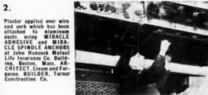
2. Plaster applied over wire and cork which has been attached to aluminum ducts using MIRACLE ADHESIVE and MIRACLE SPINDLE ANCHORS at John Hancock Mutual Life Insurance Co. Building, Boston, Mass. ARCHITECT: Cream and Ferguson. BUILDER: Turner Construction Co.
