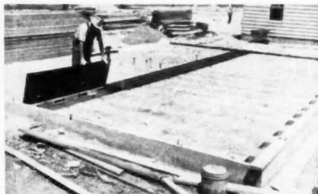
TWO-PIECE FORM of wood and steel plate is bolted to the foundation wall anchor studs. The steel strip angles downward and when mat is poured the slab edge becomes an angular baffle to throw the warm air upward as it comes out of the duct
