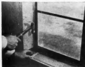
**THREE OR FOUR SHIMS** are nailed into place. These bring the sill to the proper height
