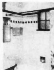
**AB1252 — PLASTIC WALL TILE** — Tilemaster, A I Plastic Molders Inc., Dept. AB, 1415-21 Diversey Parkway, Chicago 14, Ill. A bullnose cap and an out corner for the same has made it possible for a complete tile installation without the use of metal or rubber pieces. Six new colors bring the total to 32. Booth 19-20, Congress
