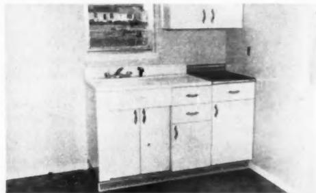
IN PORTION OF KITCHEN where cabinets are placed, ducts do not extend to wall; instead they discharge through grille in front of sink and cupboards.
