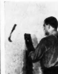
**AB12465 — STABILIZING INGREDIENT**—Flexrock Co., Dept. AB, Filbert and Culbert, W. of 36th St., Philadelphia 4, Pa. Flexite is to be mixed with cement or cement and sand to produce an easily handled mortar to speed up action in sealing off leaks in concrete walls, even against hydrostatic pressure. Said to seal off severe leaks.
