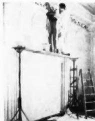
**AB12165 — SCAFFOLD JACKS** — Wilson-Albrecht Co., Inc., Dept. AB, 3565 Wooddale Ave., Minneapolis 16, Minn. All-steel, all-welded Waco Scaffold Jacks give a working platform in quick time, are lightweight, portable and free-standing. The jack is available in four sizes, adjustable every two inches from 1-foot 6-inches to 11 feet.
