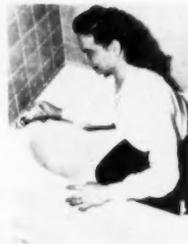
**AB12191 — CAULKING FOR TUBS**—Miracle Adhesives Corp., Dept. AB, 214 E. 53rd St., New York 22, N. Y. This new product, "Tub-Caulk," dries in one hour leaving a tough water-proof bond. It is a plastic and will not dry out. Effective for tubs, shower stalls, sinks, and for filling cracks between window frames and tile or plaster.
