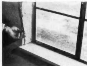
**SILL** is inserted into the opening and screwed into place. A 60 degree hole is drilled through the sill into the header and a 2½ inch screw fastens the unit
