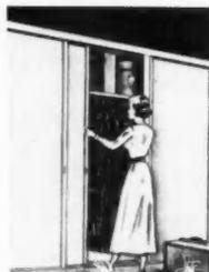
**AB12205 — SLIDING DOORS**—Farley & Lubliner Mfg. Co., Dept. AB, Dubuque, Iowa. A Broadway unit consists of two doors with surrounding frame. Doors are pre-fit, primed, ready for installation. Nylon glide rollers are used, which never need lubrication. The doors are basically wood with 3/4 inch Masonite faces.
