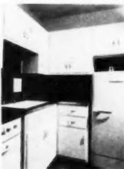
**AB1216—PLASTIC FACED PLYWOOD**—GPX, Georgia-Pacific Plywood Co., Dept. AB, 1257 Southern Finance Bldg., Augusta, Ga. Paint grade plastic faced plywood was used in these cabinets. Labor savings of 50 per cent and material savings of 5 cents a foot are claimed by the manufacturer. Less paint is required. Booth 246, Stevens.
