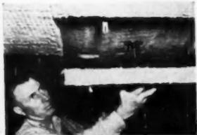
3. FIBERGLAS insulation Type PF-613, 2" thick — bonded to concrete ceiling using MIRACLE PRONGED ANCHORS at Radio City Studio 60, New York, N. Y. CONTRACTOR: William J. Smith, Inc., New York, N. Y.
