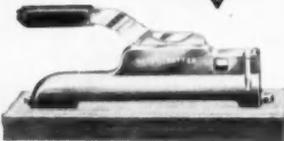
The SCOUT is a small utility cutter for asbestos siding and shingles, with front end nose punch. The cutting blade is made from a high grade steel, heat-treated, has sharp serrated teeth machined by a milling cutter. Overall length 16", height 6", width 2 1/4". Approx. wt. 3#. The base of the Scout Cutter is high-grade aluminum casting, having the proper amount of weight necessary to perform the best operation by the applicator.
