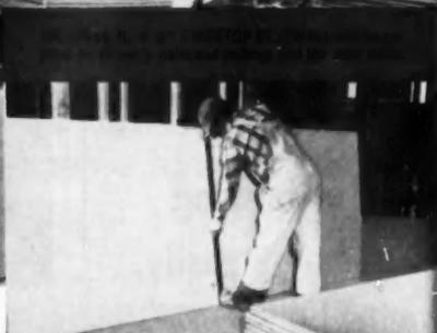
F.H.A. wall and ceiling specifications are being met successfully for the first time with a single layer of  $\frac{1}{2}$ " wallboard.
