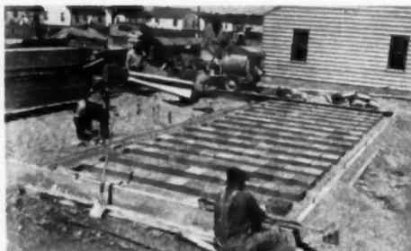
LATERAL DUCTS are laid from main duct to discharge trench along outside wall. Weight of tile-setter standing on block when placed in position serves to bed tile in vermiculite. Broken tiles between laterals prevent fill from spilling into main trunk
