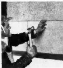
**Shingle-Backer goes up fast, stays put,** provides a firm, even under-course for exterior shingles. Saves application time and eliminates waste. Takes just four nails to apply full 48" panel. Made of genuine, weatherproofed 5/16-inch GRAVILITE insulation board. Shingles and Shingle-Backer have approximately twice the insulation value of conventional shingle application.
