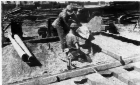
A VAPOR BARRIER is placed over the leveled off fill and is covered with a layer of loose vermiculite. Lateral ducts are laid on this material at right angles to the main trunk duct. Laterals are standard 4x12x12 inch wall tile
