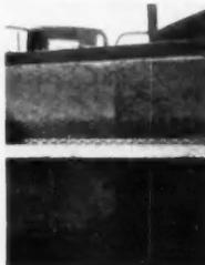
**AB12441 — TERMITE SHIELD** — B and R. Company, Dept. AB, P. O. Box 93, Plano, Texas. A new termite shield that is permanent has an expandable metal edge that is bonded to the beam. The bonding is done with cement mortar. Corner miterers are prefabricated. The shield joins together with metal clips, no soldering is needed.
