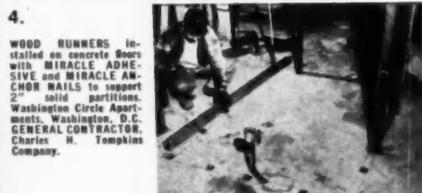
4. WOOD RUNNERS installed on concrete floors with MIRACLE ADHESIVE and MIRACLE ANCHOR NAILS to support 2" solid partitions. Washington Circle Apartments, Washington, D. C. GENERAL CONTRACTOR: Charles H. Tompkins Company.
