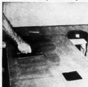
**ADHESIVE** is applied to hardboard panel with a saw tooth trowel
