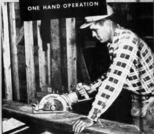
**One-hand operation.** "One hand on the saw, one hand on the work, and your eye on the blade makes accurate sawing easy with a SKIL Saw," says William Skaggs. That plan of action is demonstrated as he cuts a stair stringer with SKIL Saw Model 77.
