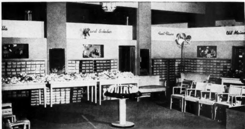
COMBINATION shoe storage racks, false wall, and shadow boxes in this shoe department of a large store were constructed of hardboards on a framework of lumber. Construction details of these various units are covered in the drawing below
