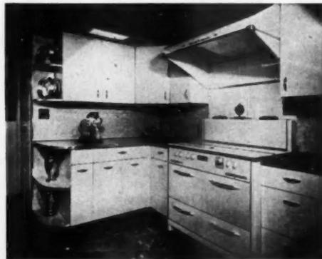
VENTILATING hood was installed over the range. New cabinets at left and right provide added convenience. In the old view note that no cabinets or work tops were placed adjacent to the range
