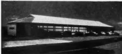
THIS FISH NET SHED, covered with Kaiser Aluminum Roofing, is designed for a seaside location in a hot climate. The roof is highly resistant to the corrosive action of salt spray from the nearby ocean because Kaiser Aluminum Roofing is *solid* aluminum—not clad or veneered. And Kaiser Aluminum Roofing reflects up to 60 per cent of the sun's rays, which means a reasonably uniform, cool temperature is maintained under the shed.
