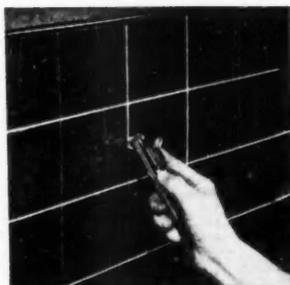
**SCOREMARKS** of tileboard are finished in a second color with a striping tool
