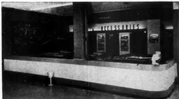
**HARDBOARD** is adaptable to modernization where curves are elements of design
