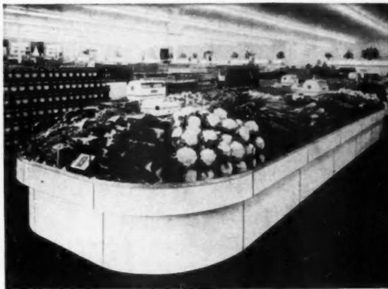
**PRODUCE** display paneled with glossy white factory-finished hardboard. Metal moldings are used at the joints. Factory-finished hardboards are easy to maintain, not easily marred
