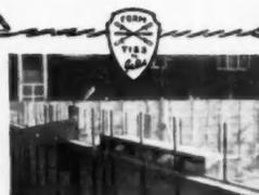
Forms come off in half the time or less. Walls are clean, even, no overlap. Use Gates Concrete Form Ties for walls 6" to 60", any height. Ties also available for in-the-wall break off.
