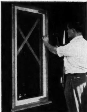
**2** **ATTACH OUTSIDE FIN** — Next, attach metal fins at jambs. The grooved edge of the fin fits over the edge of the steel frame. The flat surface of the fin is nailed to the sheathing. Exterior trim can now be applied.
