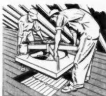
A Hunter Package Fan is the most practical and least expensive method of keeping a home comfortable on hot summer nights. This compact unit is easily installed in any new or old home. Furnished complete with fan, motor, suction box and ceiling shutter—with a choice of four sizes, to fit any home.
