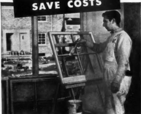
All R·O·W sash may be removed and painted at one time and in one location. Sash may be covered and stored away from frames to reduce breakage costs. Removable sash reduce reglazing and other maintenance expenses.
