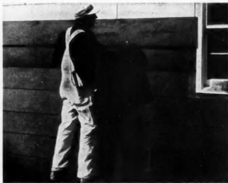
Leaving a two-inch overlap, a carpenter prepares to nail a panel of Masonite 1/4" Tempered Presdwood over the insulation sheathing on the William A. Schraegle home at Parma, O.
