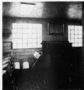
**ELECTRICAL** radiant glass heating panels are being used extensively to heat dairy barns and milk houses on farms where electricity in rural areas has been made available. The cost of the heating equipment was \$478.10. The cost of the complete wiring job including house wiring and fixtures amounted to \$236.50 for labor and \$443.60 for materials.
