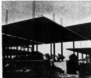
**YOUTZ-SLICK** Lift Slab building method was successfully used in first commercial test in erection of Trinity University administration building shown during construction
