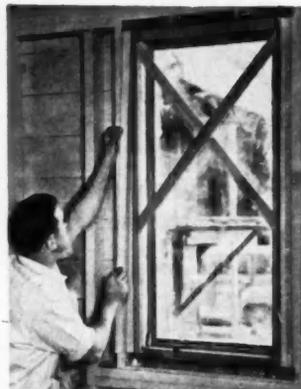
**3** **ATTACH INSIDE FIN** — To complete the installation, apply the inside metal fins at head, sill and jambs. Fins fit under the lip of the steel frame and are nailed to the studding. This insures a tight weatherseal all the way around the window.
