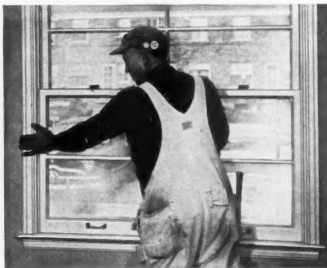
Free Paint Lock in this Amazing Way: Press exposed metal sash channels (at left) and sash against spring pressure, paint lock is broken. A whole house takes just a few seconds.
