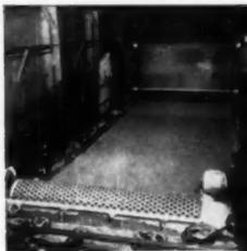
A wet blend of wood fibers passes through the board "former" in Simpson's Insulating Board Products factory.
