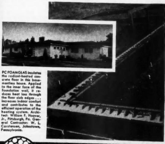
PC FOAMGLAS insulates the radiant-heated concrete floor in this basement house. Applied to the inner face of the foundation wall, it reduces heat loss through the floor slab edges . . . increases indoor comfort and contributes to the efficient operation of the heating system. Architect: William F. Hoover, Jr., Pittsburgh, Pa. General Contractor: W. L. Carlensen, Johnstown, Pennsylvania.
