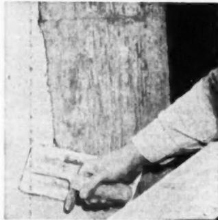
NU-WALL being applied directly to poured concrete column. Approximately 250 to 300 yards of NU-WALL was applied per man each day. 1/8" plaster finish is all that was used to complete job.
