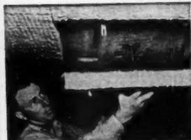
3. FIBERGLAS Insulation, Type PF-613, 2" thick — bonded to concrete ceiling using MIRACLE PRONGED ANCHORS at Radio City Studio 68, New York, N. Y. CONTRACTOR, William J. Sealy, Inc., New York, N. Y.
