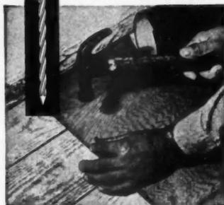
To make your linoleum underlays hold tightly and lay flat permanently, secure them with Hassall linoleum underlay drive screws. They are spiral-threaded and cement-coated for maximum holding power. Heads are flat countersunk type. Size: 1 1/4" x #3 ga. State quantity when writing for prices to:
